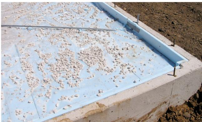
**Photograph 2: Perimeter Slab Edge Insulation and Perimeter Slab Insulation**—Two inches of rigid insulation is about the maximum practical thickness possible. Notice that the sheet polyethylene “vapor barrier” is located on the top of the rigid insulation between the rigid insulation and the bottom surface of the concrete – in direct contact with the concrete. Do not, and I repeat, do not locate the polyethylene under the insulation as it will keep the insulation wet.
