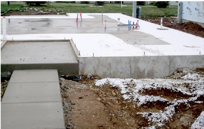
**Photograph 5: Poor Persons Infrared**—Look at the snow melt pattern outlining the under slab insulation.
