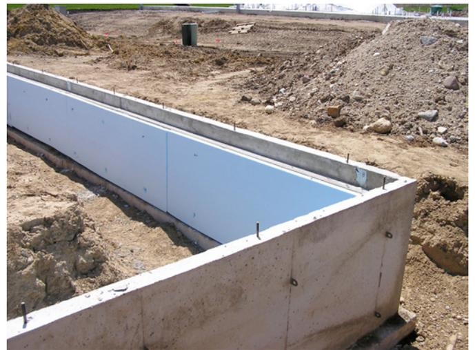
**Photograph 1: Insulated Stem Wall**—Rigid insulation full height on the inside of the stem wall. Note the deep “seat” cast into the inside of the top of the stem wall. This “seat” will receive the perimeter edge insulation and the perimeter slab insulation as well as the concrete.
