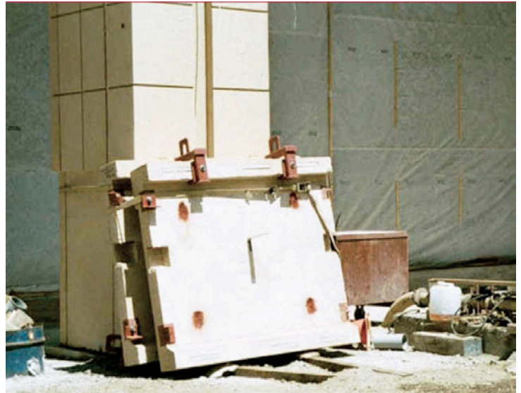
Photograph 2: Back Side of Panel —First condensing surface if interior air gets access to surface.
