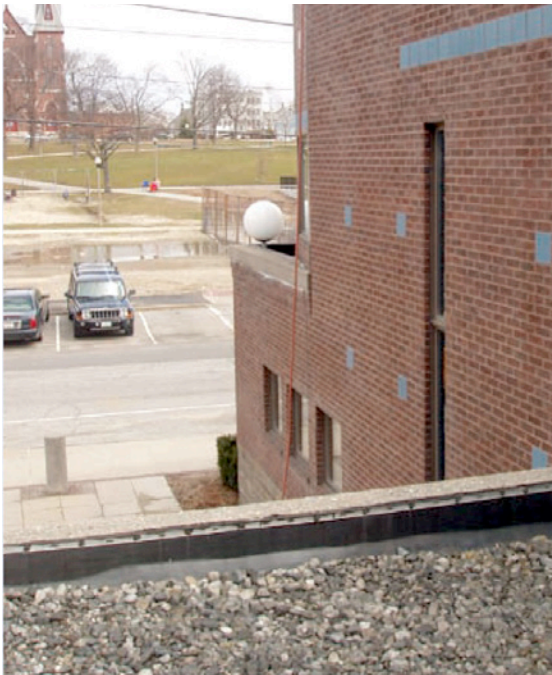
Photograph 3 (left): Membrane Shrinkage —Notice the roofing membrane being pulled away from the cant strip. Photograph 4 (right): Tear in Membrane —Membrane shrinkage results in the membrane pulling apart.
