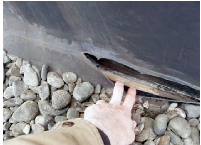
Photograph 3 (left): Membrane Shrinkage —Notice the roofing membrane being pulled away from the cant strip. Photograph 4 (right): Tear in Membrane —Membrane shrinkage results in the membrane pulling apart.
