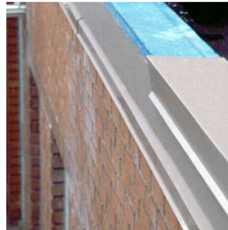
Photograph 1: Excellent Water Management —Notice the membrane under the coping. Notice the slope to the interior. And, notice the drip edges.
