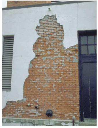
**Photograph 3: Scupper**—This is a no brainer. Don't dump the roof water onto the wall. This is not an insulation problem. This is just dumb.
