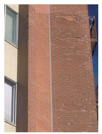
**Photograph 4: Early '80s Ontario Apartment**—The brick is clearly experiencing freeze/thaw damage. It should not be doing this because the brick is not being exposed to what I would define as an extreme exposure. The brick turned out to be pretty bad when tested with an  $S_{crit}$  of less than 0.5, which is unusual for a 30-year-old brick. Most of us felt that by the '80s we had figured out how to make good brick. Apparently, that's not the case here.
