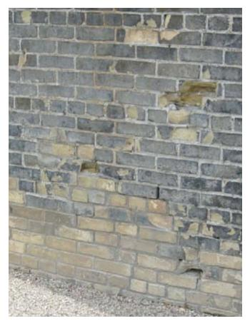
**Photograph 2: "Classic" Freeze/Thaw Damage**—Low to the ground, not very exposed to rainwater and in really bad shape. It turns out that this is a "bad" brick with a low S<sub>crit</sub>.
