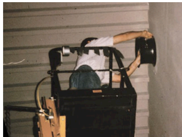
Photograph 11: Duct Blaster® pressurization of parapet assembly.
