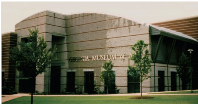
Photograph 8: Fire hose wetted reservoir cladding.
