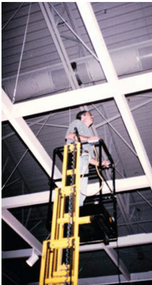
Photograph 9: Installing pressure taps.
