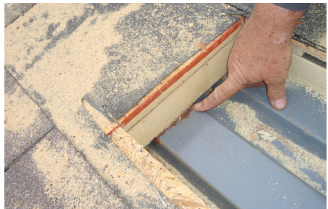
Photograph 10: Rust Stains —Note the evidence of moisture at the panel joints on the top surface of the fluted metal roof deck.
