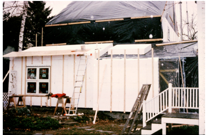
Photograph 1: World’s Largest Canadian Beer Cooler Located in Westford, MA —Barn retrofit with 8 inches of rigid foam on the exterior walls and 10 inches of rigid foam in one layer on the roof. The key thing to note is that the rigid foam on the roof is in one layer. Because it is in one layer it leads to convection.
