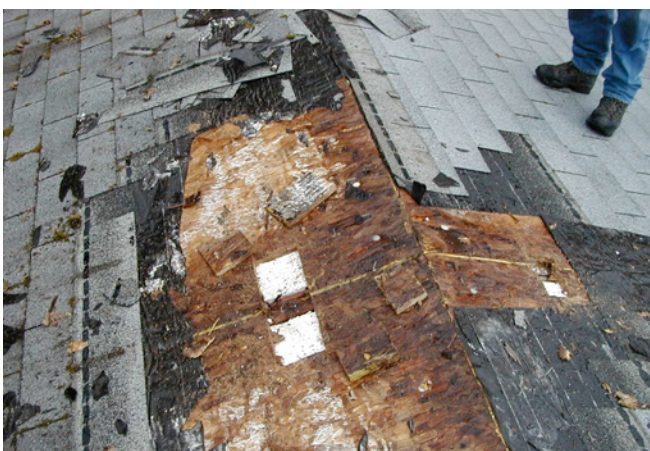
Photograph 5: Moisture Damage —Rot at panel joints and ridge.
