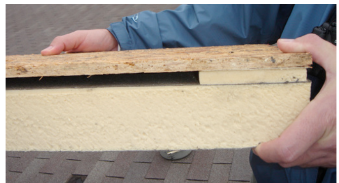
Photograph 8: Vented Foam Panel —The upper panel surface is OSB that acts as a nail base for shingle and other roofing systems.
