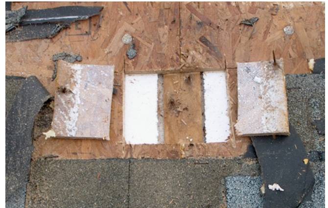
Photograph 6: Micro Air Ducts —Note the air gap on each side of the SIP joint spline creating parallel micro air ducts. The upper pair of air ducts are typically connected to the lower pair of air ducts at panel joints.
