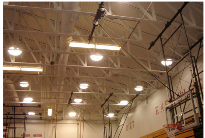
Photograph 7: Sloping Fluted Metal Roof Deck —Condensed water from exfiltrating interior moisture laden air in the winter and infiltrating exterior moisture laden air in the summer leads to moisture damage.
