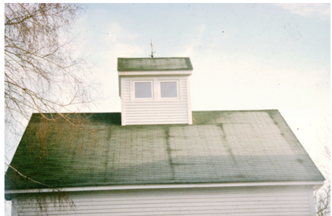
Photograph 2: Professional Embarrassment —Convective cells evident in frost melt pattern on shingles.
