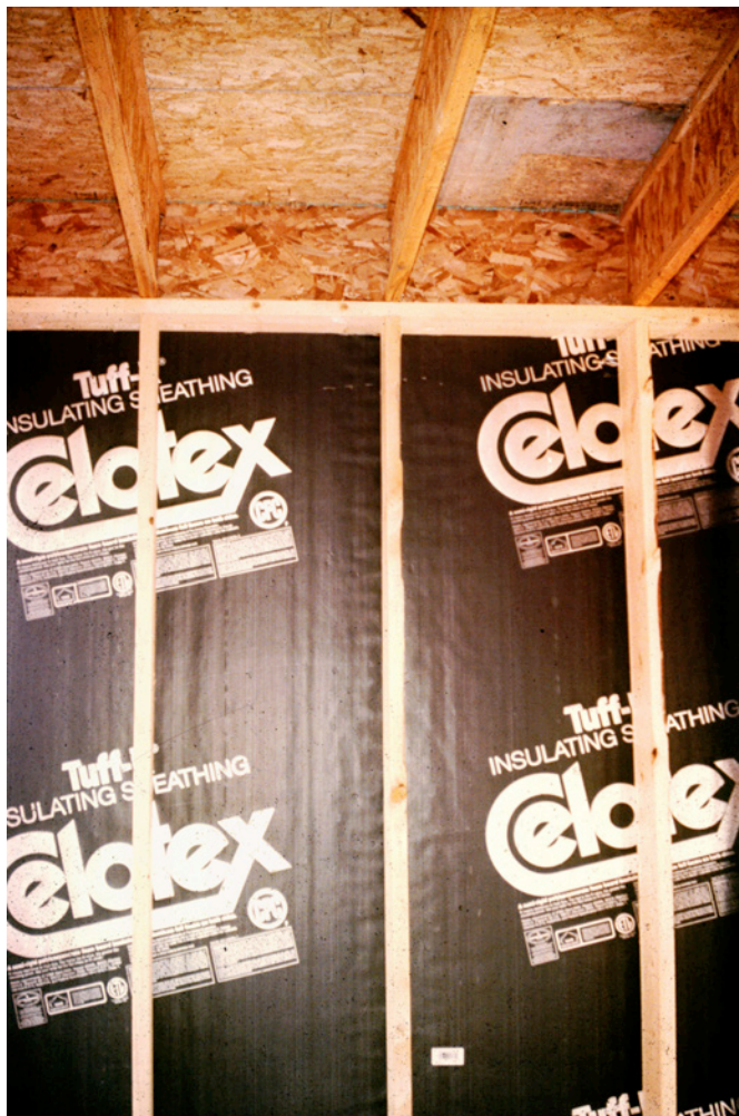
Photograph 1: Stack Framing - Everything lines up so that double top plates are not necessary.
