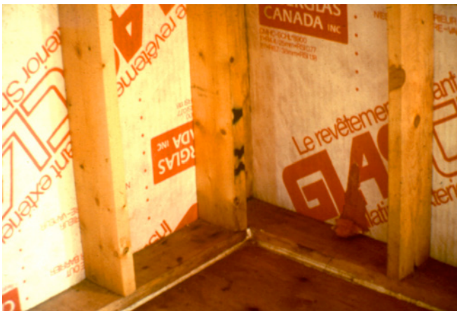
Photograph 3: Corner Framing - My first advanced frame building in 1982 using a two-stud corner.
