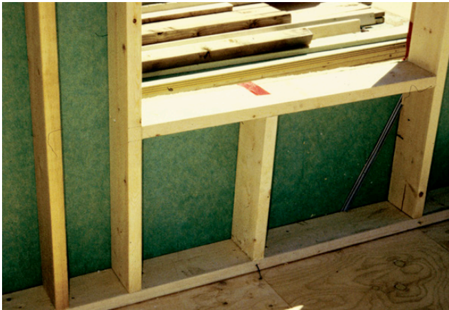
Photograph 2: Window Opening - Non-load bearing wall window openings are clean without jack studs and cripples.
