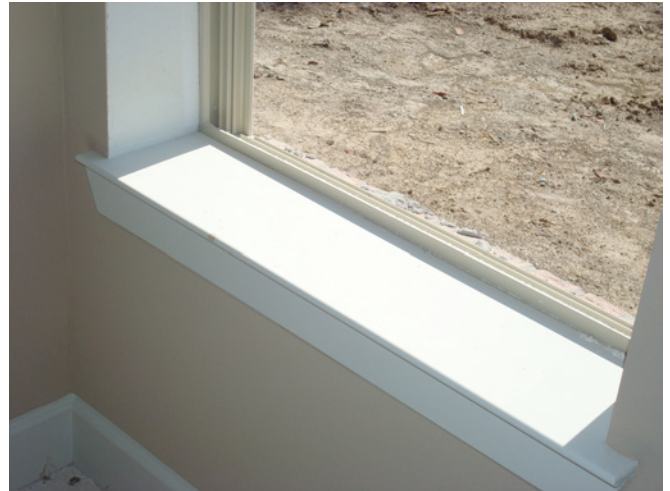
Photograph 9: Deep Window Openings - The combination of advanced framing and insulating sheathing leads to deep window openings. Window returns are typically gypsum board with wood trim only at the bottom.
