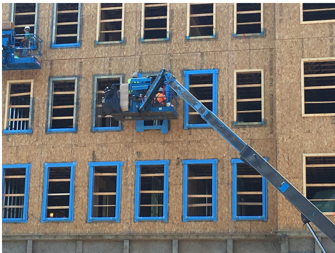
Photograph 2 – Water Proofing the ROESE - The “bump outs” are “water proofed” with “peel and stick” flashing membranes. Note the primer being installed prior to the installation of the “peel and stick” flashing membranes. All good. All very good.
