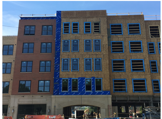
Photograph 3 – ROESE Window Installation - The windows are installed in the openings and a fully adhered water control layer is installed. The fully adhered water control layer is integrated with the flashing membranes at the “bump out” openings. This is all good. Excellent, in fact. No water control issues. None at all. And no air control issues. So what is my problem? It is just that the wood “bump out” is a thermal bridge. What is the point of continuous insulation if we run a thermal bridge through it at every punched opening?
