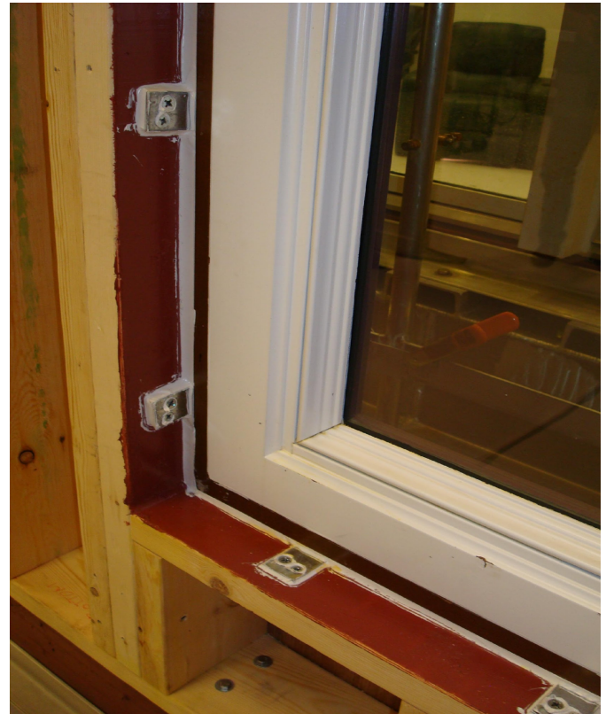
Photograph 7 – High Wind Zone and Seismic Zone Attachment – This window is in the high wind zone of coastal Florida. Straps make it work structurally. In fact that is the only way to install windows in high wind zones and seismic zones regardless of the sheathing type. Note that the thermal bridge goes away when straps are used.
