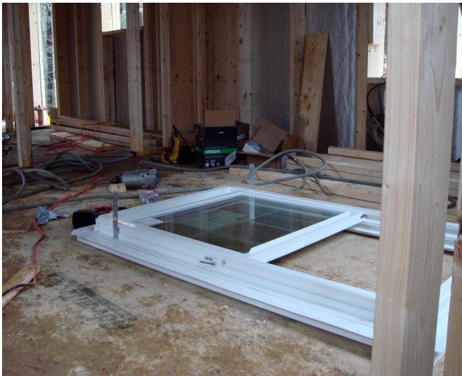
Photograph 6 – Straps - How does the window industry recommend attaching non flanged windows? Straps. Straps baby.....straps. Note in the photograph we are using straps with a flanged window. I can't see how this can possibly be an issue for the manufacturers of windows as they already allow the use of straps. In fact straps are the only means of attachment for non-flanged windows. How can adding straps to flanged windows not work? Exactly. There is no argument against this.
