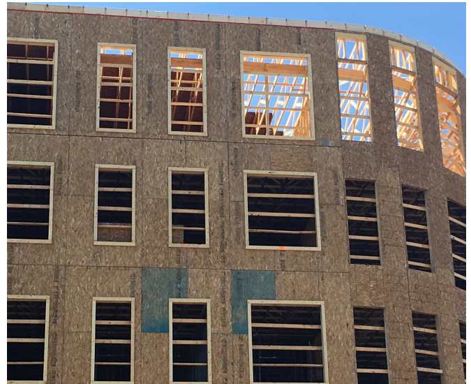
Photograph 1 – ROESE In Action - The wall framing is sheathed with oriented strand board (OSB). The window openings are “picture framed” with a wood “bump out”. The thickness of the wood “bump out” is intended to match the thickness of the continuous insulation to be installed later.
