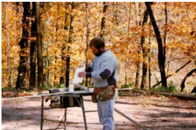
Photograph 4: Sealing End Cuts - Over time coating of the back surfaces of siding was extended to the cut ends of siding and trim. Wood is anisotropic...it absorbs water differently based on the grain/fiber direction. Cut ends absorb way more water than the face of siding and trim. Painting of cut ends became necessary to control decay of wood and wood based claddings as it reduced water absorption.
