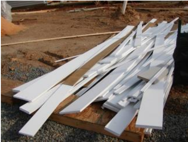
Photograph 10: Modern Trim - Today virtually all wood trim and engineered wood claddings, fiber cement and composites come coated on all six sides or protected on all six sides.
