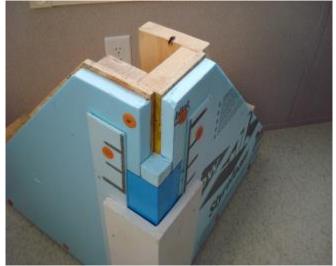
Photograph 11: Air Gap – Not complicated with continuous insulation less than 1 1/2 inches thick. The spacer strips are 1/4 inch to 3/8 inch strips of foam or sill gasket material. No issues. Easy.
