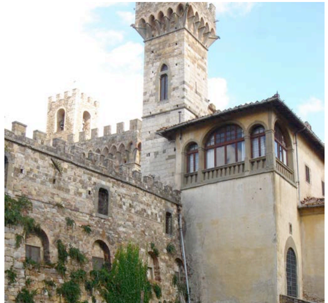
Photograph 1: French Chateau —A nice place to store wine is in its cellar.
