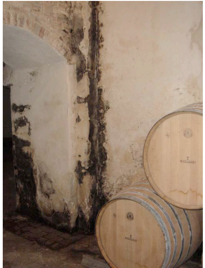
Photograph 5: Mold in Cellar —I am shocked, just shocked to see mold in a cellar. One of the reasons French wine tastes differently than California wine...
