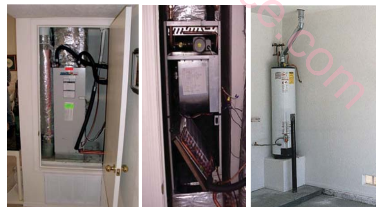
Air handler closet located in hallway
