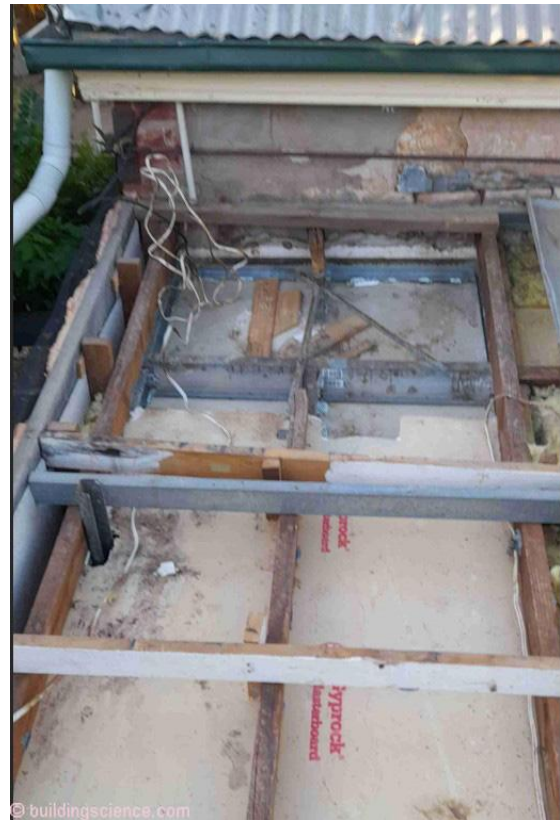
Photograph 7: Insulated deteriorating Australian roof (photo Courtesy Jessica Allen, Climasure, Australia)
