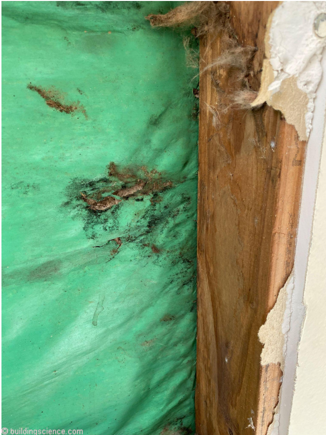
Photograph 6: The drying potential of the exterior claddings was reduced and lead to decay and mold
