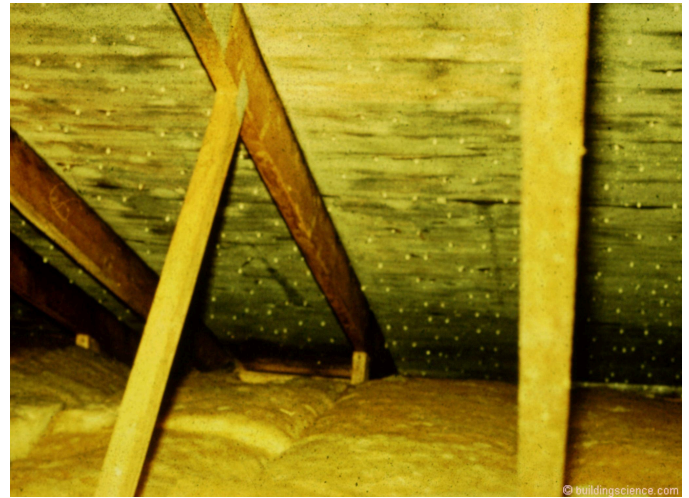
Photograph 1: Attic rot in a Canadian attic – thank you CHIP
