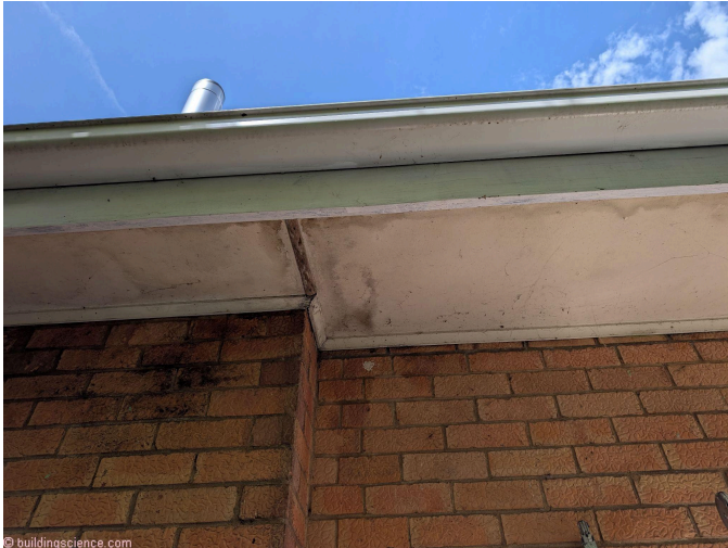
Photograph 9: More soffit condensation damage (photo Courtesy Jessica Allen, Climasure, Australia)
