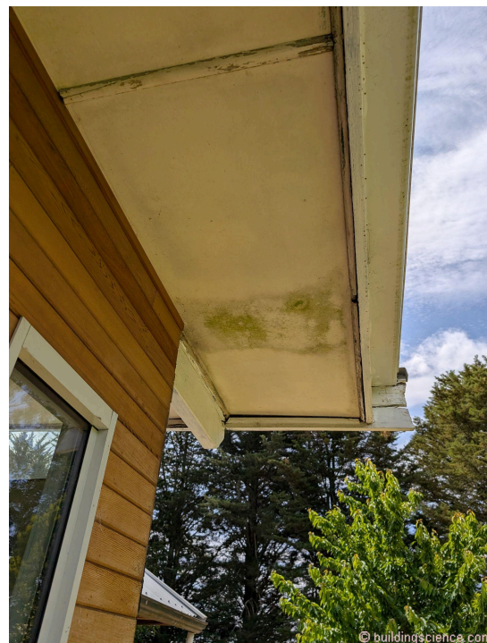
Photograph 8: Soffit condensation damage (photo Courtesy Jessica Allen, Climasure, Australia)
