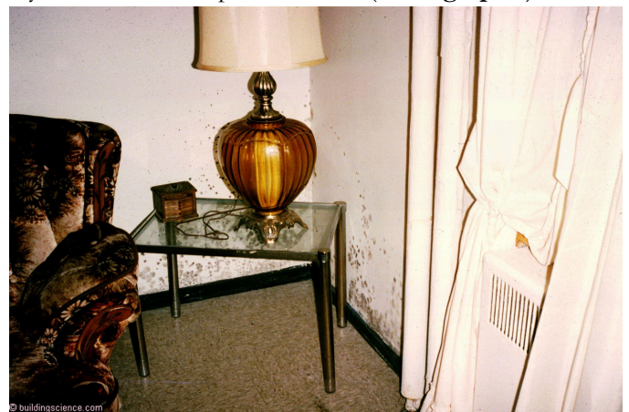
Photograph 2: Interior surface mold in a Canadian home – thank you CHIP and COSP
