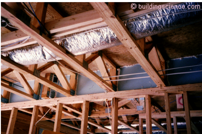
Photograph 4: Gypsum board blocking used with a floor truss assembly. Note the location of a vertical member within the floor truss
