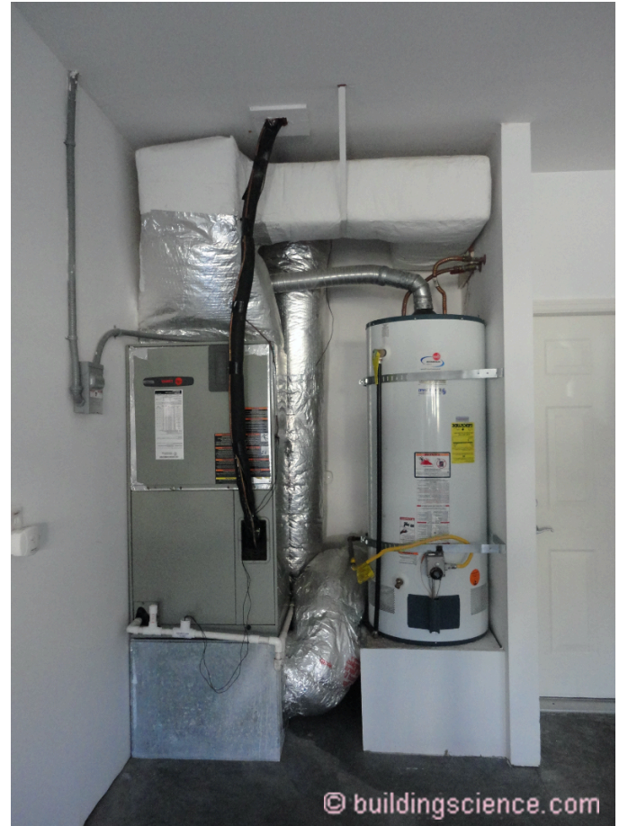
Photograph 8: Mechanical air distribution systems (forced air furnaces/AC units) and associated ductwork should not be installed in attached garages due to the potential risk for air leakage of such systems drawing air from garages into occupied unit spaces
