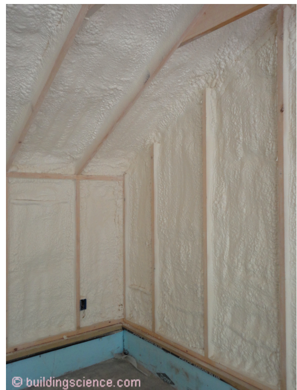
Photograph 7: Spray foam cavity insulation on the walls separating the garage from the exterior. Again, note that the wall assembly will need to meet the applicable fire rating requirements.
