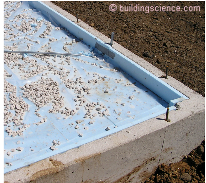
Photograph 6: Insulation detail at the stem wall portion of the garage foundation.
