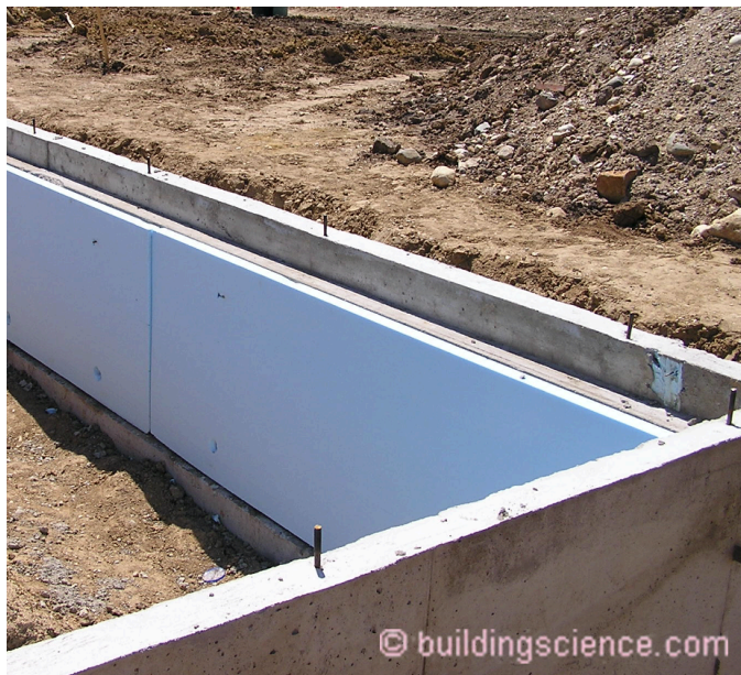
Photograph 5: Insulation detail at the stem wall portion of the garage foundation.
