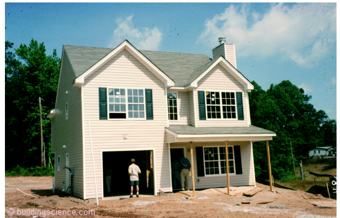
Photograph 1: Garages are often “tucked in” to houses typically with living space/conditioned space above the garage
