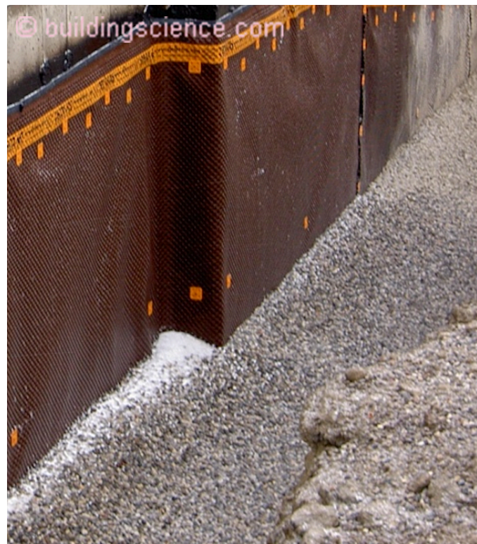
Photograph 1: Drainage layer located on exterior of the waterproofing
