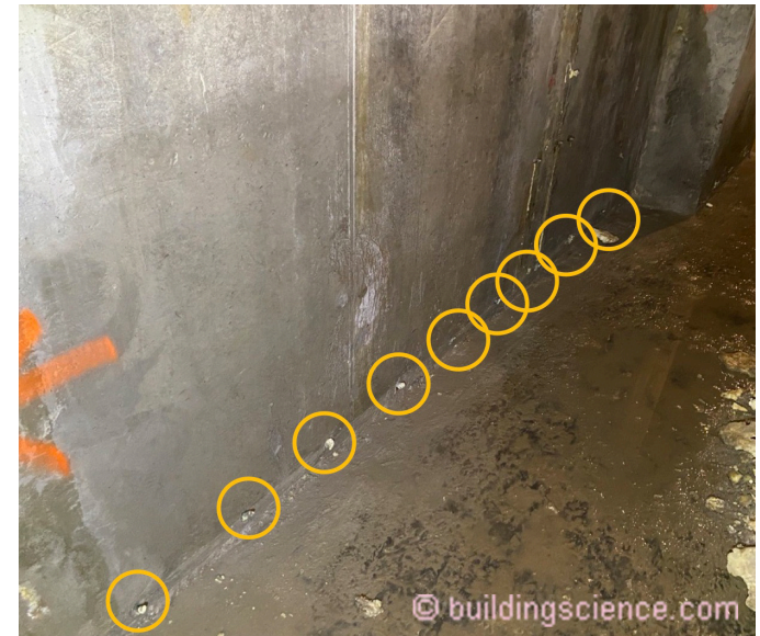
Photograph 2: Injection sealing for “spot” ground water leakage
