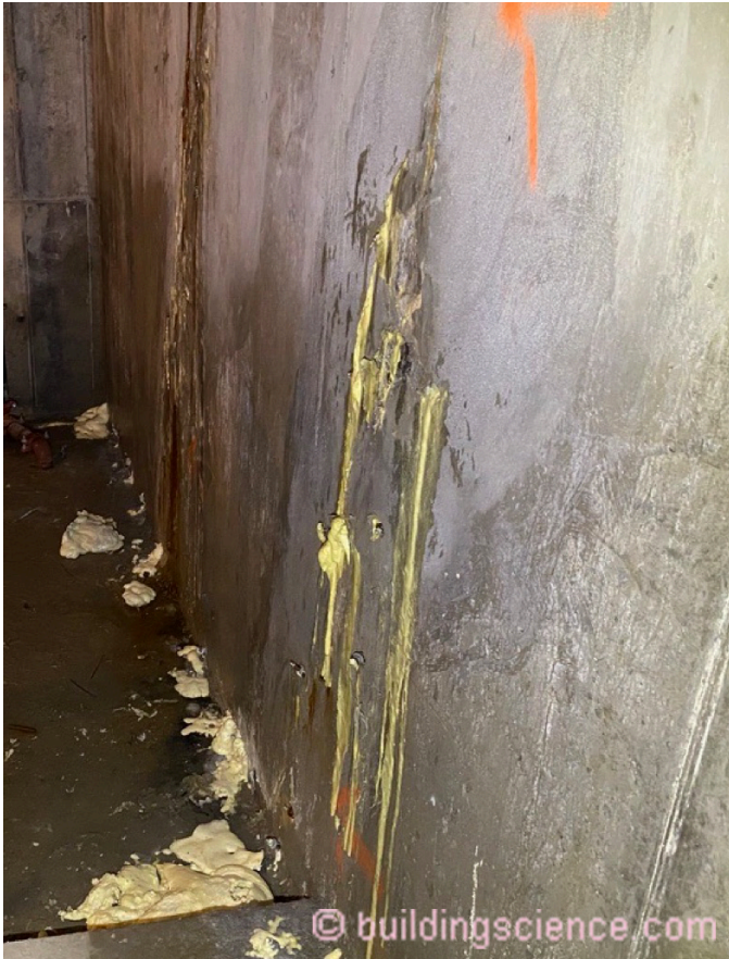
Photograph 3: Injection sealing for “intermittent” ground water leakage
