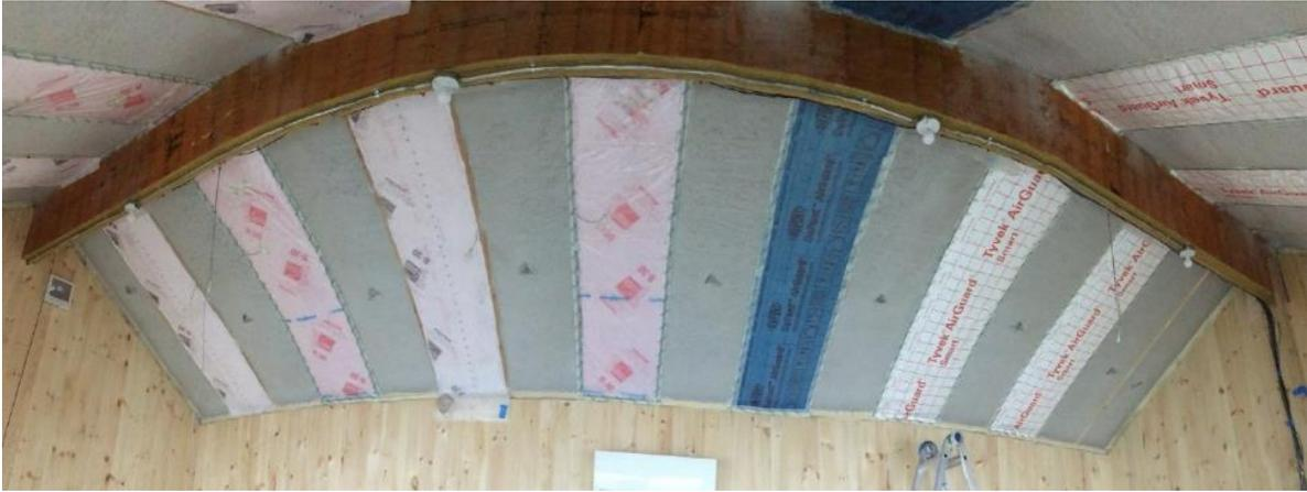
Figure 18. North-facing roof bays after vapor control membrane installation
