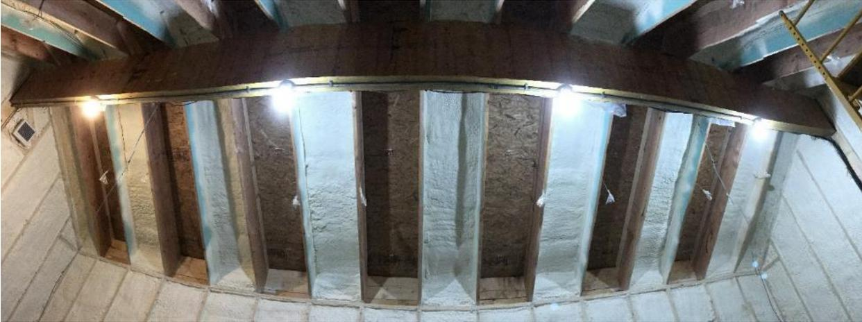
Figure 16. North-facing roof bays after spray foam installation
