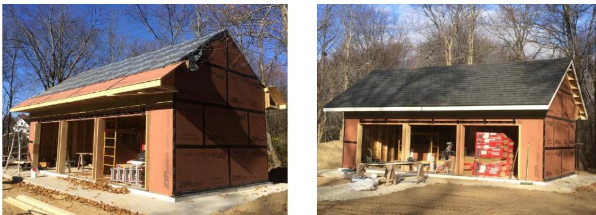
**Figure 11.** Self-adhered underlayment (left) and asphalt shingles (right)
