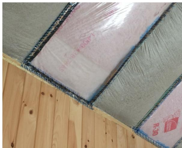
**Figure 130. Roof 3 north vapor retarder failure (January)**
