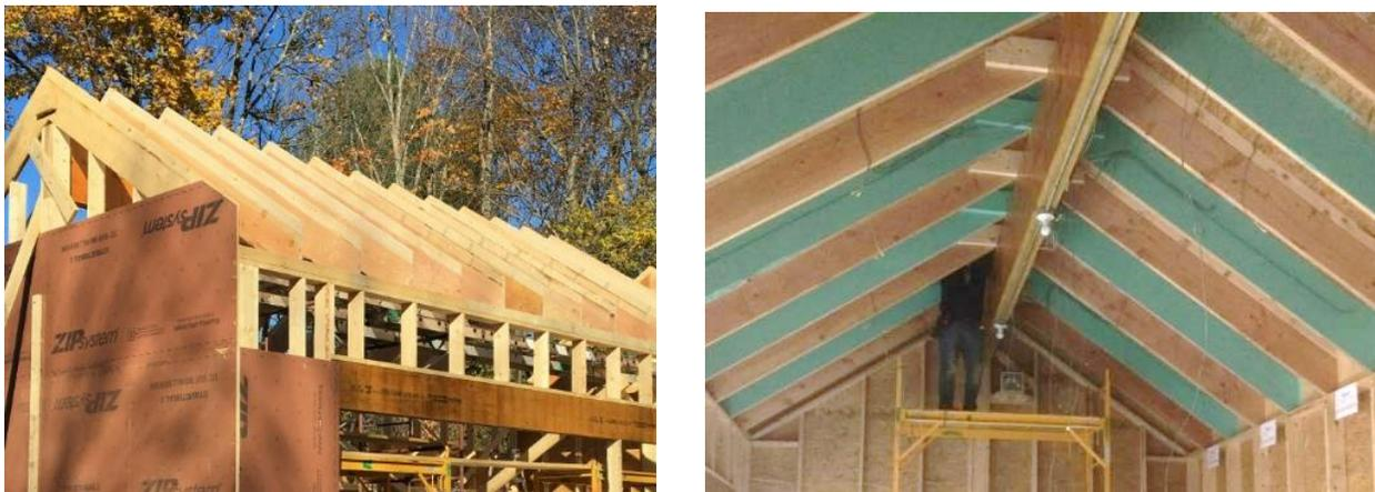
**Figure 10.** 2x12 and 2x4 rafters (left), air and vapor barrier on guard bay rafters (right)
