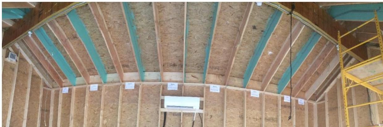
**Figure 15. North-facing roof bays after instrumentation**
