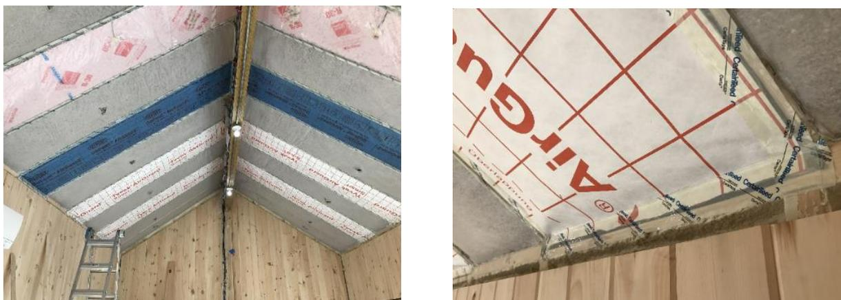
Figure 13. Interior vapor control membranes (left), double-tape air sealing detail (right)
