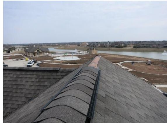
**Figure 3. Houston diffusion vent showing ridge condition**
