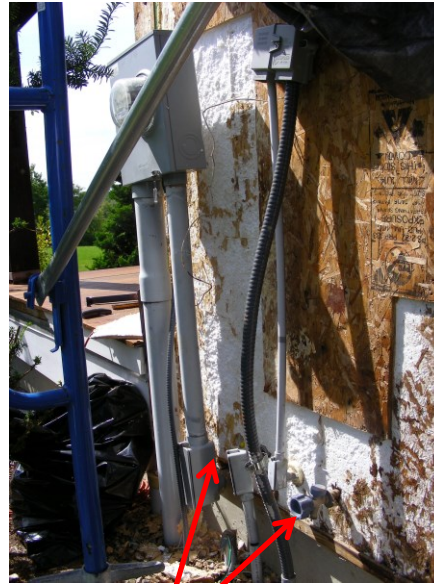
No sealant at the electrical penetrations
