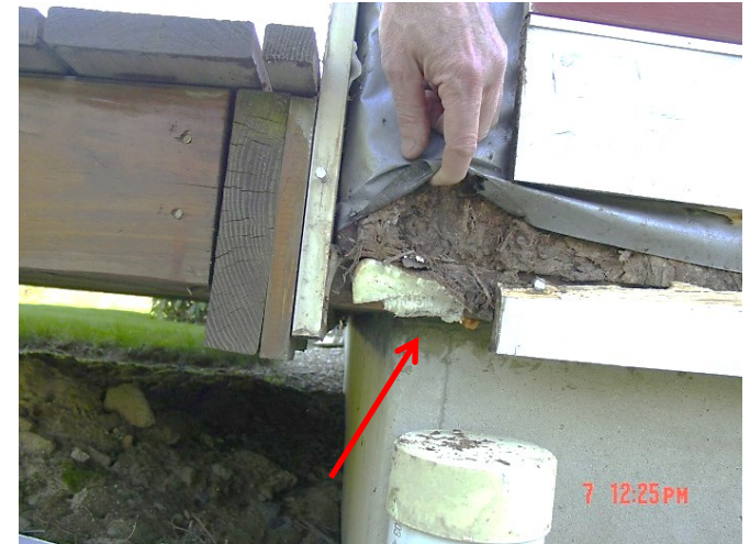
No sealant at the electrical penetrations
