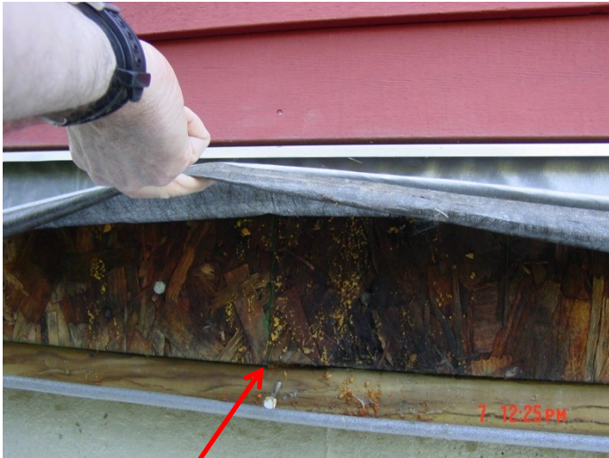
No sealant at the sill
