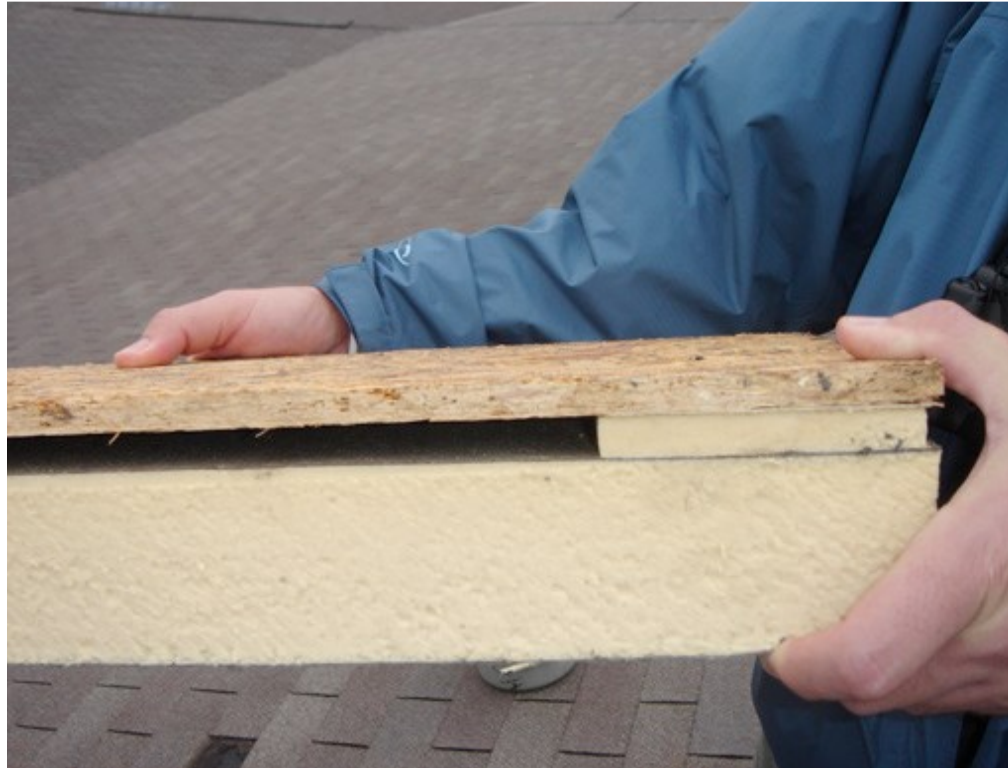
Photograph 8: Vented Foam Panel —The upper panel surface is OSB that acts as a nail base for shingle and other roofing systems.
