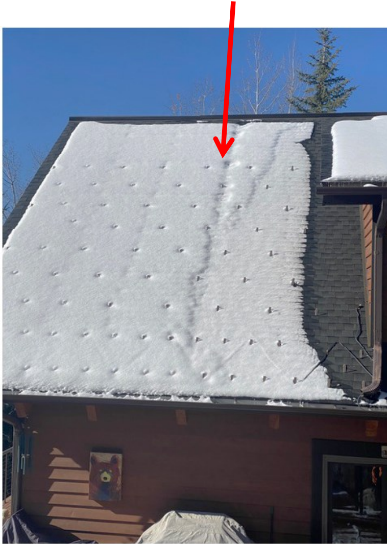
Photograph 1: The vertical snow melt lines correspond with the SIP assembly joints
