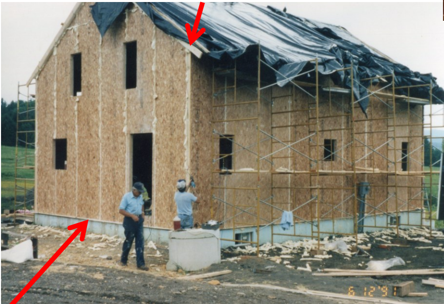
These wall panels cover the rim joists
