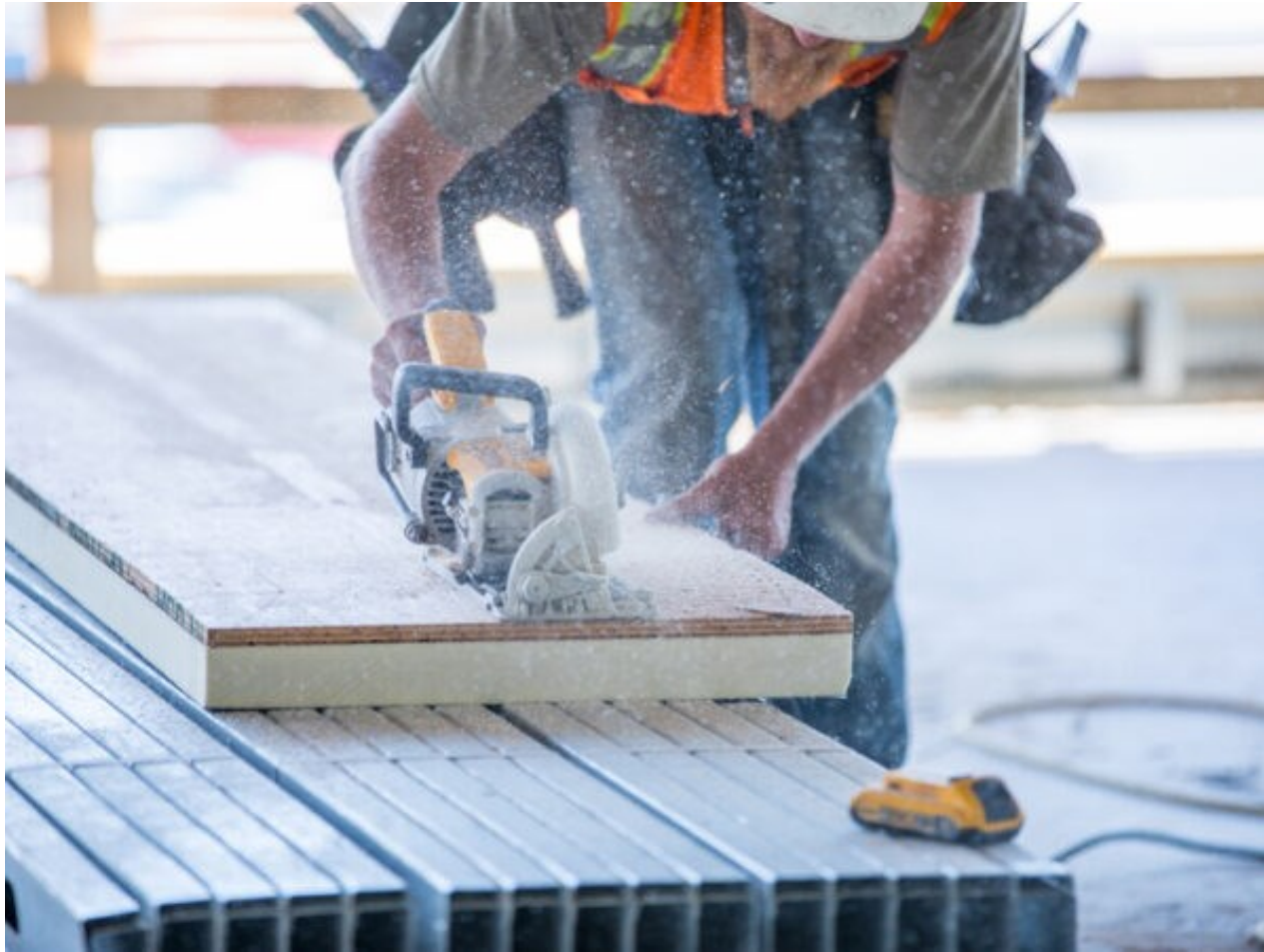
Cutting SIPs to size
