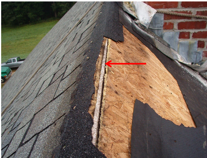
No sealant at the sill
