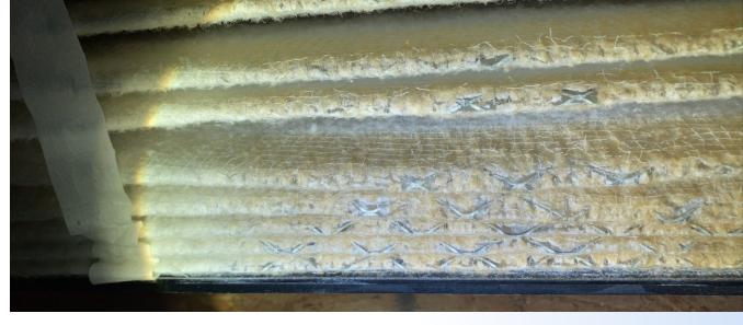
UV/PCO damage to HVAC components
