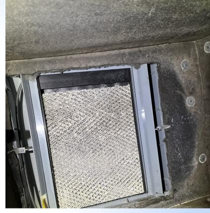
Humidifier discharge into porous liners
