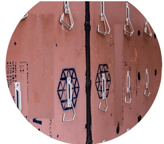
Direct attachment of cladding
