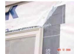
Head flashing at new window
