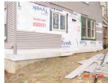
Siding removed to remediate flashing
