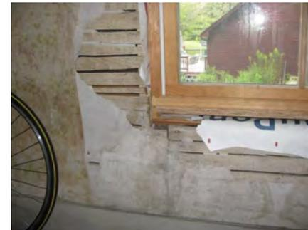
Existing replacement windows installed without flashing
