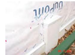
Drainage plane remediation at base of wall
