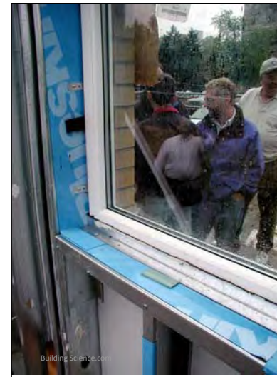
Continuous interior angle provides backdam and airtight continuity
