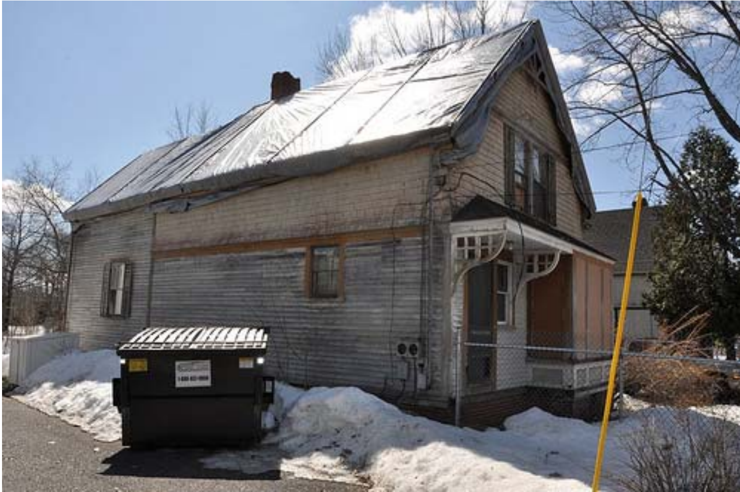
57 Depot Street prior to construction
