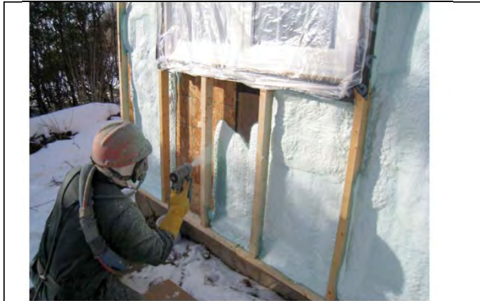
Figure 15 : Installation of high density spray foam in an Offset Framed Wall in a cold climate
