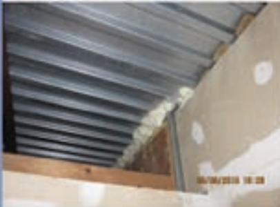
Assess opening size and select material consistent with the QAS Manual. Complete any roof-wall joint opening into the sides of the space.
