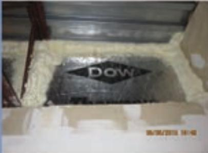
Fasten all edges and air seal in place. In this instance adhesive 2-component foam has done both tasks - Smart!
