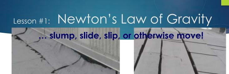
And the effects of gravity can be magnified by other factors... such as asphalt type (softening point), amount of adhesive, temperature, etc...
