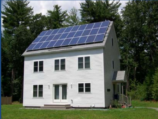
A Custom Home in Stow, MA 15 ½ thick walls, Air infiltration of .50 ACH @50 pascals
