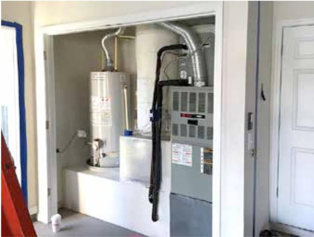
**Photograph 4: Gas Water Heater and Gas Furnace In Closet—**Standard gas water heaters and gas furnaces need combustion air—basically a big hole connecting the closet to the garage. Defeats the purpose which was to stop the sweating.
