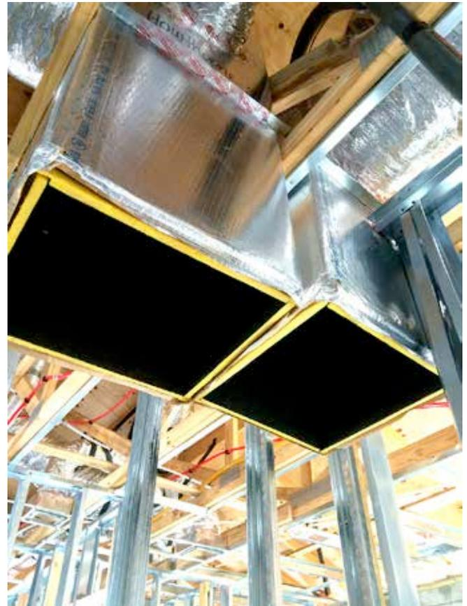
**Photograph 9: Rigid Duct**—Go with rigid duct as it is much easier to seal where it penetrates ceilings.
