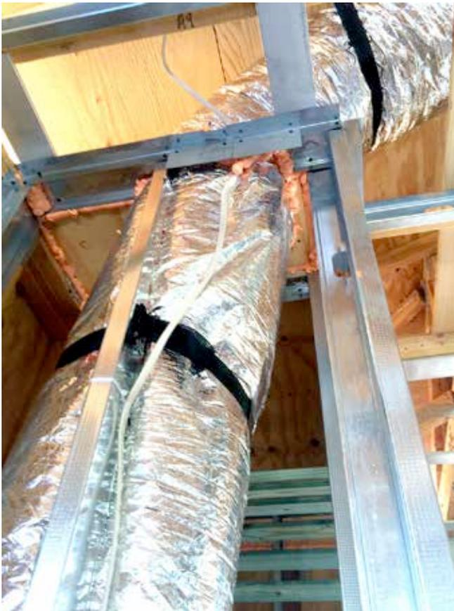
**Photograph 8: Flex Duct**—The mechanical closet is going to be slightly negative. The ductwork penetrating the ceiling needs to be sealed in an airtight manner if the ceiling is at the underside of a vented attic. You do not want to pull hot humid air down into the mechanical closet from the attic. The supply and return ductwork should not be flex duct as it is extremely difficult to seal.
