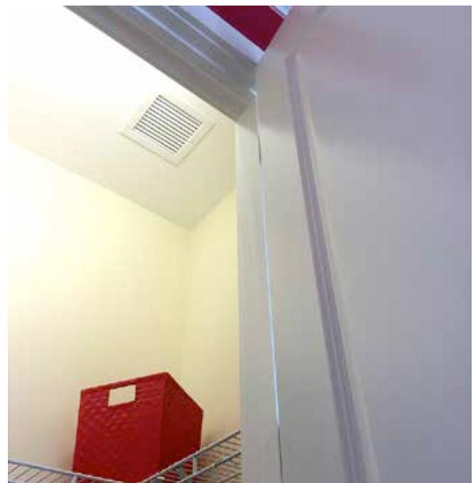
**Photograph 12: Closets Need Returns**—What spaces have the least load? Closets. Closets need “active” returns at the ceilings and undercut doors. Closets are now getting colder.
