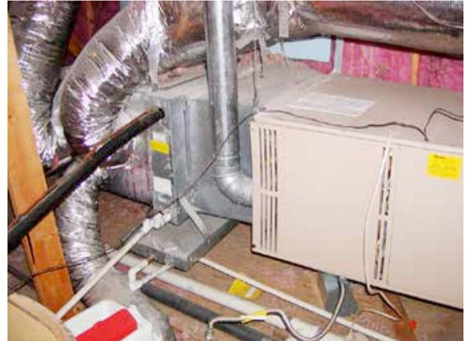
**Photograph 1: Air Handler in Attic**—The worst thing you could do is install furnaces and air conditioning systems in vented attics. The attics are way hotter than the outside in the summer and cold and miserable in the winter—and in hot humid climates it gets ugly. You can't get at them easily to service them. They don't last very long. They need to be in a better place.
