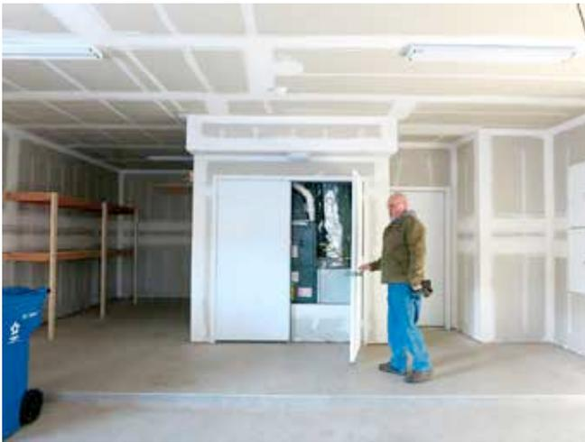
**Photograph 5: Sealed Combustion—**If the gas furnaces are sealed combustion and the water heaters are sealed combustion then transfer air from the garage is not necessary. Great approach...except... closet gets cold.
