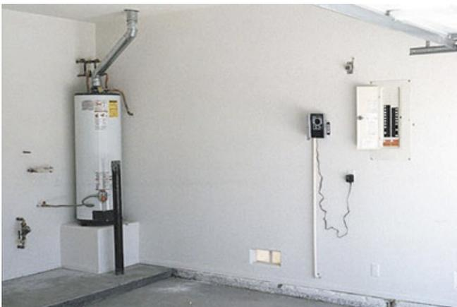
**Photograph 6: Lonely Water Heater—**Leaving the standard gas water heater outside of the closet solves the combustion air problem for the gas water in the closet as does changing the gas water heater for an electric water heater.
