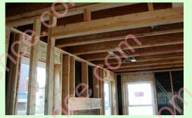
Above: Single top-plate, 24-inch o.c. in-line framing and metal cross bracing
