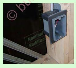
Left: Air tight electrical box and cross bracing
