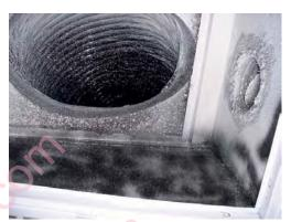
Outside air duct connected to return duct; note outside air damper on right
