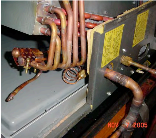
Figure 14: TXV bulb permanently strapped and insulated
