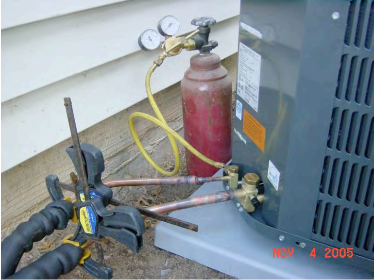
Figure 9: Brazing connections at outdoor unit with nitrogen flowing internally
