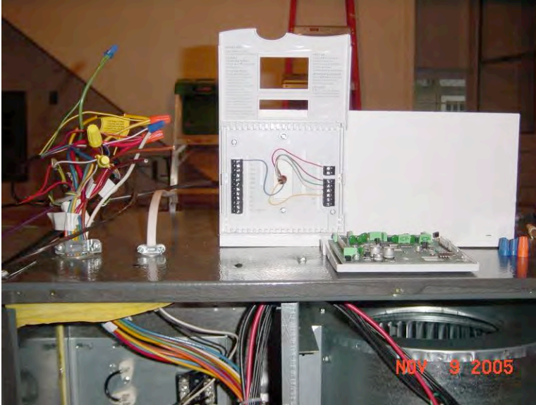
Figure 18: Low-voltage controls wired; thermostat and air handler unit settings configured
