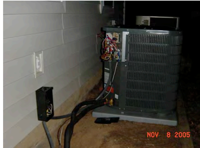
Figure 16: Indoor and outdoor units electrically wired
