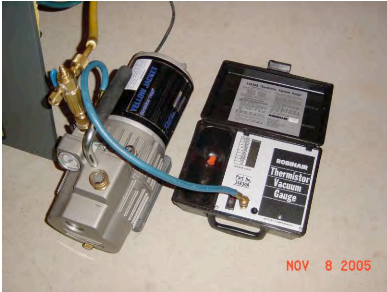
Figure 13: System evacuation with 2-stage vacuum pump and digital vacuum gauge
