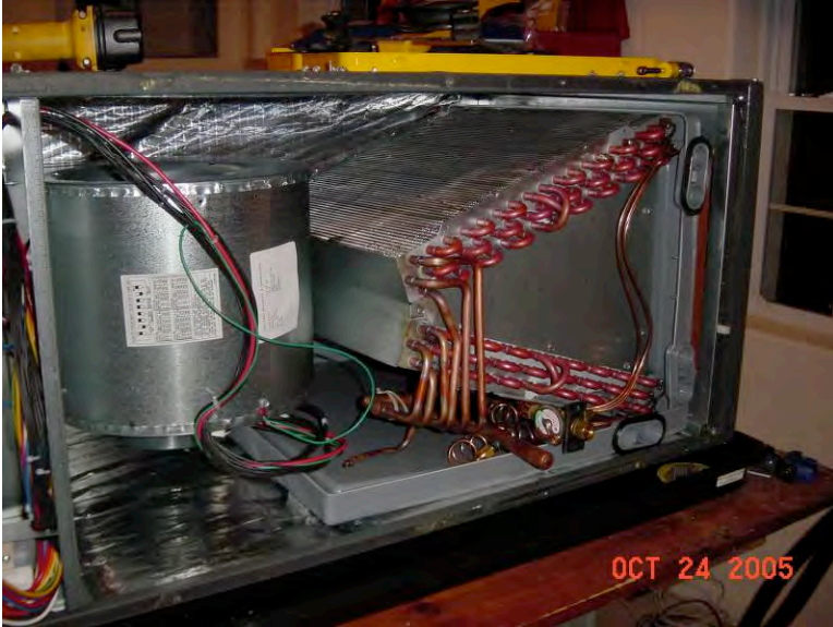
Figure 7: Indoor unit with ECM blower and evaporator with TXV
