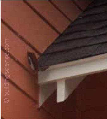
Figure 3. Kick-out flashing at roof-wall intersection
