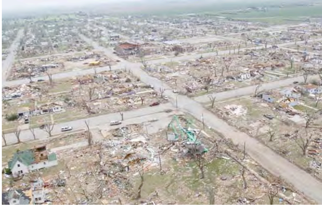
Figure 1.1: Aerial Photograph of Tornado Damage at Greensburg, KS (source: Jaime Oppenheimer/The Wichita Eagle)
