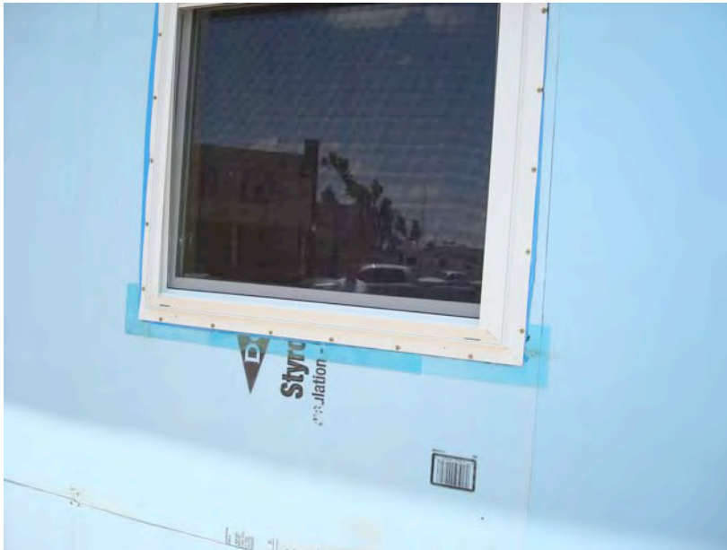
Figure 4.9: Photograph of partially complete window flashing. Pan flashing visible under window.
