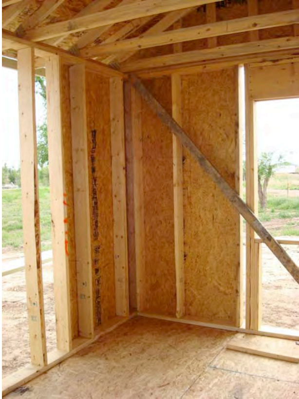
Figure 4.5: Photograph of OSB shear panel at corner of advanced frame wall
