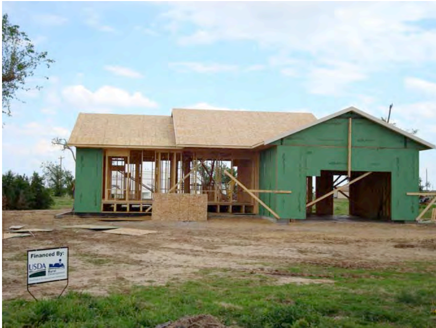
Figure 4.6: Photograph of complete advanced framing with OSB shear panels.
