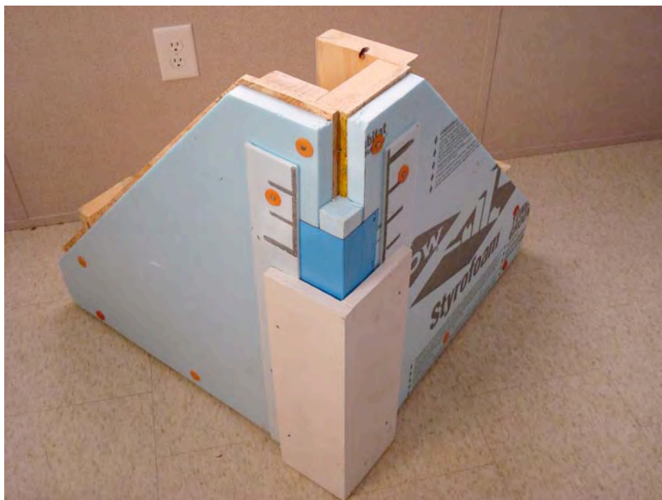
Figure 5.1: Photograph of two-stud corner with insulating sheathing and trim mock-up
