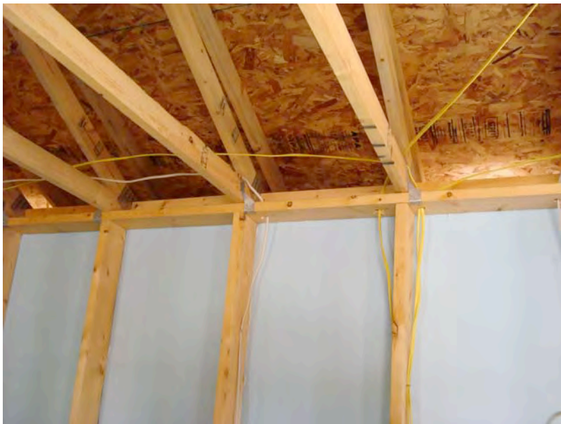
Figure 4.8: Photograph of stacked roof and wall framing
