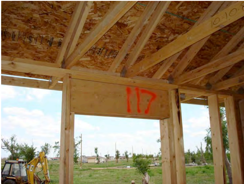
Figure 4.4: Photograph of advanced framed opening in load-bearing wall
