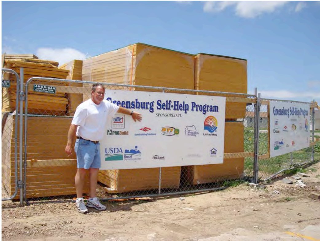
Figure 4.1: Photograph of Self-Help Housing Program board with Dow foil-faced insulation piled behind
