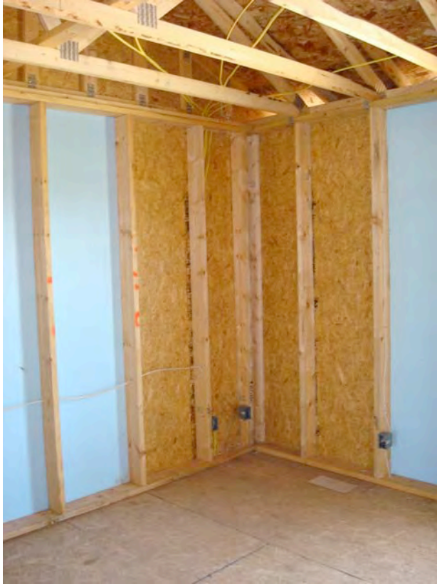
Figure 4.7: Photograph of OSB shear panel with insulating sheathing over advanced frame wall
