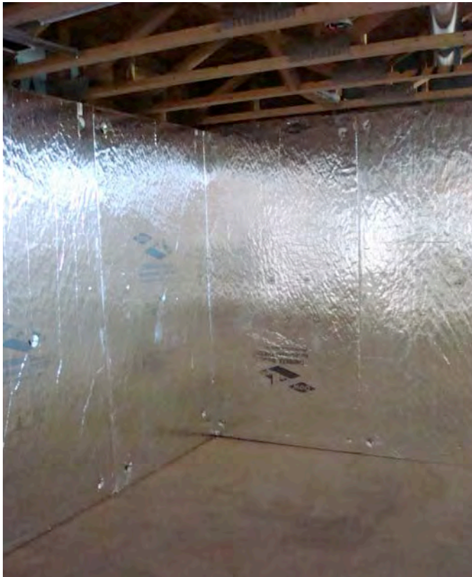
Figure 4.2: Photograph of basement insulation system
