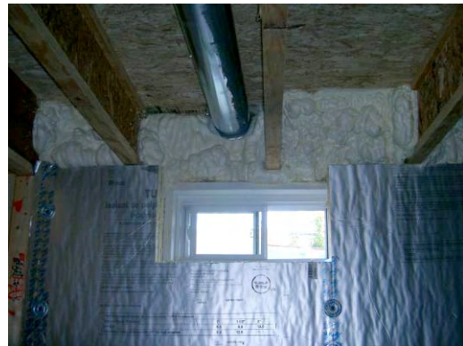
Figure 1.35: High density spray foam air seal around enclosure penetration
