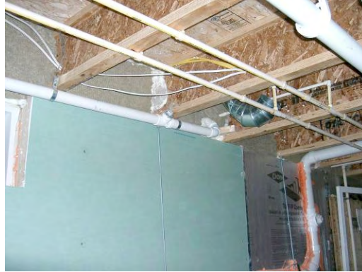
Figure 1.40: Gypsum board over foil-faced foam
