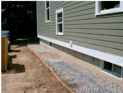
Figure 1.34: Gravel drainage and “no-planting zone” perimeter
