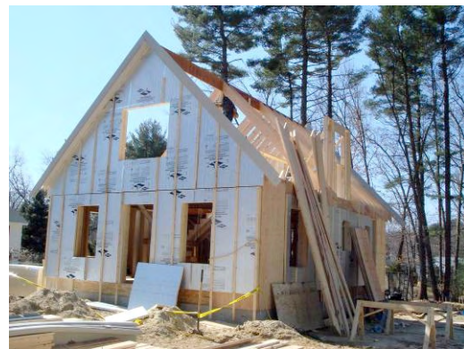
Figure 1.29: Framing, foam and furring strips
