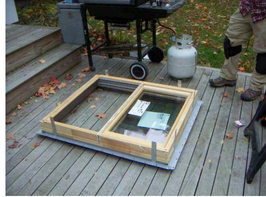
Figure 1.19: Metal strap attachment for window-to-frame connection
