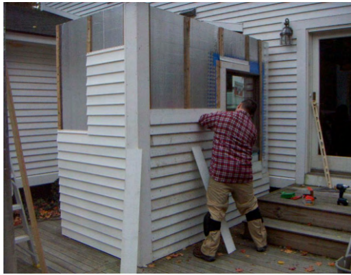
Figure 1.14: Exterior mockup construction (wood and vinyl siding attachment)
