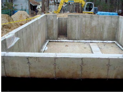
Figure 1.26: Foundation walls
