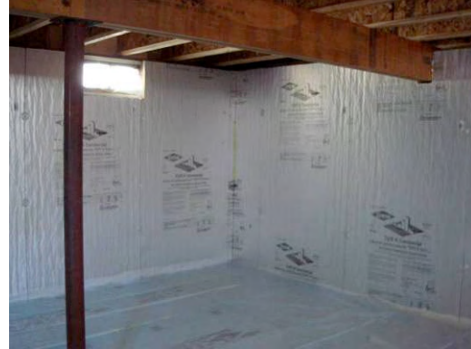
Figure 1.27: Basement insulation
