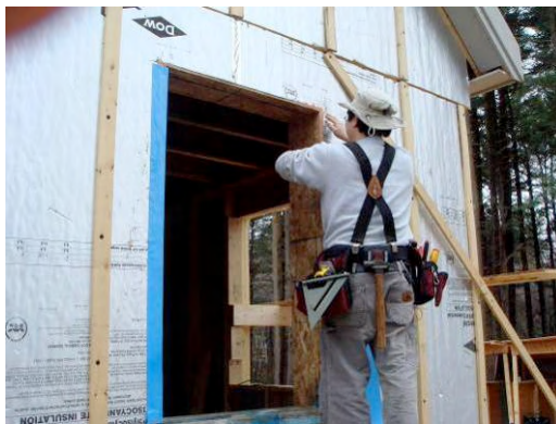
Figure 1.38: Kohta Ueno from BSC flashing a window opening
