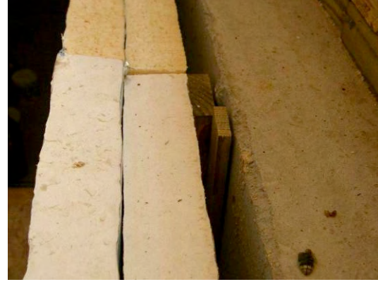
Figure 1.25: Close-up of basement foam detail (pre air sealing)
