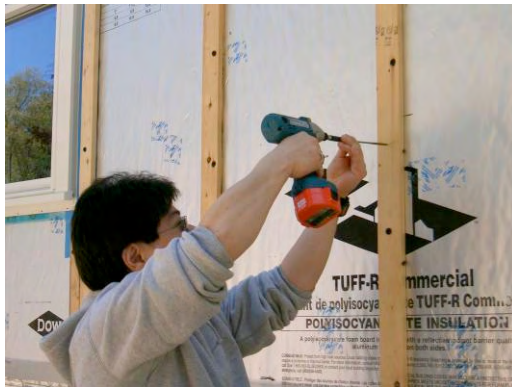
Figure 1.30: Kohta Ueno from BSC testing a furring strip fastener
