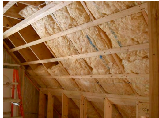
Figure 1.31: Roof insulation
