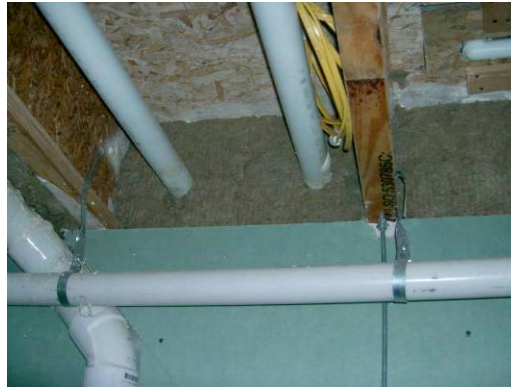
Figure 1.38: Roxul insulation over spray foam at rim joist
