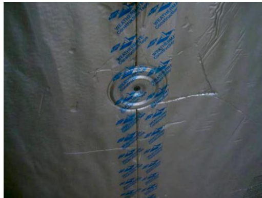
Figure 1.39: Roofing washers fastening foil-faced foam to furring strips
