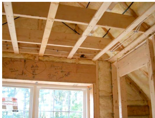
Figure 1.41: Second floor strapping and collar ties
