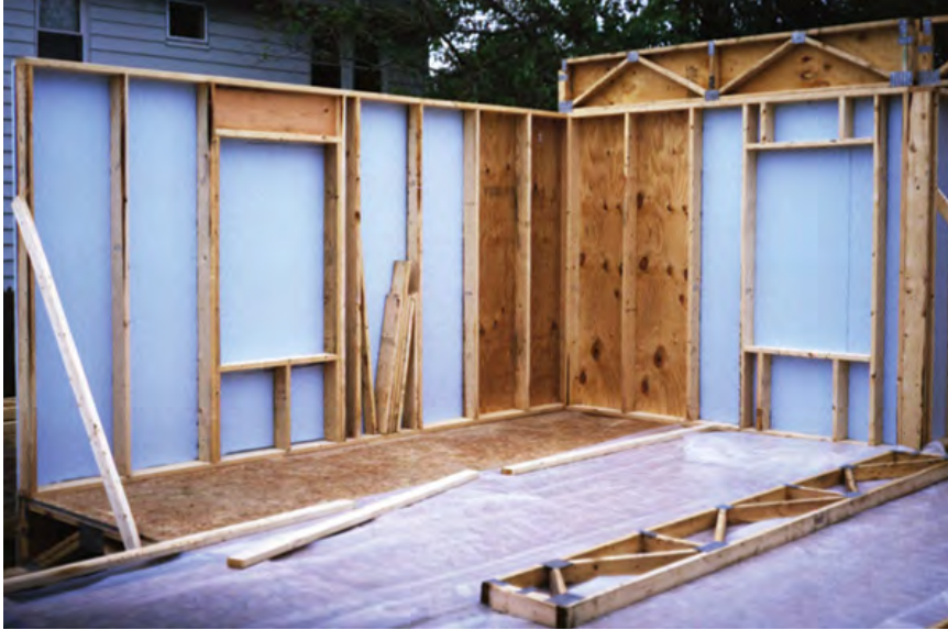
Figure 6: Exterior Walls Non-Load Bearing Headers Removed
