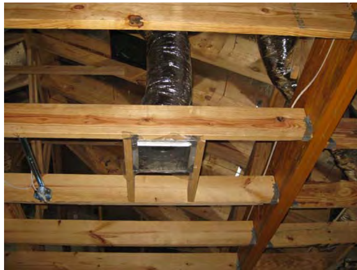
Figure 1 - supply boot with duct mask
