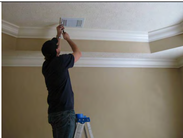
Remove supply register.
