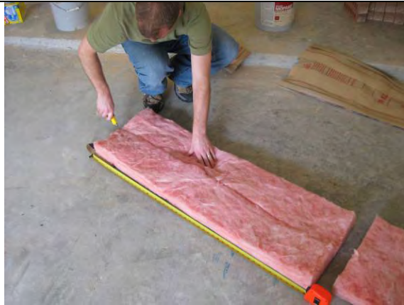
Cut fiberglass in half lengthwise.
