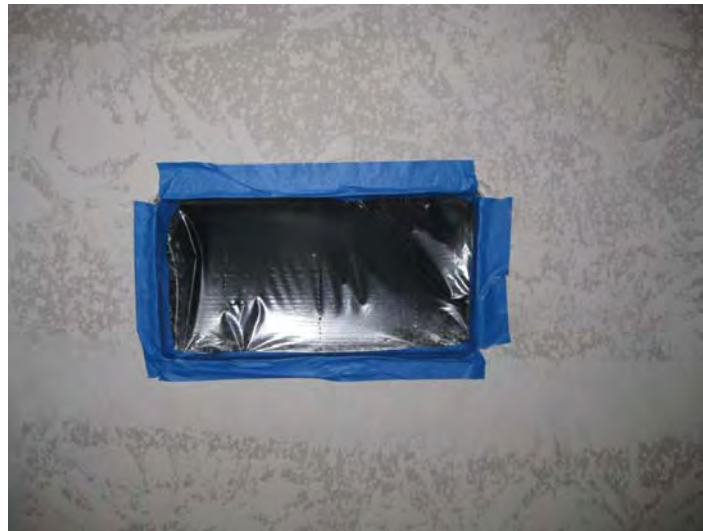
Figure 2 - Supply boot with duct mask adhered to inside of flange
