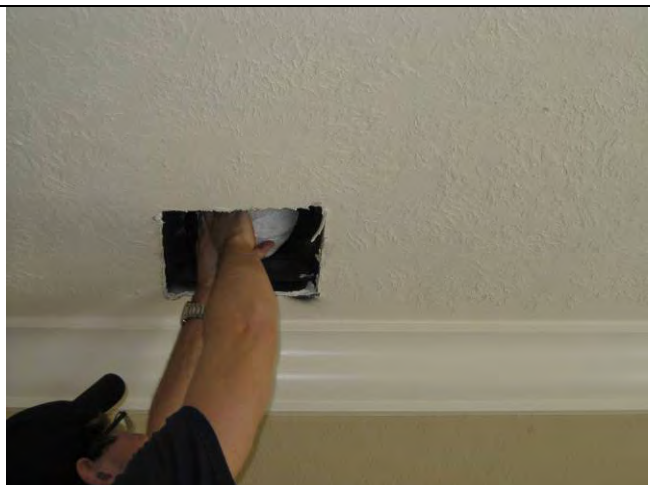
Compress fiberglass cylinder and place in supply
