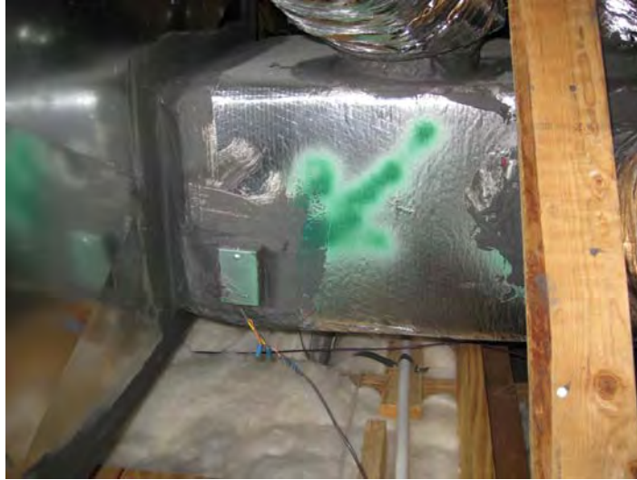
Figure 3 - Remedial duct sealing at area noted by Energy Sense
