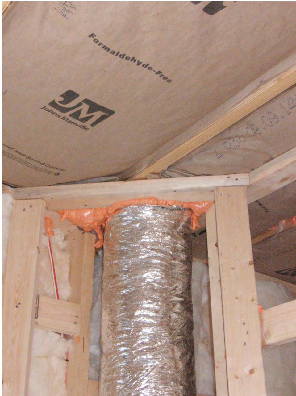
Airsealing HVAC Penetrations to Unconditioned Attic
