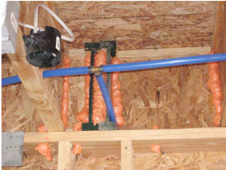
Figure 3.3.5: Framing and Plumbing Penetrations Sealed at Garage Wall
