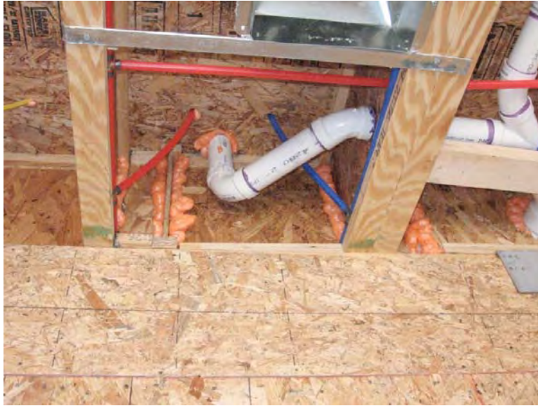
Figure 3.3.6: Framing and Plumbing Penetrations Sealed at Garage Wall
