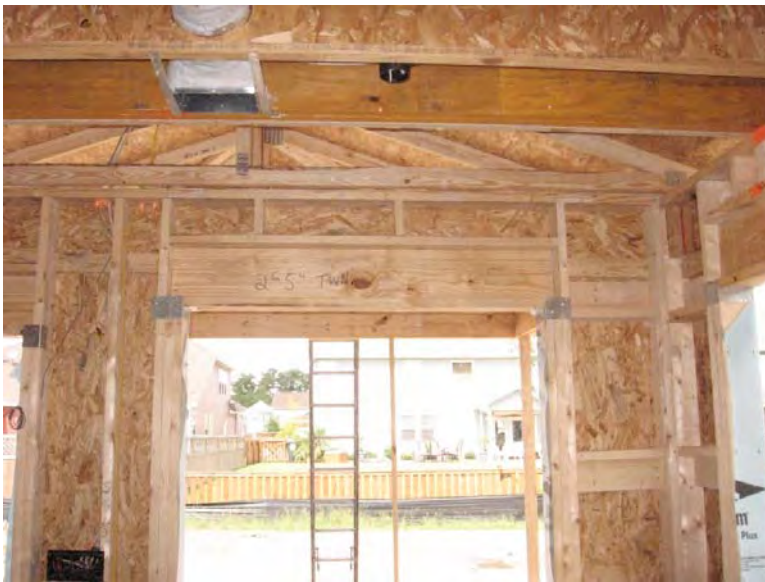
Figure 3.3.3: Header in Non-Load Bearing Wall
