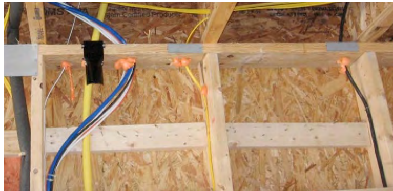
Figure 3.3.7: Electrical Penetrations Sealed at Top Plate
