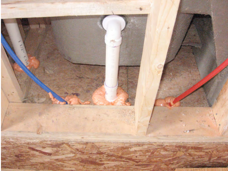
Airsealing of plumbing penetrations
