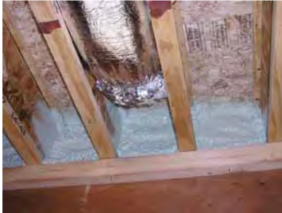
Figure 1.3.7: Closed cell spray foam at rim joist
