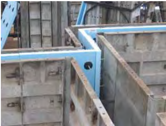
Figure 1.3.5: Thermomass foundation system
