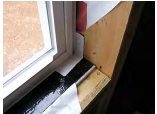
Figure 1.4.2: Window installation at sill
