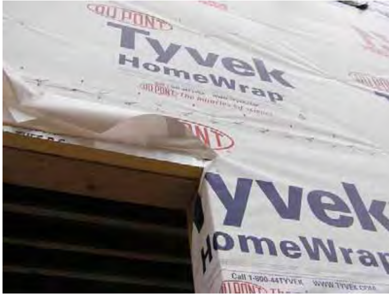
Figure 1.3.4: Tyvek ® installed over 2" foil-faced polyisocyanurate
