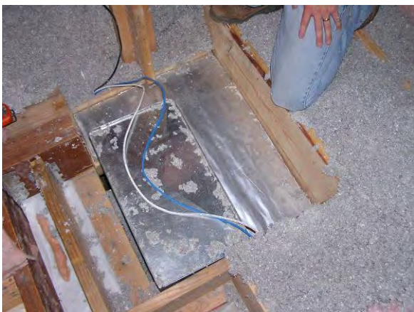
Figure 9: Polyiso cut and fit into opening
