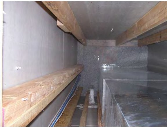
Figure 8: Blocking in duct chase at first to second floor interface
