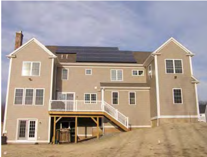
Figure 1.3.13: Lot 4 with 7kW PV array installed on the South facing roof
