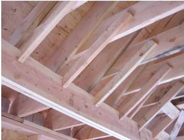
Figure 1.3.3: Dropped ceiling soffit framing
