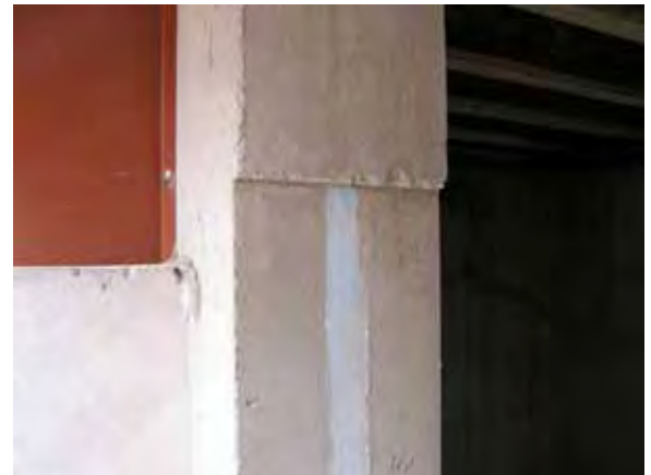
Figure 1.3.6: Insulation at bulkhead door opening
