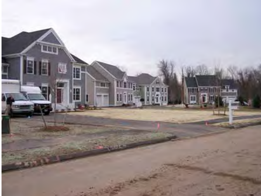
Figure 1.2.1: Completed houses at Hamilton Way
