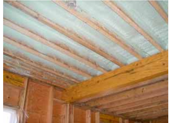
Figure 1.3.8: Closed cell spray foam floor over the garage
