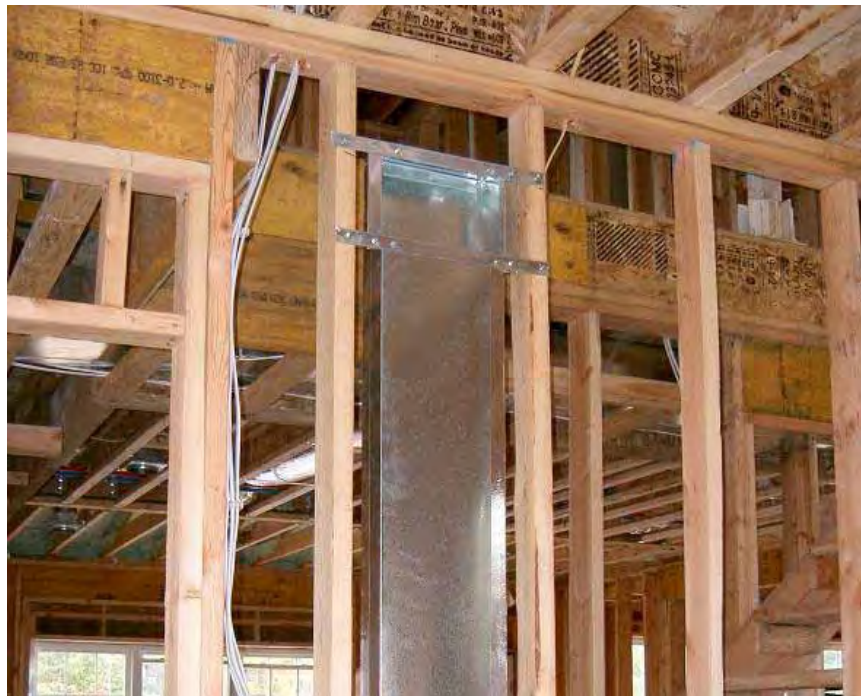
Figure 1.4.5: High wall register roughed in
