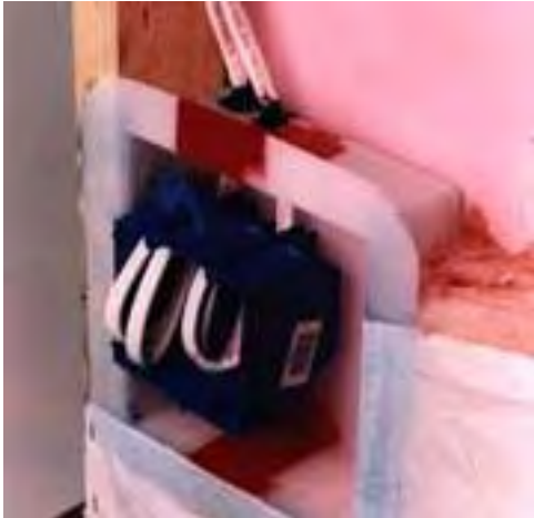
Figure 3: Airtight Electrical Box Pan (Photo courtesy of LESSCO)
