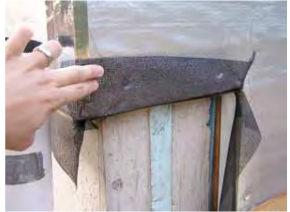
Figure 1.4.4: Installation of insect screen at foundation
