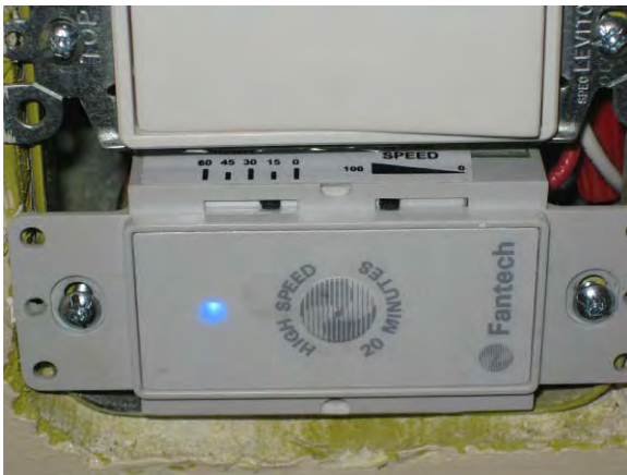
Figure 12: Fantech Venttech switch; note left hand slider (60 to 0)—minutes runtime/hour
