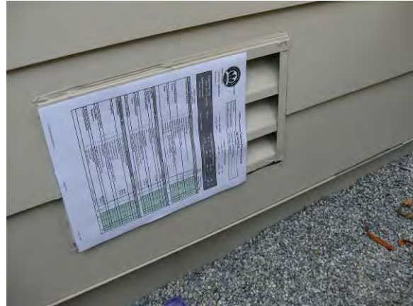
Figure 7: Suction at economizer damper due to leakage past damper
