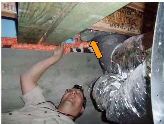
Figure 10: Removed 4" duct from outdoor air (economizer/free cooling) box
