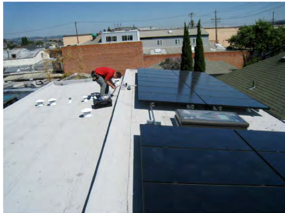
Figure 10.3.26: Installation of solar radiation sensor during data acquisition system setup
