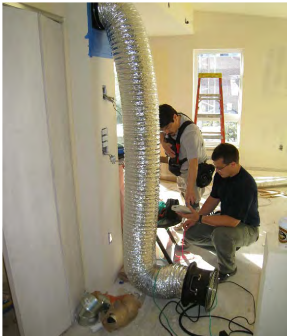
Figure 19: Duct leakage testing, showing fan
