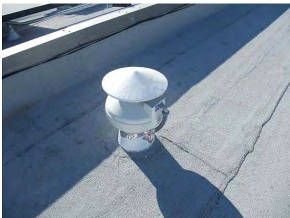
Figure 10.3.16: Fantech FR150 inline fan retrofitted on HRV exhaust side
