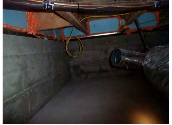
Figure 10.3.6: Interior view of conditioned crawl space ("thermal basement")
