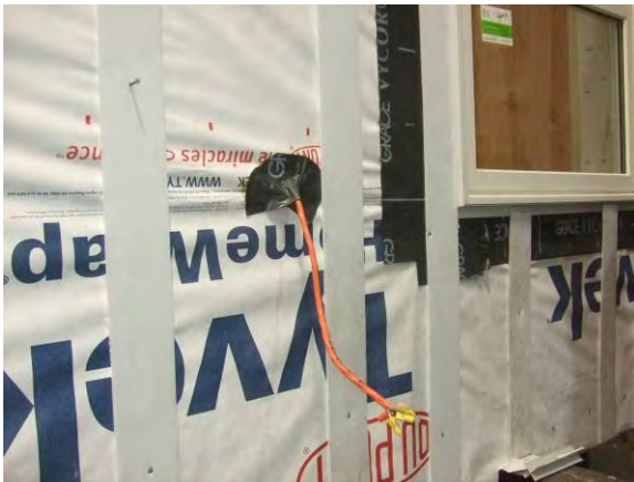
Figure 2: ZETA current 1/4" rainscreen practice using plastic corrugated sign board
