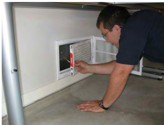
Figure 2: Removal of return grille filters
