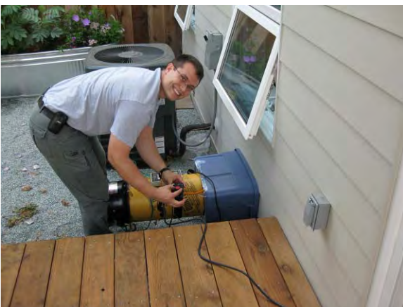
Figure 4: Measurement of economizer flow
