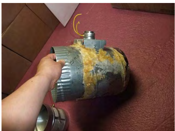
Figure 14: Example of 10” motorized damper with stops and gaskets
