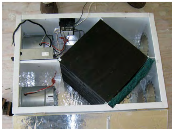
Figure 10.3.15: Interior of HRV, showing heat exchanger (plastic core) and filter
