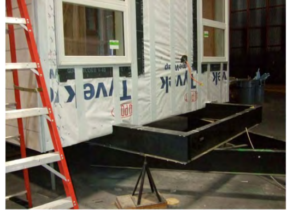
Figure 10.5.8: Plastic “sign board” furring strip installation at lap siding portions
