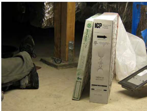
Figure 1: MERV 13 2" filter vs. MERV 8 4"
