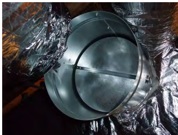
Figure 13: Motorized damper shown without any stop or gasket installed
