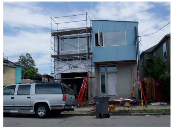
Figure 10.4.4: Site finishing work on assembled modules (June 2009)
