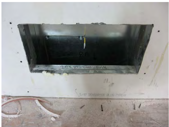
Figure 29: T/RH sensor installed in first floor return duct
