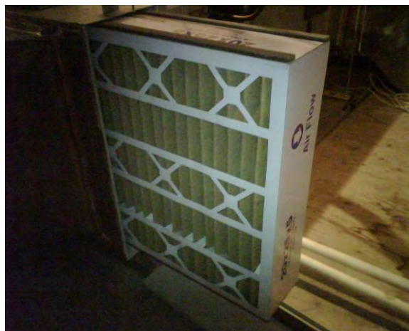
Figure 18: Example of 20x25x5 filter used in Air Bear housing
