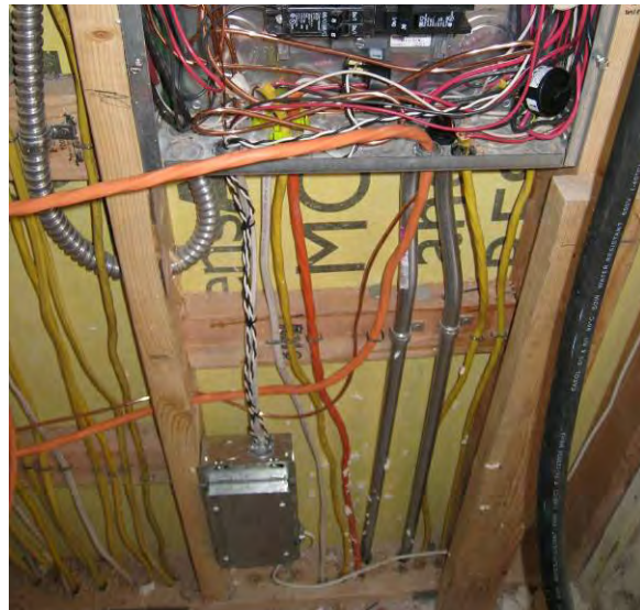
Figure 39: Watt-hour transducer for outdoor HVAC unit (in lower electrical box)
