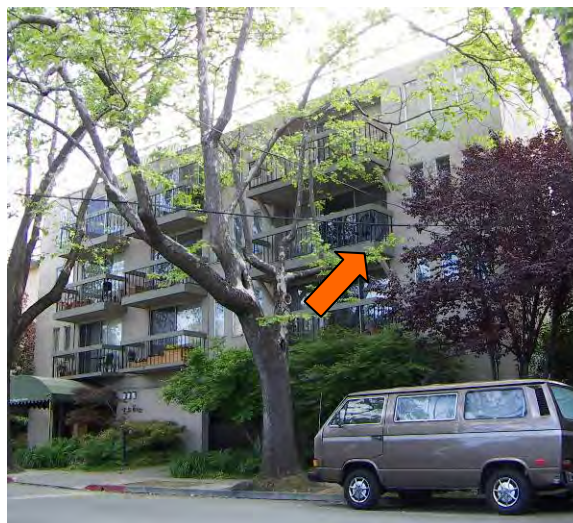
Figure 2: Street view of apartment building, indicating location
