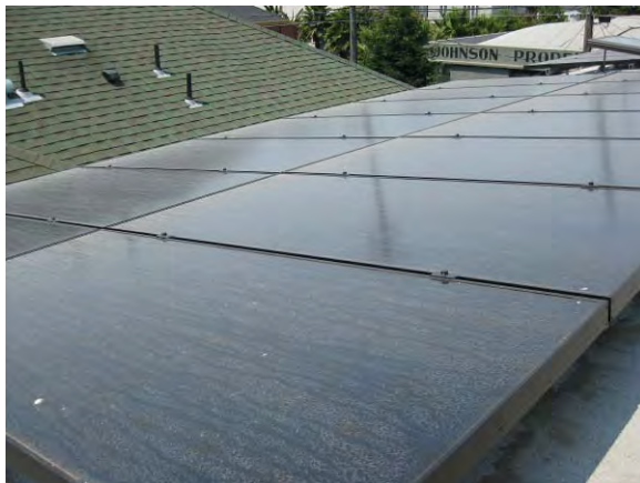
Figure 24: Photovoltaic array condition
