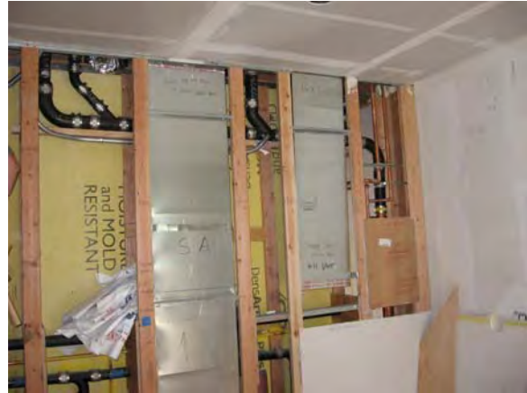
Figure 25: Mechanical core from interior side, showing uninsulated mechanical core
