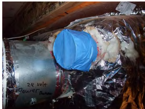
Figure 11: Removed 4" duct connection to return side of air handler (temporary seal)
