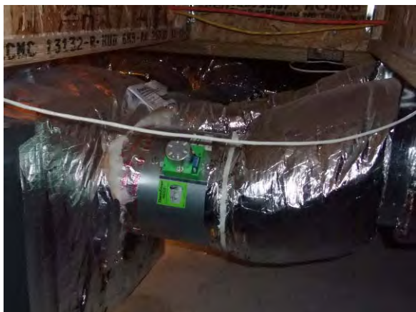
Figure 12: Motorized damper used on 10” economizer duct (DuroZone NSPRD024-10)
