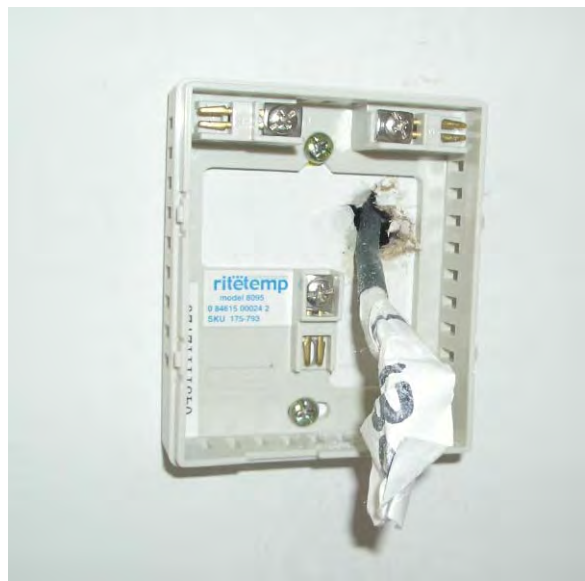
Figure 6: Fake thermostat temperature sensor
