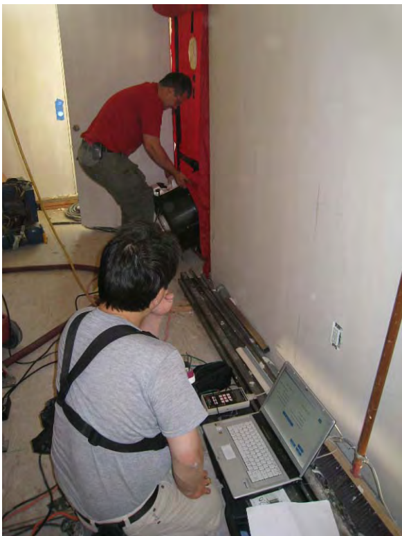
Figure 1: Blower door testing, showing installation of fan in door to garage
