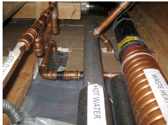
Figure 10.4.11: Tempered water output sensor (left) and incoming drain water temperature (right)
