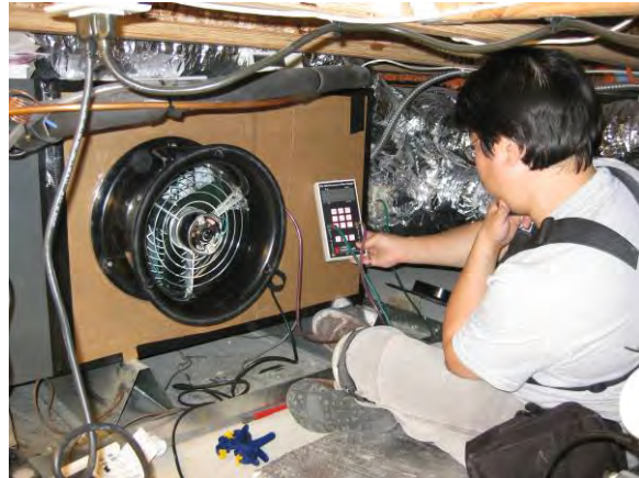
Figure 4: Testing air handler total system flow with duct blaster as metered orifice
