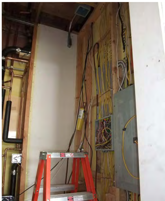
Figure 2: Mechanical room, showing open plumbing core, ceiling, and electrical panel wall
