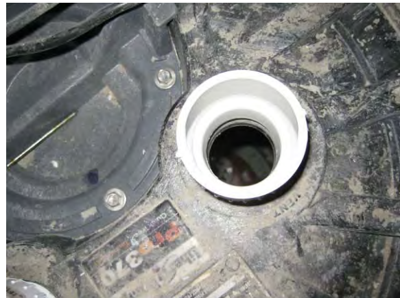
Figure 20: Open port on sump pit
