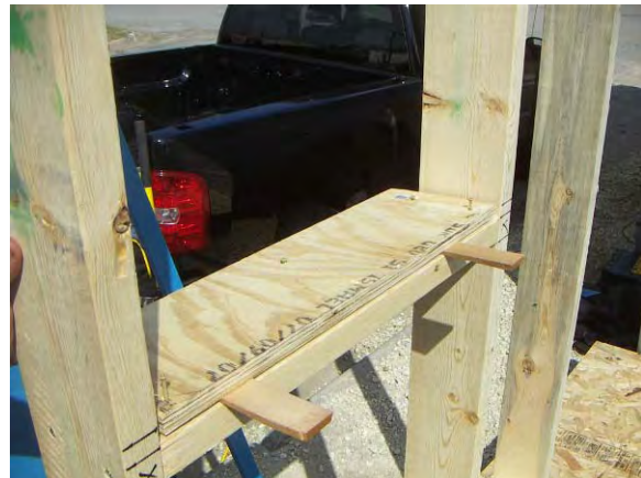
Figure 3: Rough sill extension for window dead weight (interior view)
