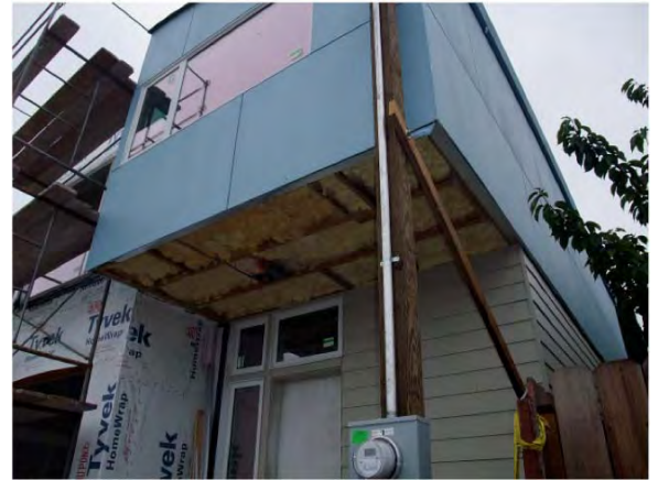
Figure 10.3.4: Spray foam installation (overhang over front porch)
