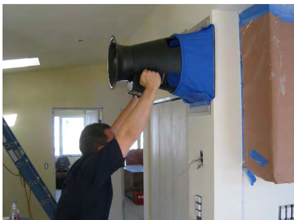
Figure 7: Measurement of registers using flow hood
