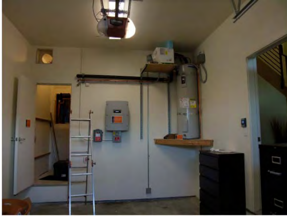
Figure 10.3.12: Water heater reinstalled in garage Figure 10.3.13: Plumbing connections
