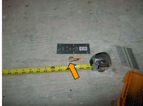
Figure 9: First floor slab temperature sensor (installed before casting slab)
