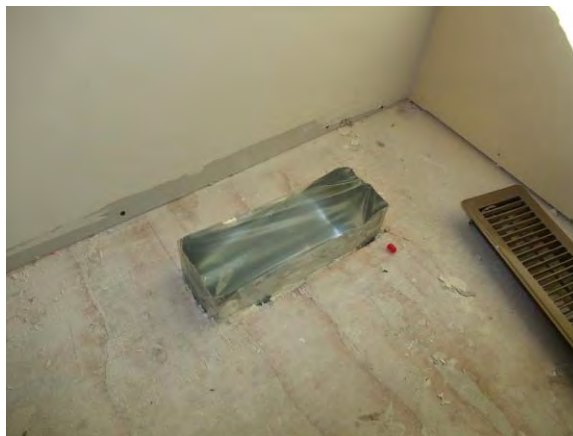
Figure 20: Sealing of registers with duct mask
