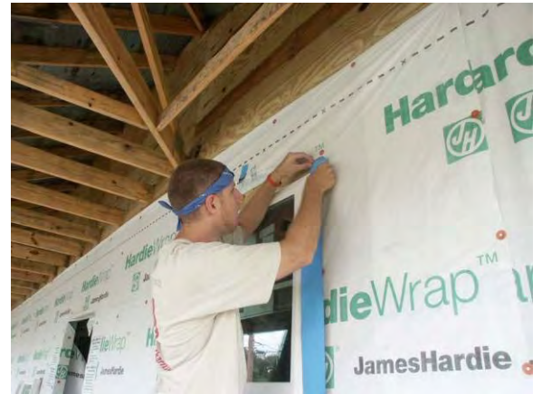
Figure 9.4.10: Installing jamb flashing
