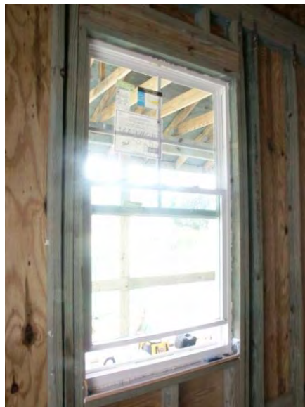
Figure 9.4.11: Installed window
