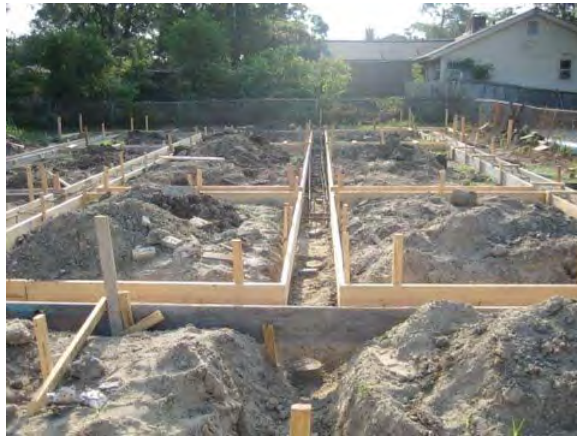
Figure 9.4.1: Wood piles and concrete grade beam formwork
