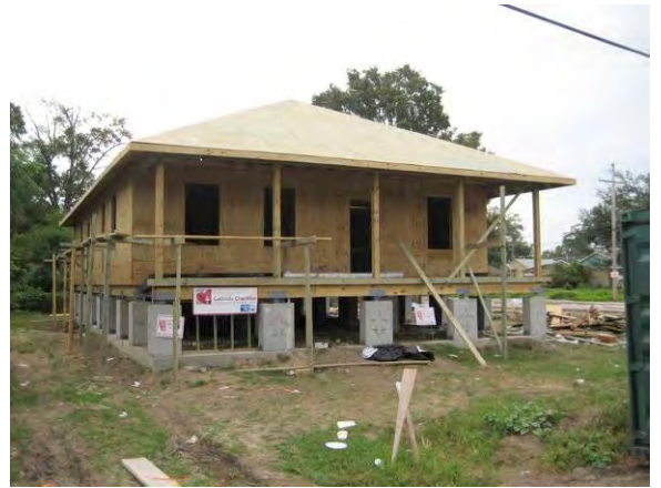
Figure 9.2.5: Treated roof sheathing
