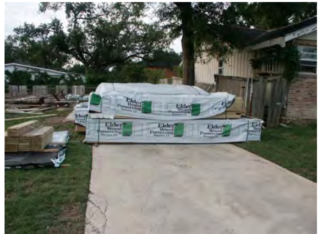
Figure 1.2 – Treated lumber arrived on site
