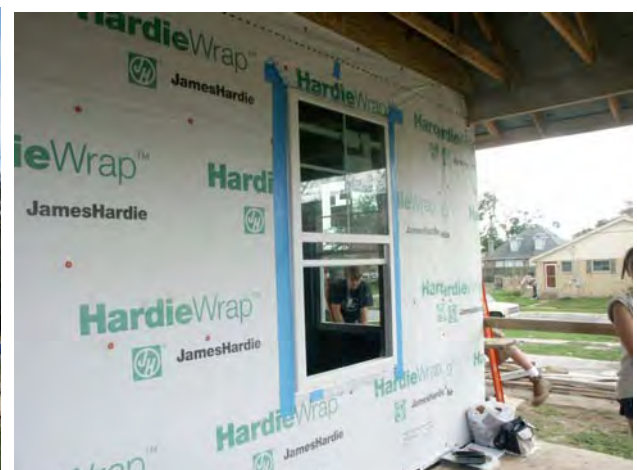
Figure 1.2 – Installed window with flashing
