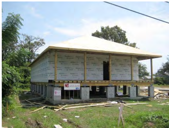
Figure 9.2.4: Roof trusses and treated wall sheathing
