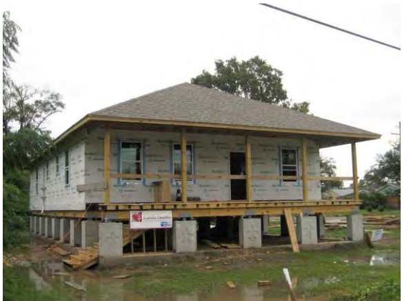
Figure 9.2.7: Roof shingles and windows
