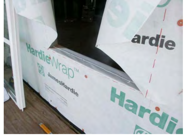
Figure 9.4.8: Cut housewrap and bead of caulk at sill
