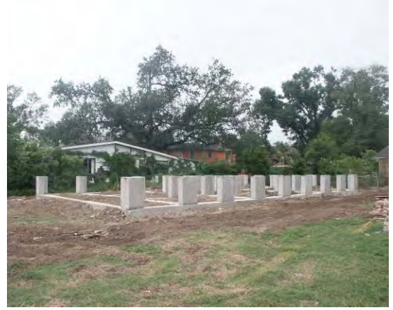
Figure 9.3.4: Concrete grade beams and piers
