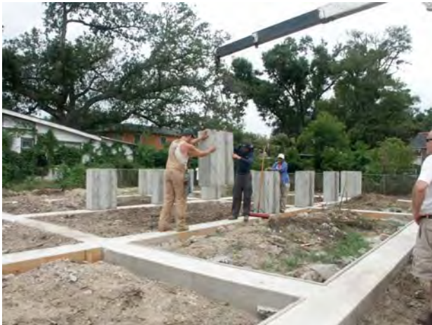
Figure 1.1 – Volunteers setting the piers
