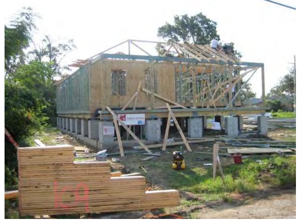
Figure 9.2.3: Roof trusses and treated wall sheathing
