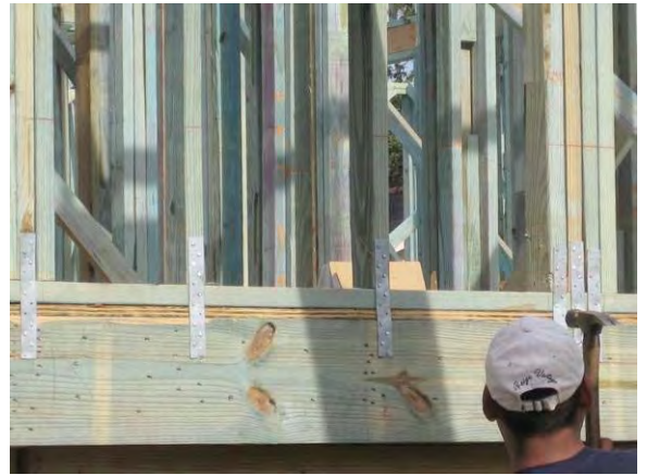
Figure 9.4.2: Wall stud to rim joist straps
