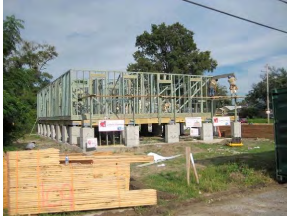
Figure 9.2.2: Concrete piers, treated floor framing and borate treated wall framing
