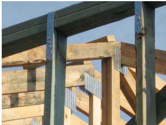
Figure 9.4.3: Top plate to wall stud straps
