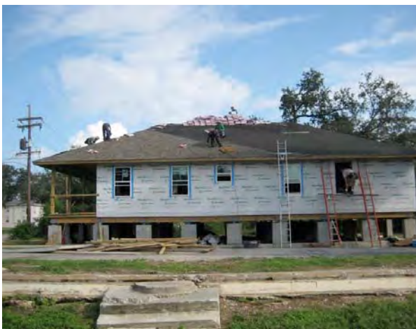
Figure 1.1 – Volunteers installing windows
