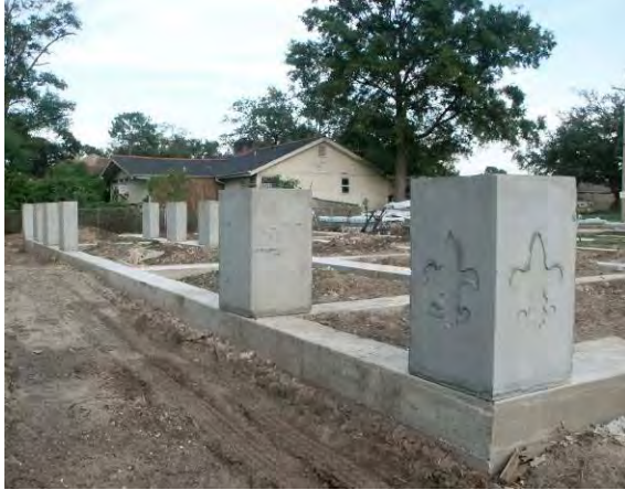
Figure 9.3.3: Concrete grade beams and piers
