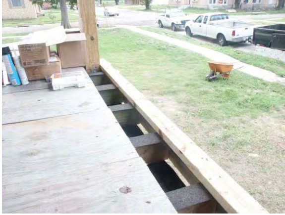
Figure 9.4.5: Self-adhered membrane on top of porch floor joists
