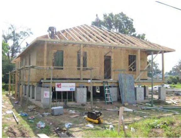
Figure 9.2.4: Roof trusses and treated wall sheathing
