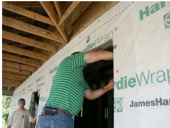
Figure 9.4.9: Folding and securing housewrap at jambs
