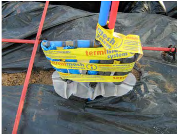
Figure 8.3-13: Termimesh® termite barrier installed at slab penetrations before slab casting
