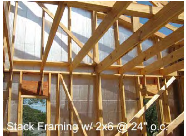
Figure 8.3-8: Stacked framing
