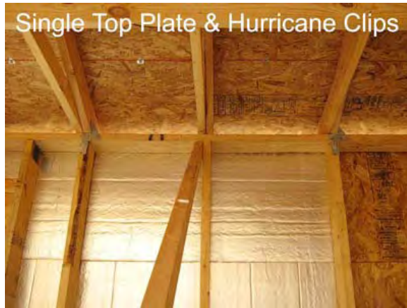
Figure 8.3-7: Advanced framed walls – 2x6 studs at 24" o.c.
