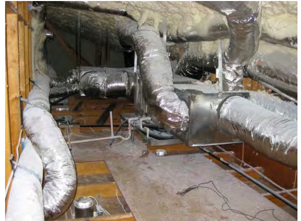
Figure 8.3-4: Open cell low density spray foam unvented cathedralized attic with the HVAC system
