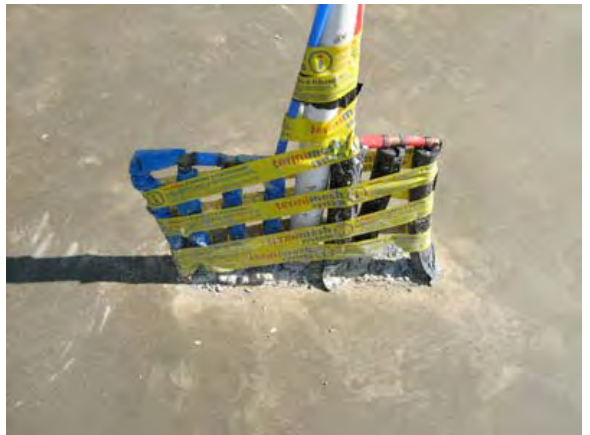
Figure 8.3-14: Slab penetrations after slab casting
