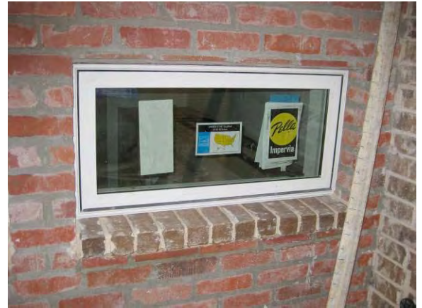
Figure 8.3-12: Window with brick cladding installed
