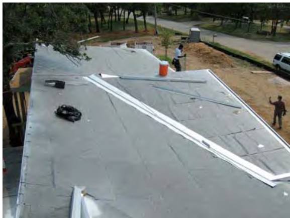
Figure 8.3-5: Fully adhered roofing membrane installed before standing seam roof
