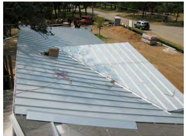
Figure 8.3-6: Standing seam metal roof
