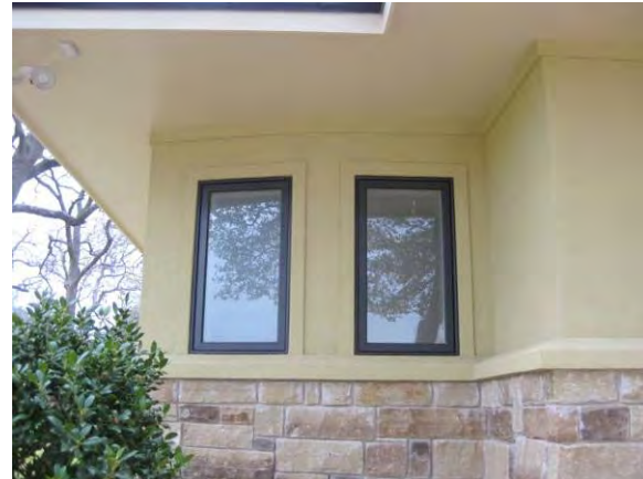
Figure 7.3-12: Window with cladding installed
