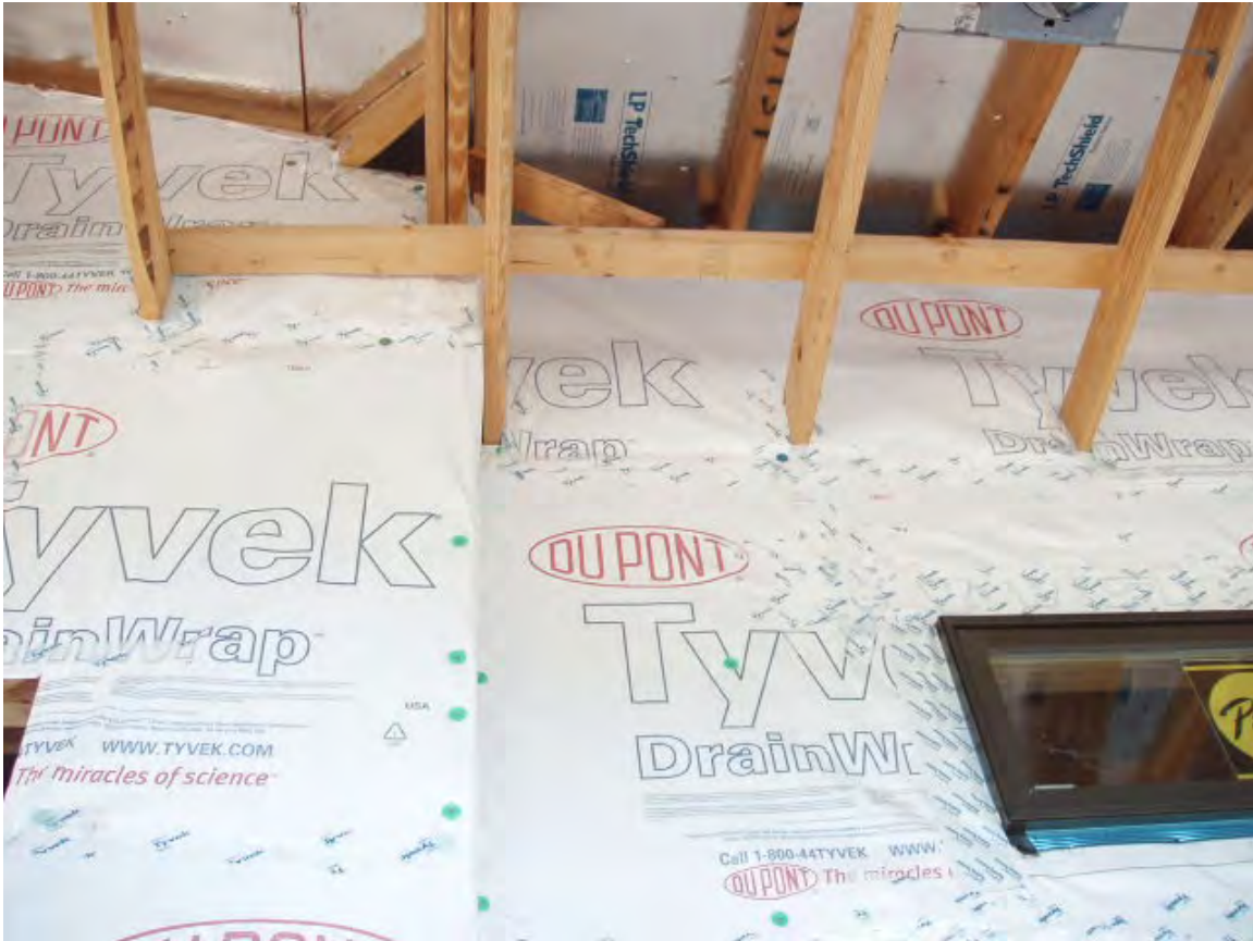
Figure 2: Walls wrapped with Tyvek® DrainWrap™
