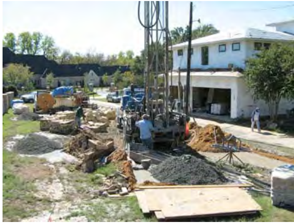
Figure 7.3-17: Well drilling
