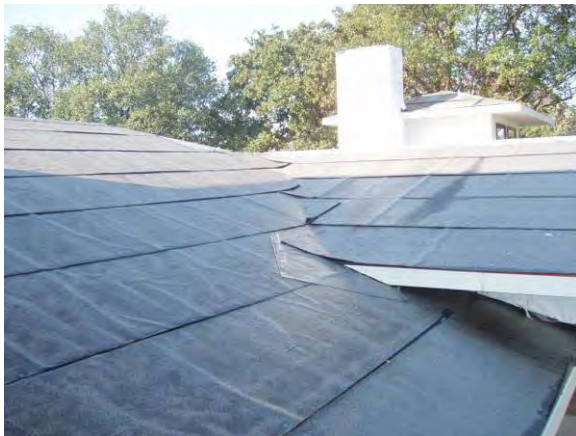
Figure 7.3-5: Fully adhered roofing membrane installed before standing seam roof
