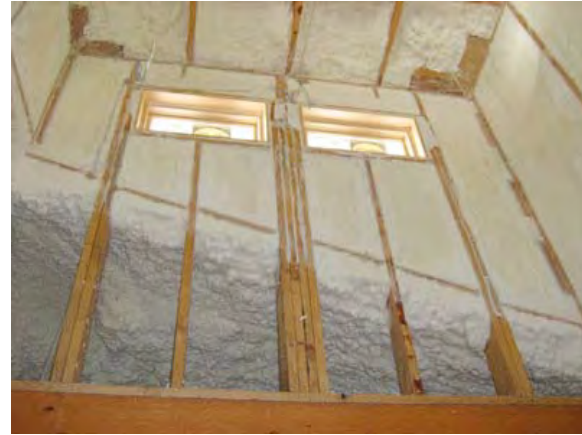
Figure 7.3-16: Low density open cell spray foam in attic knee walls
