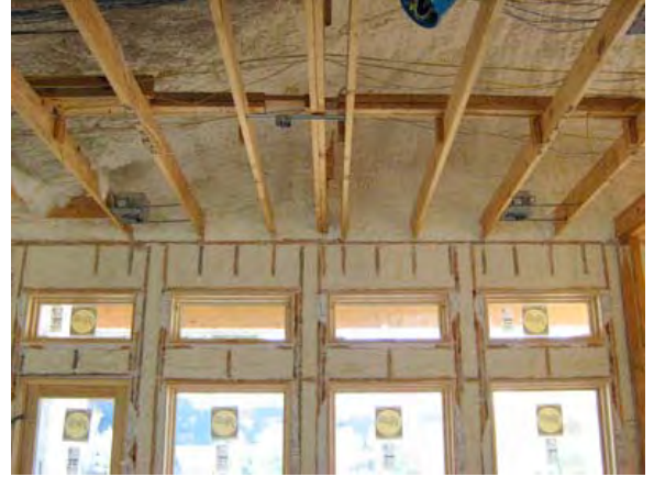
Figure 7.3-4: Open cell low density spray foam in walls and unvented cathedralized attic
