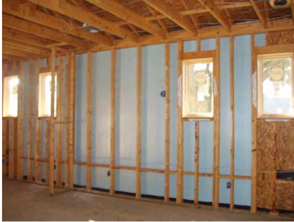
Figure 7.3-7: Advanced framed walls – 2x6 studs at 24” o.c.
