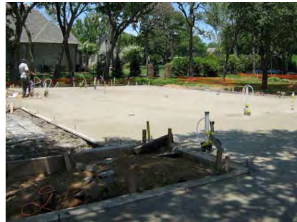
Figure 7.3-14: 51% Fly Ash post tensioned slab on grade
