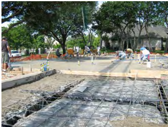
Figure 7.3-13: Slab reinforcement before casting
