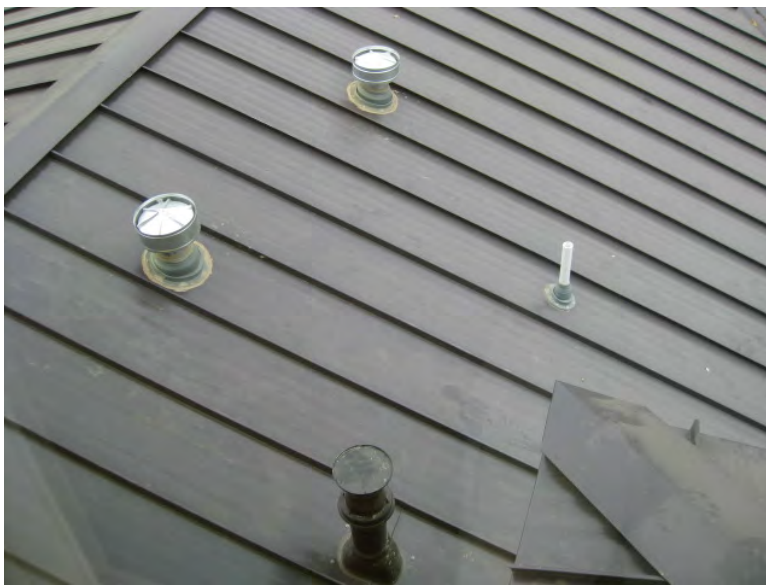
Figure 4: Standing seam metal roof
