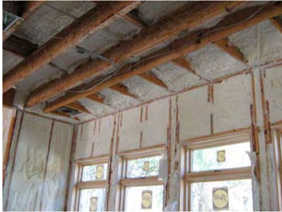
Figure 7.3-15: Low density open cell spray foam in unvented cathedralized attic (R-30) and walls (R-20)
