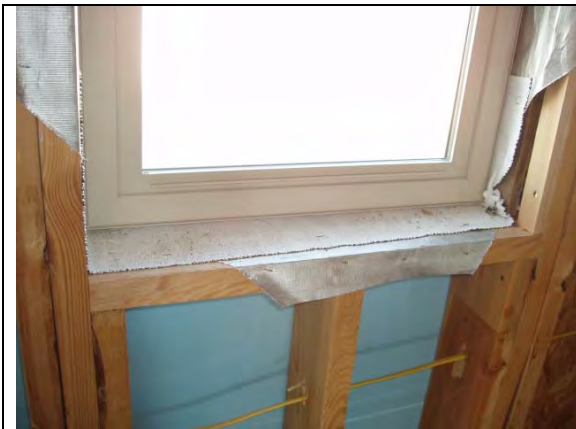
Window framing with FlexWrap
