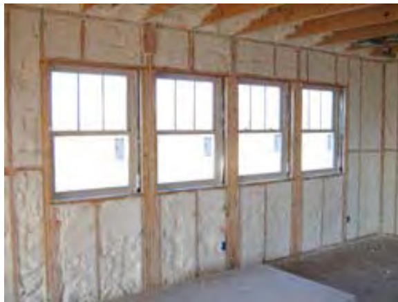
Figure 6.3.17: Wall cavities insulated
