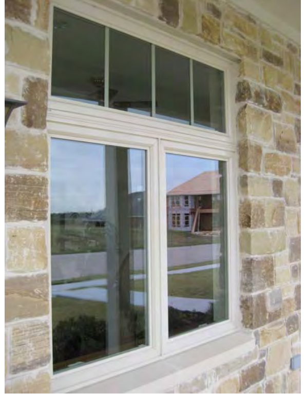
Figure 6.3.16: Vinyl windows with stone cladding installed
