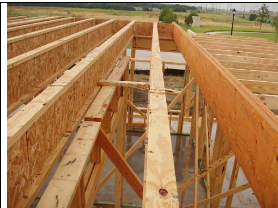
16" TJI floor joists stack framed over first floor studs
