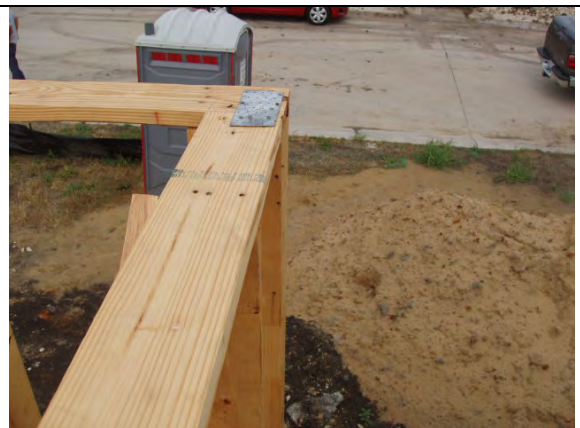
Connector plate at corner framing
