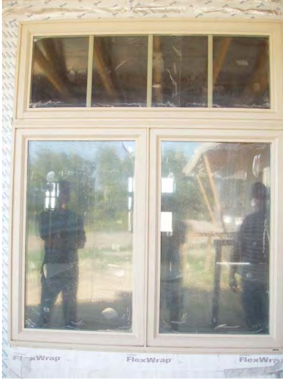
Figure 6.3.15: Vinyl framed windows before cladding installation
