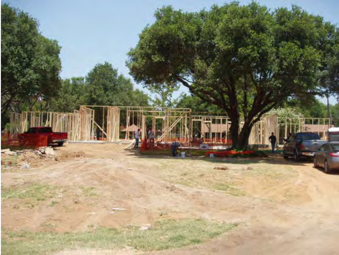
Figure 2: 2009 Colleyville House framing
