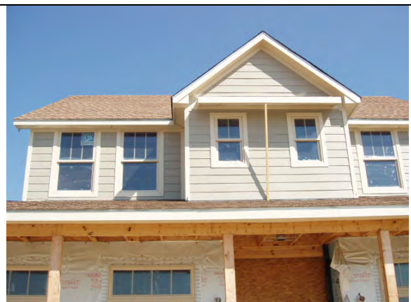
Second Floor Hardie Board is installed.
