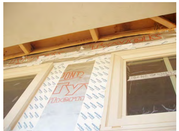
Figure 6.3.14: StraightFlash™ installed on the jambs and at the head of the rough opening
