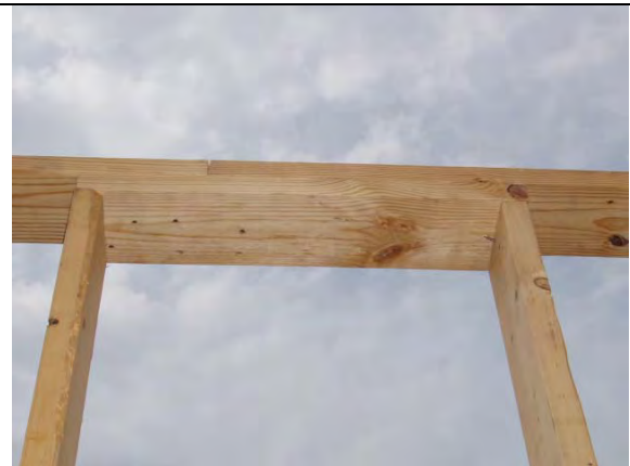
Stud used as a splice connector in between studs
