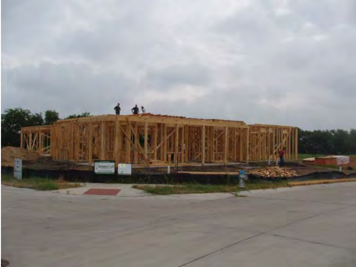
Figure 1: Prosper House first floor framing
