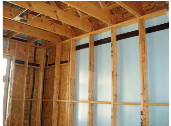
Figure 6.3.11: Another method of joining the single top plates together: line the joint on top of an existing stud
