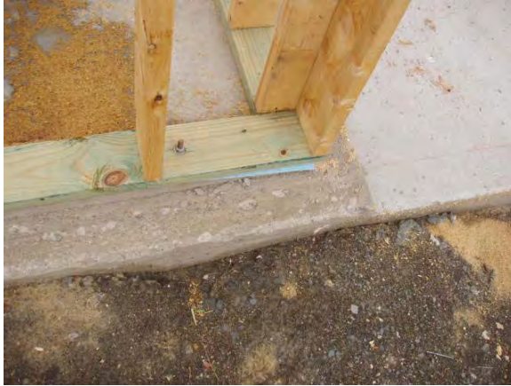
Figure 6.3.4: Two stud “energy corner”
