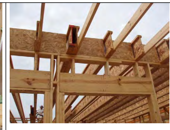
Header hangers were considered but Greencraft decided to frame with jack studs.
