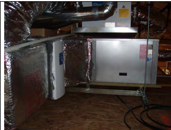
Horizontal air handler (with large pleated filter) with GeneralAire Model 1300 dehumidifier (on top)
