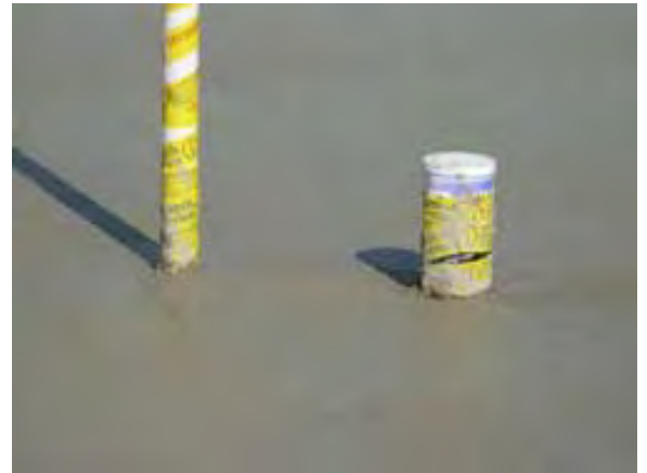
Figure 6.3.3: Penetrations after slab casting
