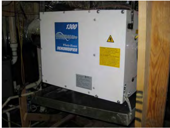
Figure 6.3.26: GeneralAire® Model 1300 whole house dehumidifier
