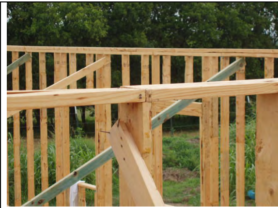
Top plate splice positioned on stud
