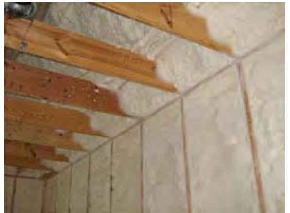
Figure 6.3.18: Insulation continues up the rim joist and under the roof sheathing
