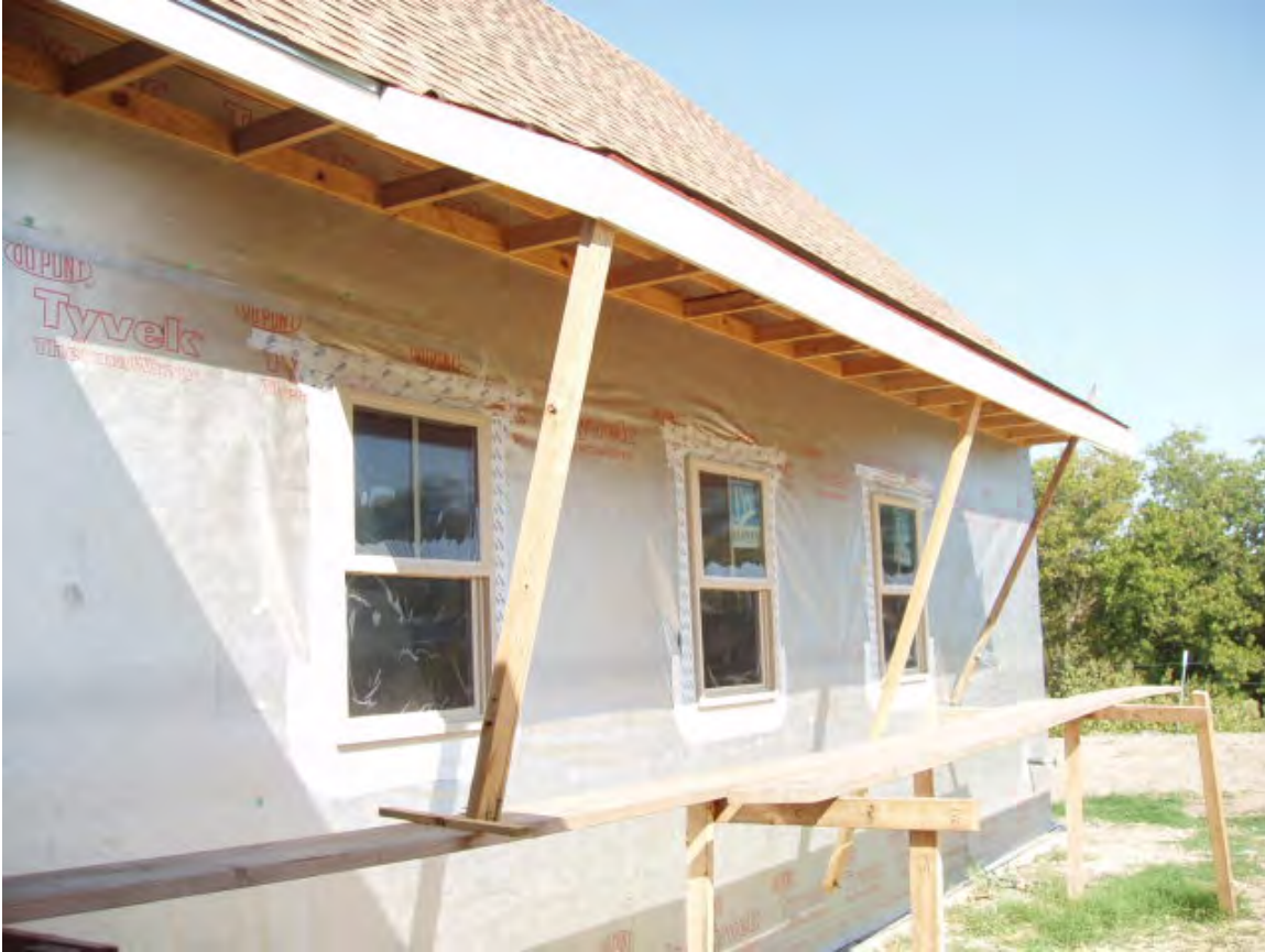
Figure 2: Walls wrapped with Tyvek® ThermaWrap™
