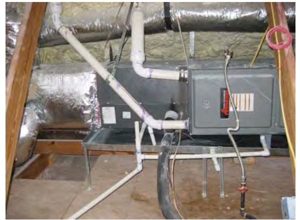
Figure 6.3.24: Unit 2 (2-ton) for the second floor
