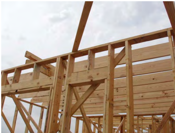
Figure 6.3.6: Single top plate
