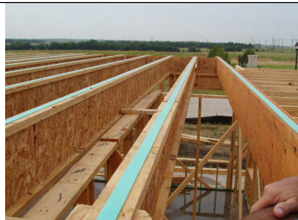
TJIs with sound isolation tape
