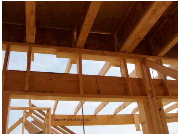
Figure 6.3.10: Stack framing of the floor joists on the
