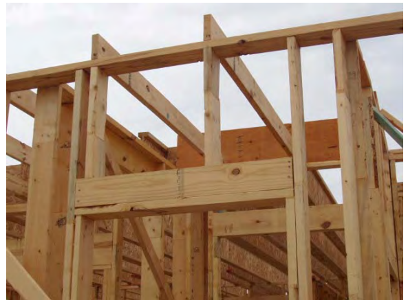
Figure 6.3.7: Another view of the single top plate
