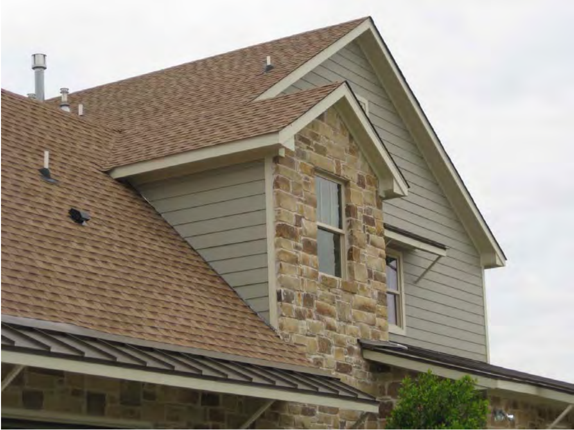
Figure 4: Composition Shingles metal roof
