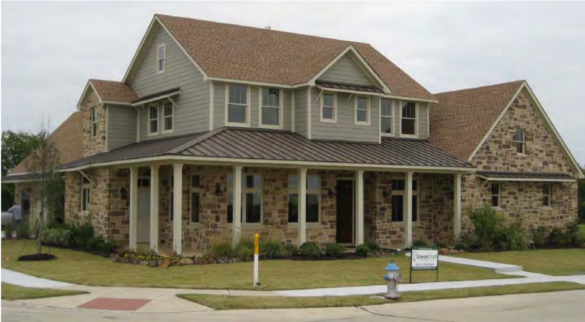
Figure 1: Greencraft Prosper House at 2481 Stonybrook Dr, Prosper, TX
