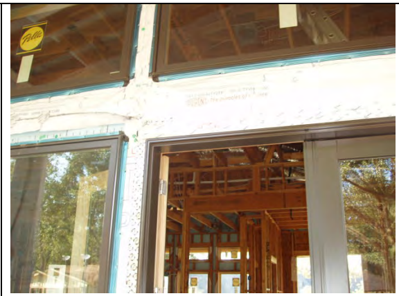
Pella® Windows installed with proper flashing
