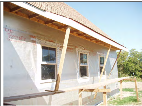
Tyvek® ThermaWrap™ installed on first floor before cultured stone
