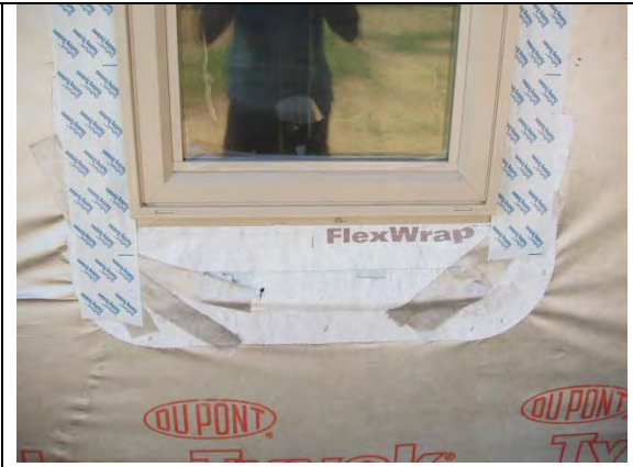
Double flashed sill flashing with FlexWrap
