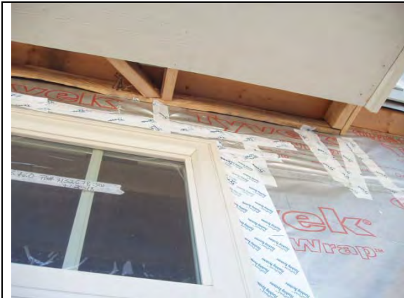
Header flashing piece added
