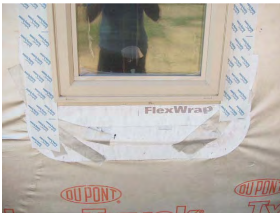
Figure 6.3.13: FlexWrap™ installed at the window sill
