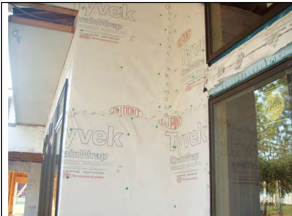
Tyvek® DrainWrap™ cap nailed and taped
