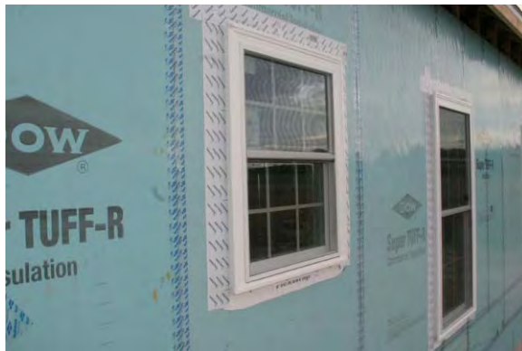
Figure 5.3.3: Taped connections at jambs, head, and joints in foam
