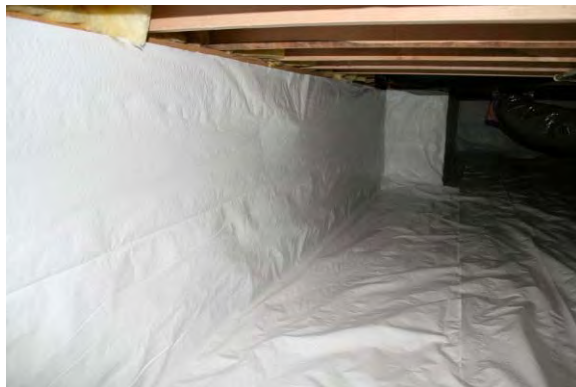
Figure 5.5.2: Groundsheet lines interior of crawlspace
