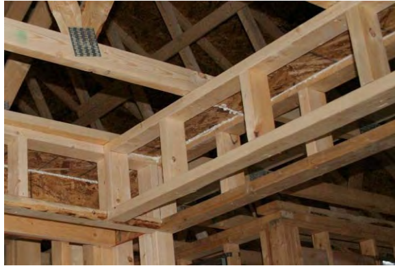
Figure 5.3.5: Blocking in ceiling assures airtightness
