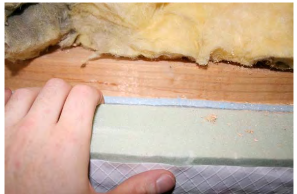
Figure 5.5.3: Air gap behind foam and groundsheet
