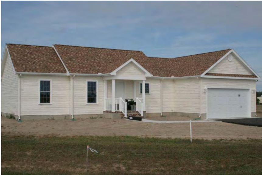
Figure 5.2.1: Front entrance (South) of Allen home before testing
