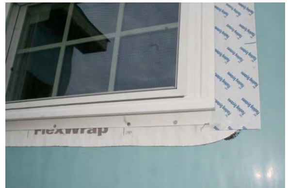
Figure 5.3.4: Membrane flashing at window sill
