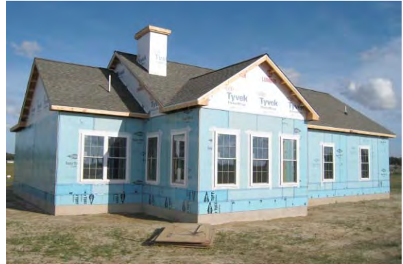
Figure 5.2.3: Alexander house plan during construction
