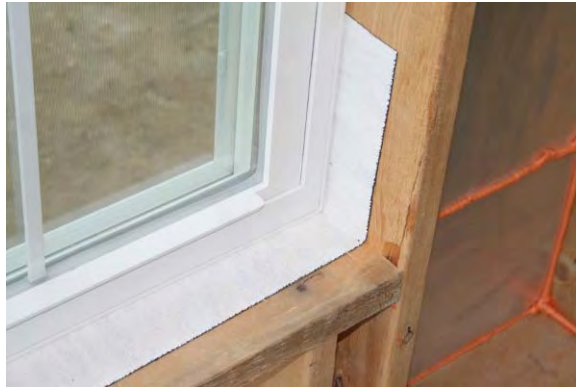
Figure 5.5.4: Installed window with flexible membrane
