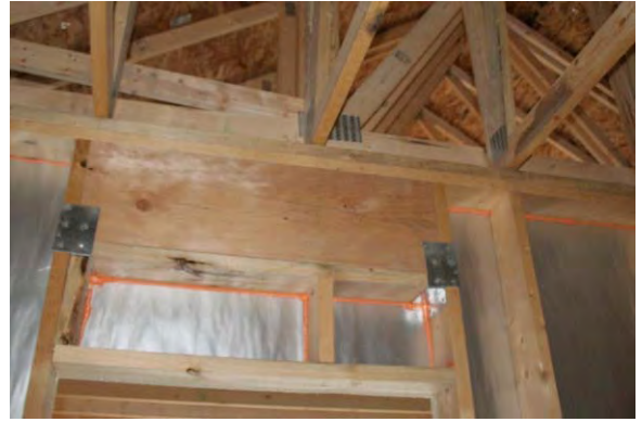
Figure 5.3.6: Spray foam connects sheathing to framing
