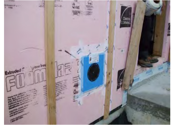
Figure 4.4.3: Pre-manufactured mechanical penetration flashing
