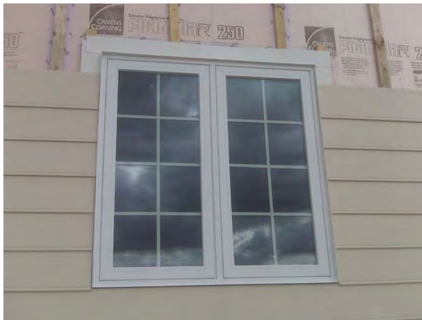
Figure 4.4.4: Custom metal channel at window perimeter
