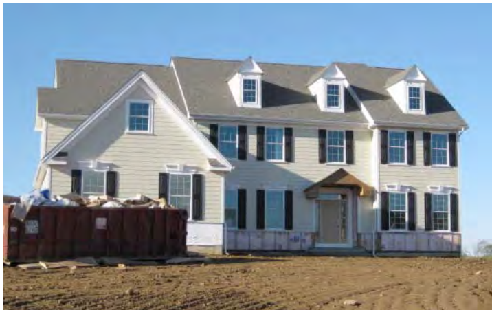
Figure 4.2.1: House near completion
