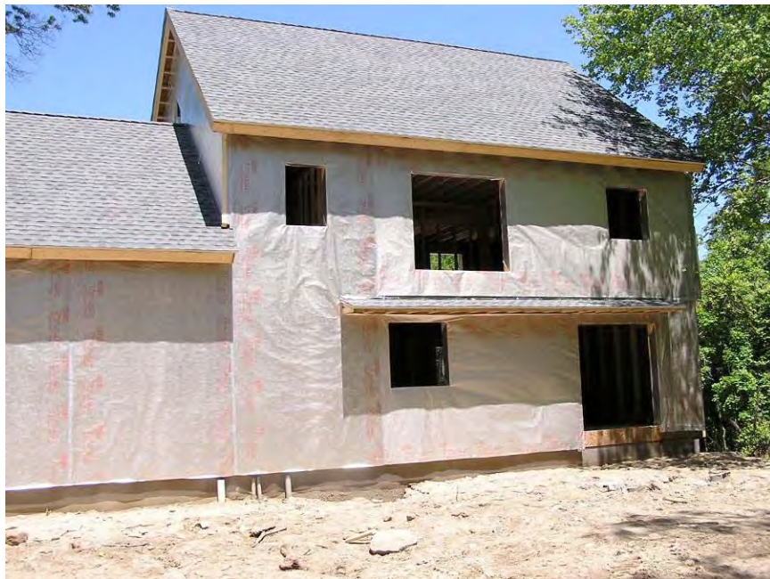
Figure 3.2: Roof overhang provides partial shading for glazing on South elevation
