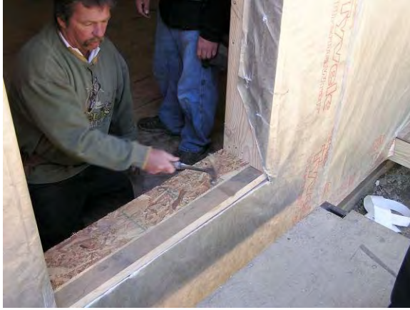
Figure 3.13: Framer installing back dam material before application of sill pan flashing
