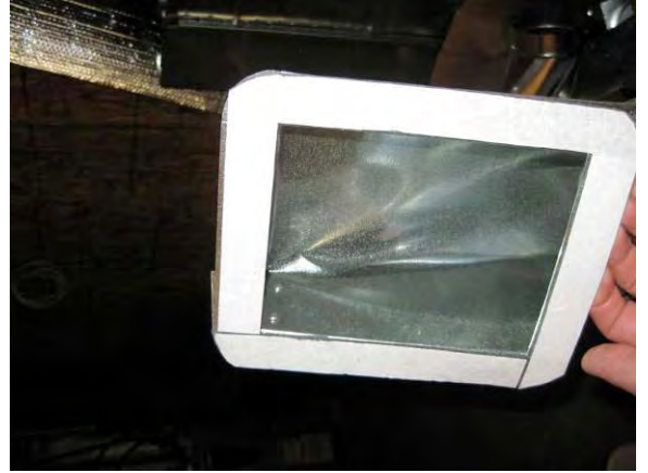
Figure 3.16: Gasketed register boot
