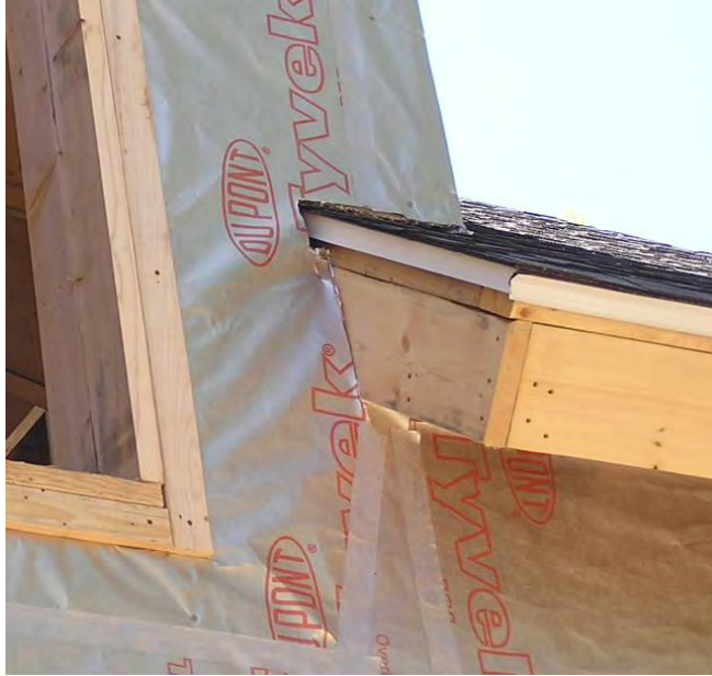
Figure 1 - Roof Rake Return
