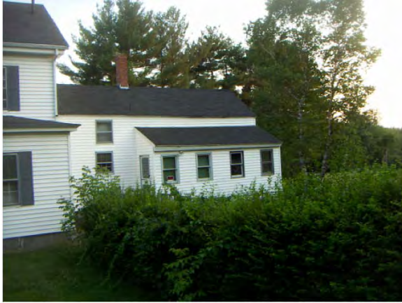
Figure 2.3: Existing rear addition
