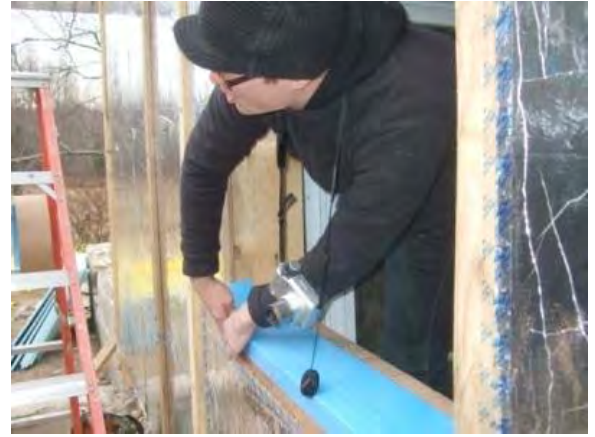
Figure 2.33: BSC engineer demonstrating window flashing
