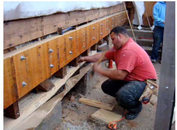
Figure 2.23: Toenailing of existing studs to replacement beam
