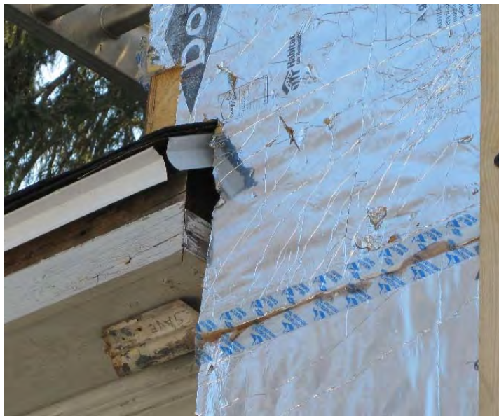
Figure 2 - Front entry porch roof at corner
