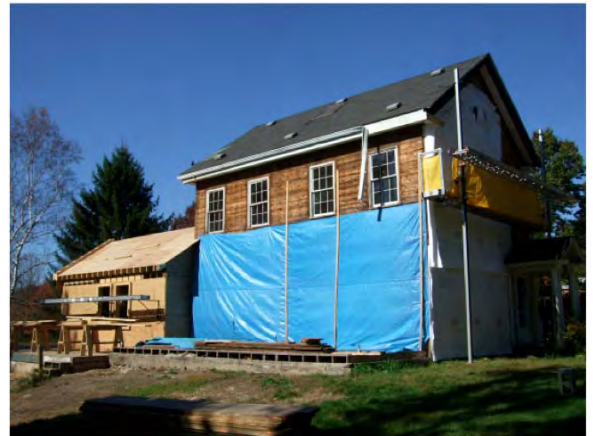
Figure 2.2: South elevation showing demolition and new rear addition
