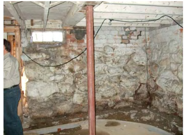
Figure 2.6: Existing rubble stone foundation
