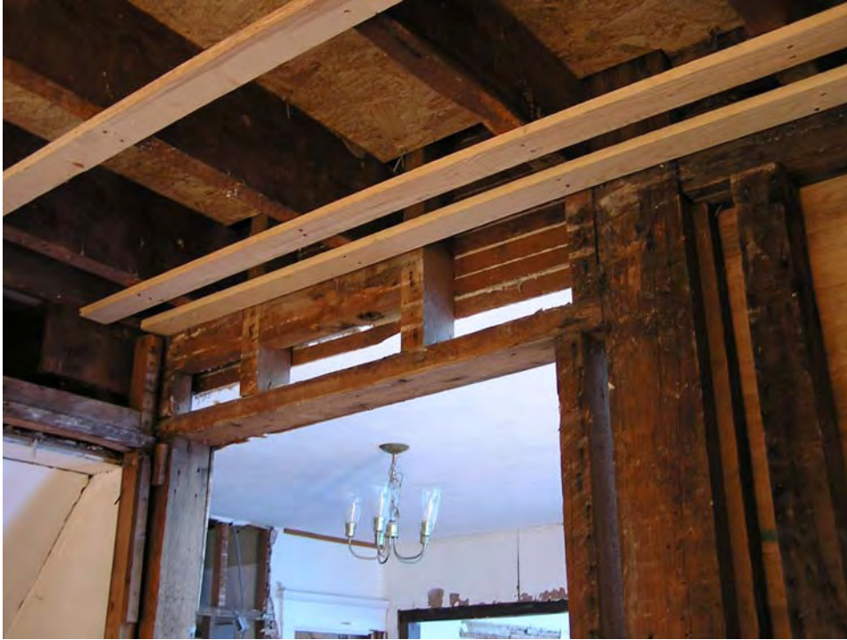
Figure 1: Opening to addition_1.JPG
