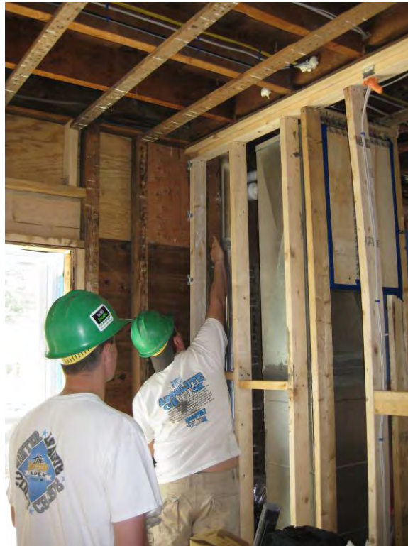
Figure 21 - Habitat volunteers locating and sealing duct leaks
