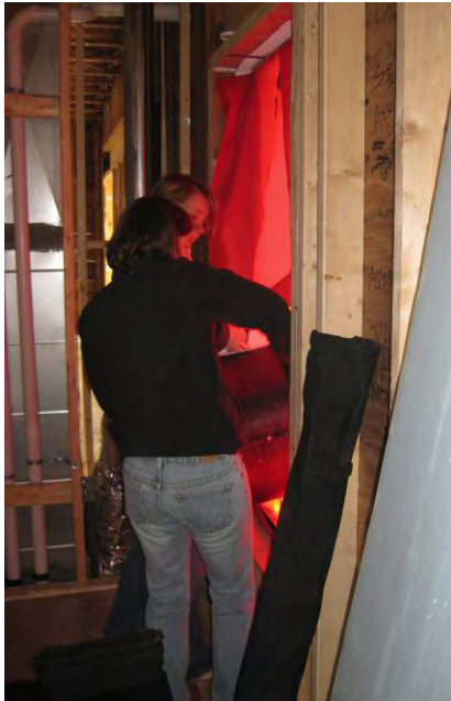
Figure 6 - blower door installation
