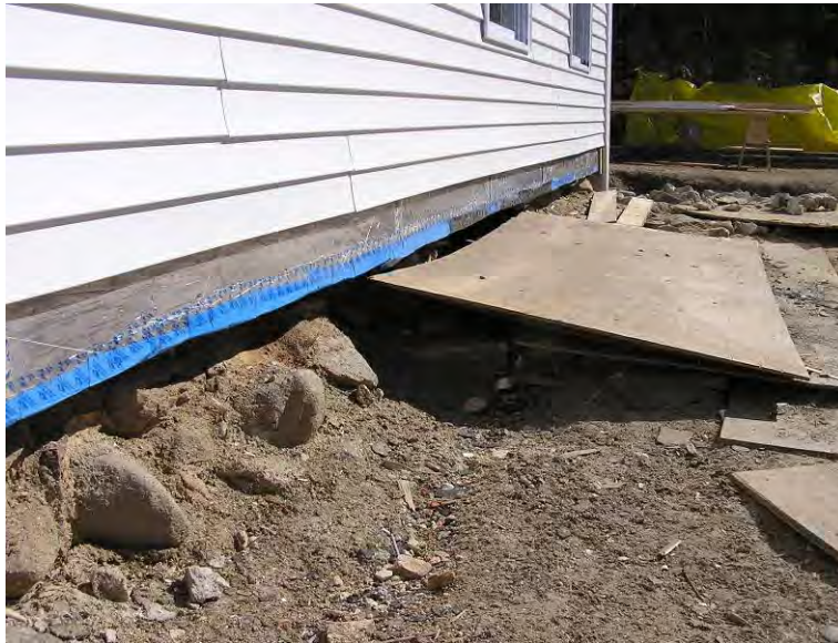
Figure 13 - sill to wall air barrier transition
