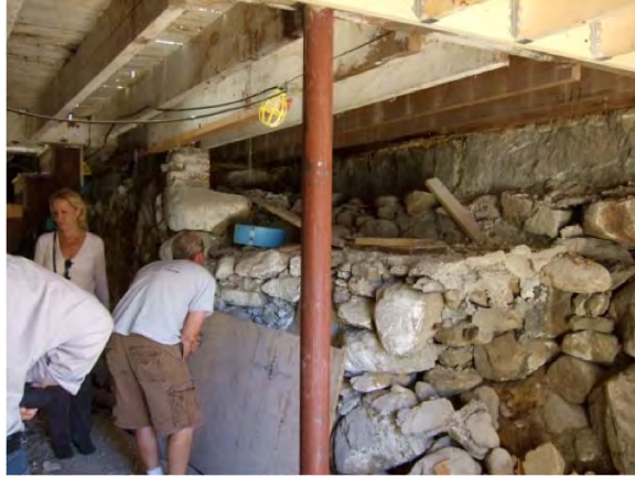
Figure 2.17: Evaluation of foundation risks
