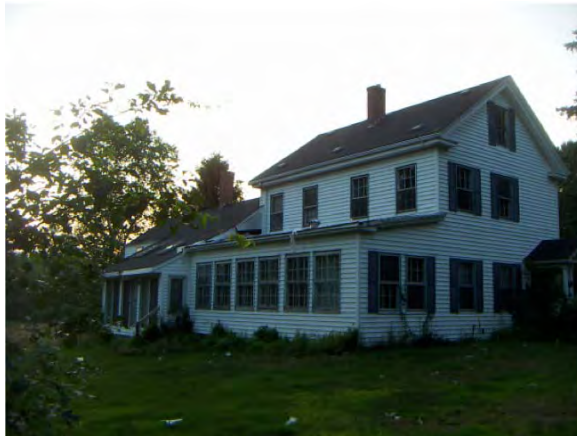
Figure 2.1: South elevation showing added sunroom and rear addition demolished prior to retrofit
