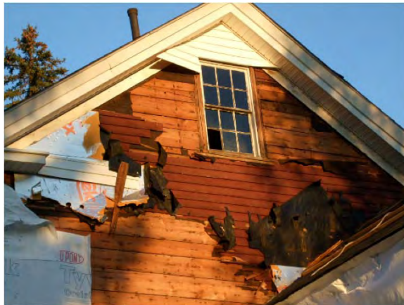
Figure 2.5: Demolition photo showing multiple layers of exterior wall cladding
