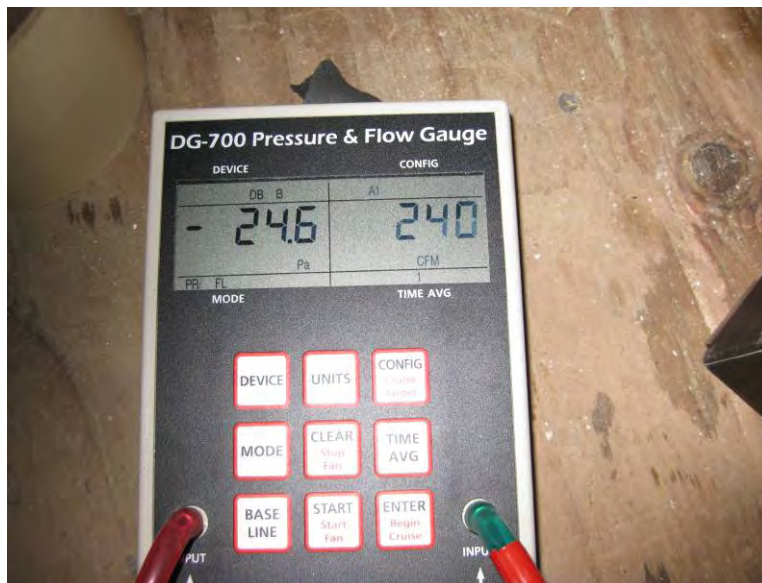
Figure 22 - duct leakage test results after duct sealing
