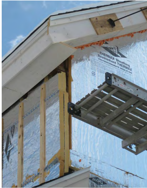
Figure 3 - Foam Sheathing Corner
