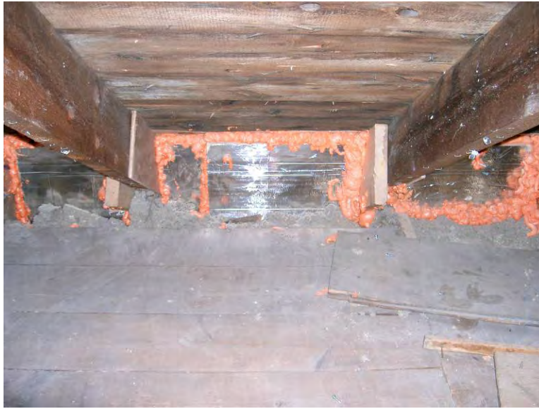
Figure 2 - air sealing at existing roof eave
