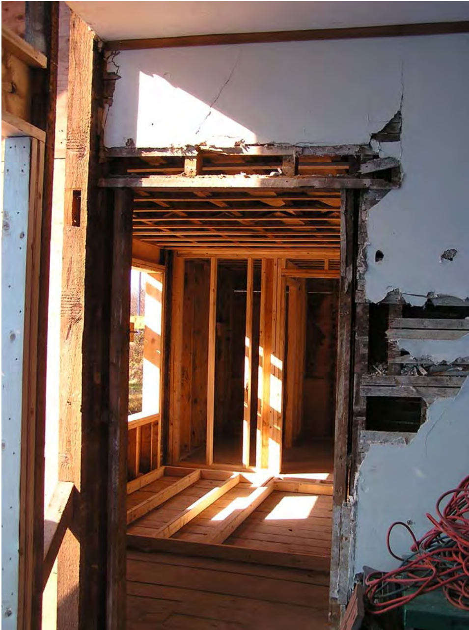
Figure 3: Opening to addition_3.JPG
