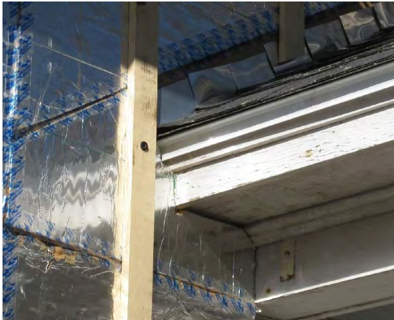
Figure 3 – Roof over front entry at front wall
