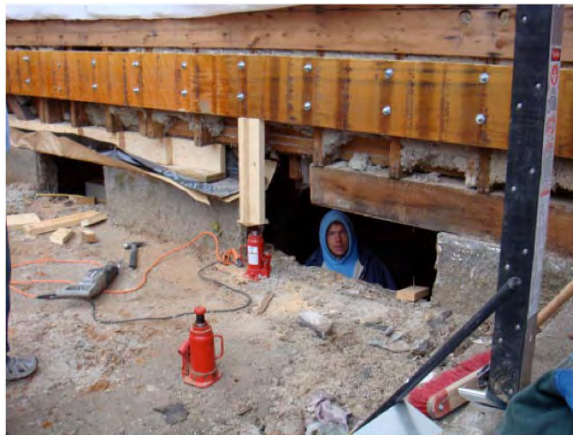
Figure 2.22: LVL used as lifting beam for sill replacement
