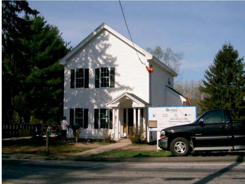
Figure 2.7: Bedford Farmhouse Retrofit nearing completion
