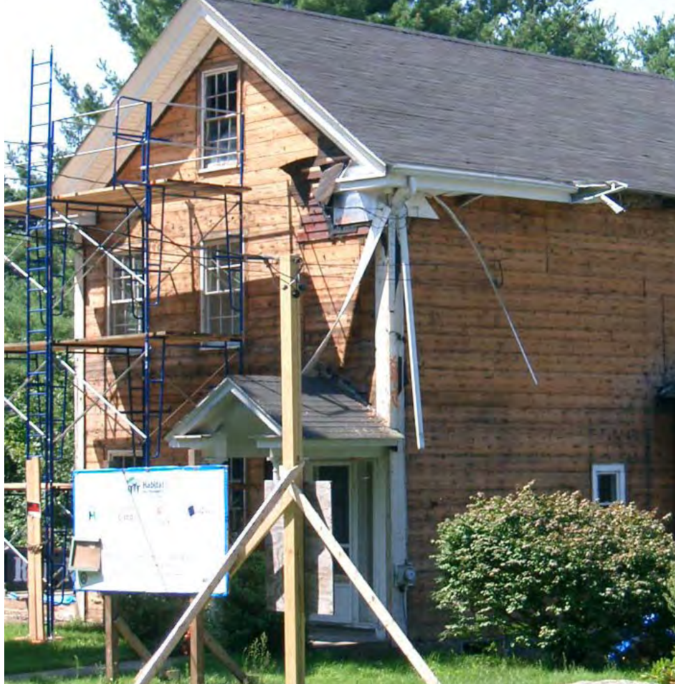
Figure 1 - Earlier trim details revealed during demolition
