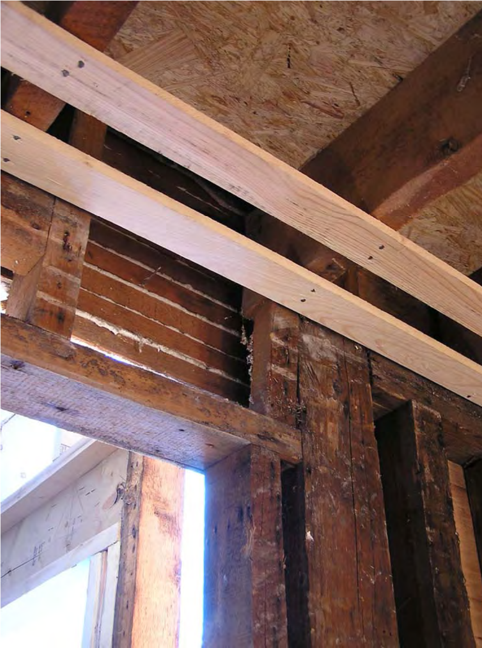
Figure 2: Opening to addition_2.JPG
