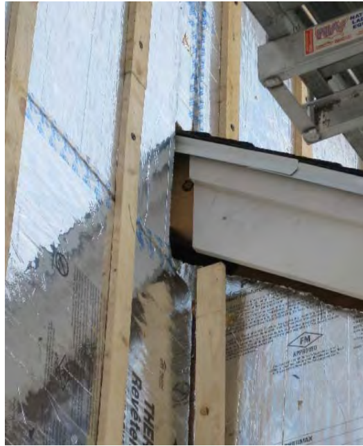
Figure 1 - Kitchen Roof Rake at Adjoining Wall
