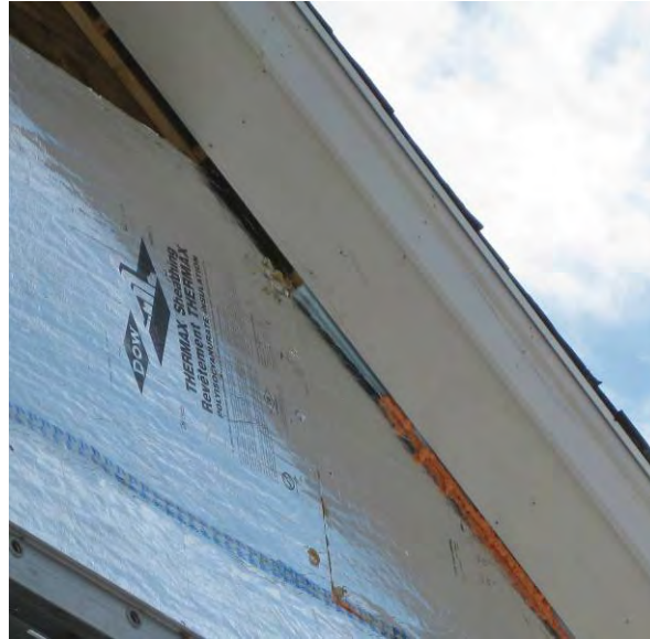
Figure 12 - insulating sheathing at West gable
