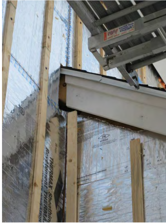
Figure 4 - Wall to Roof Connection
