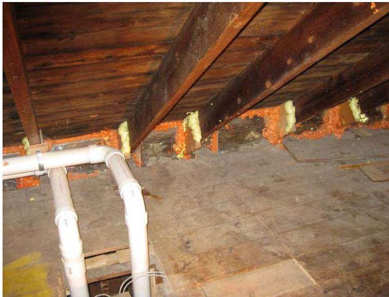
Figure 9 - additional air sealing at existing roof eaves
