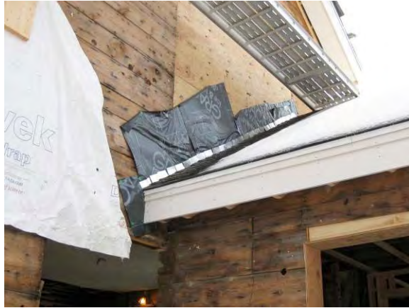
Figure 2.28: Step flashing applied behind intended location of drainage plane
