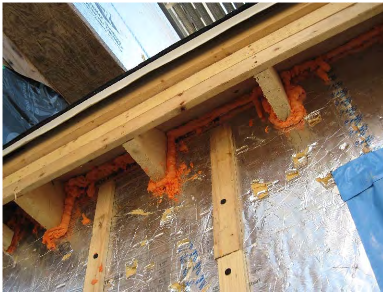
Figure 1 - air sealing at addition roof eave
