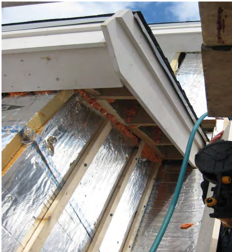
Figure 11 - addition roof rake during construction prior to air sealing remediation
