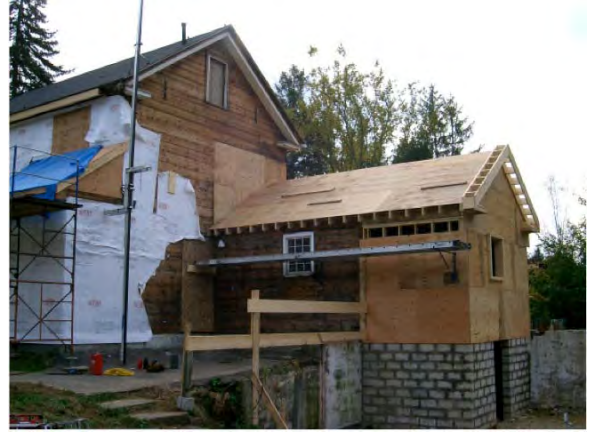
Figure 2.4: Rebuilt rear addition
