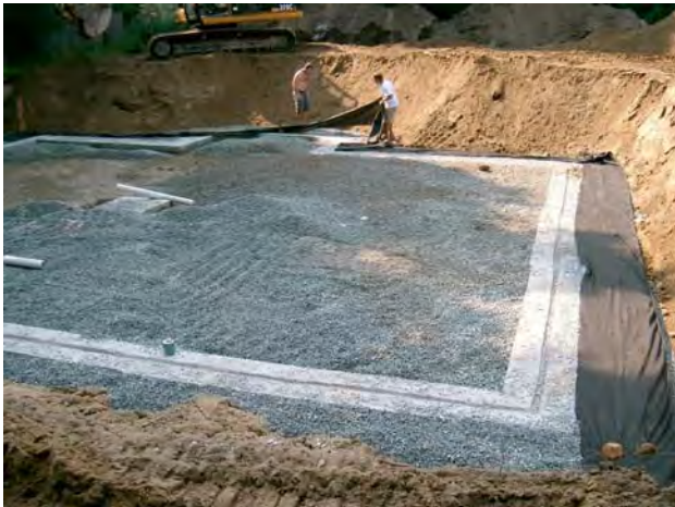
Figure 1.1 – Installing filter fabric
