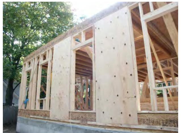
Figure 1.2 – OSB sheathing
