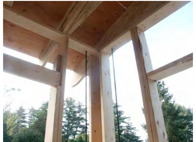
Figure 1.2 – Threaded rod tie-downs
