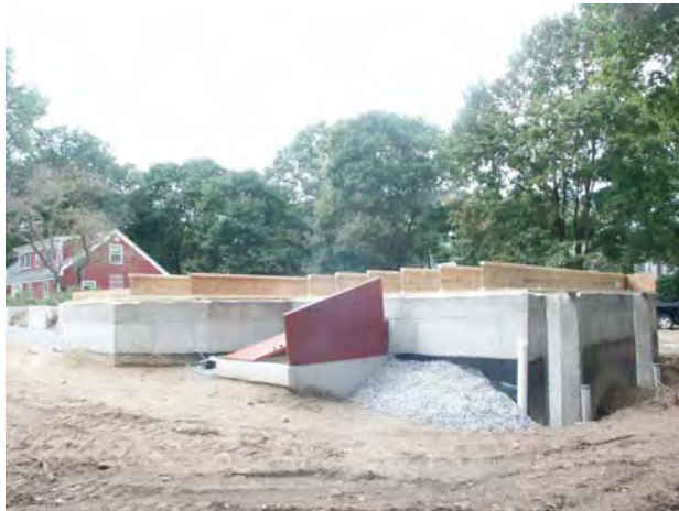
Figure 1.1 – Framing as seen from back of house
