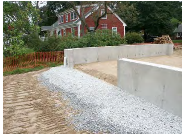
Figure 1.2 – Gravel above backfill at garage
