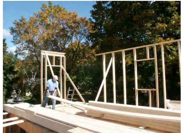
Figure 1.2 – Second floor walls and dormer wall
