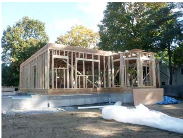
Figure 1.1 – Framing from back of house
