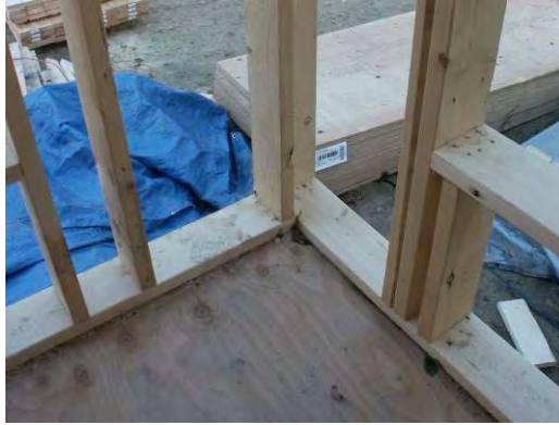
Figure 1.4.5: Two stud corner
