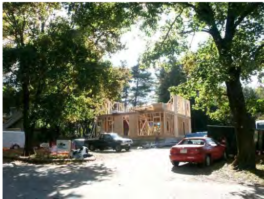
Figure 1.2.6: Second floor wall framing
