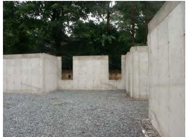
Figure 1.2 – Inside view of foundation walls
