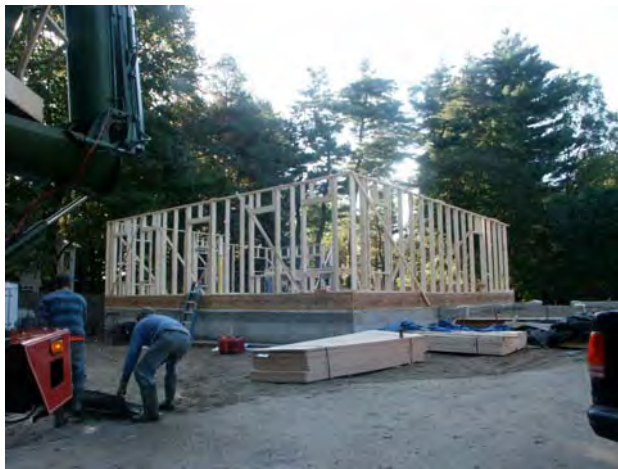
Figure 1.1 – First floor wall framing
