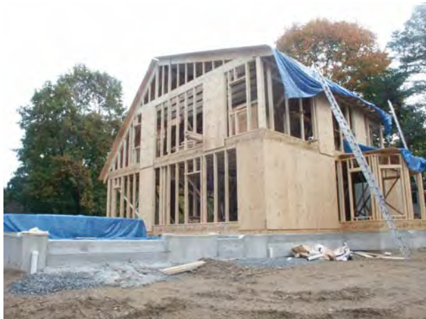
Figure 1.1 – Framing from back of house
