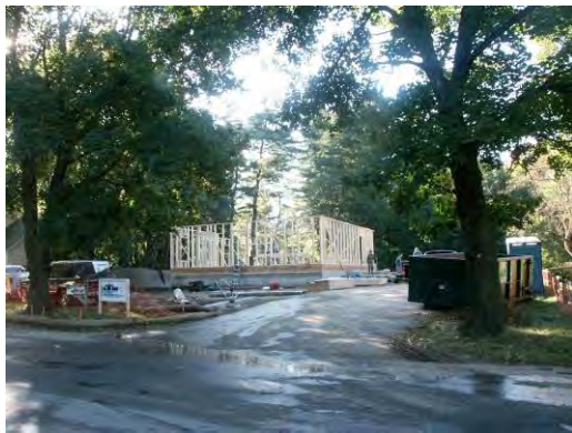
Figure 1.2.4: First floor wall framing
