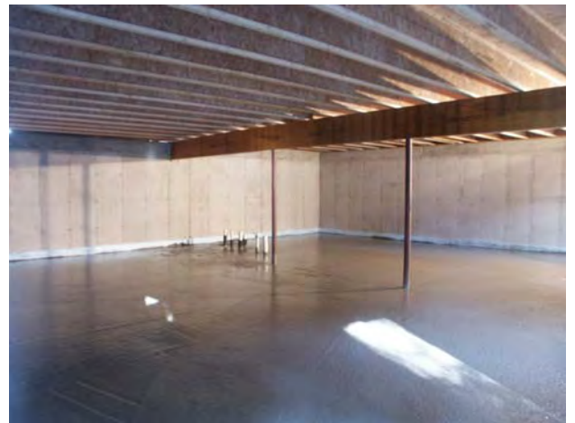
Figure 1.2 – Basement slab and perimeter foam
