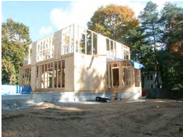
Figure 1.1 – Framing from back of house
