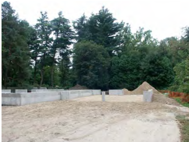
Figure 1.1 – House and garage foundation walls
