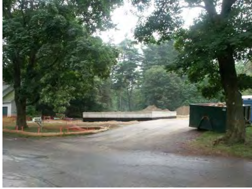
Figure 1.2.2: Main house foundation and applied damproofing
