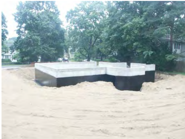
Figure 1.1 – Foundation walls with dampproofing
