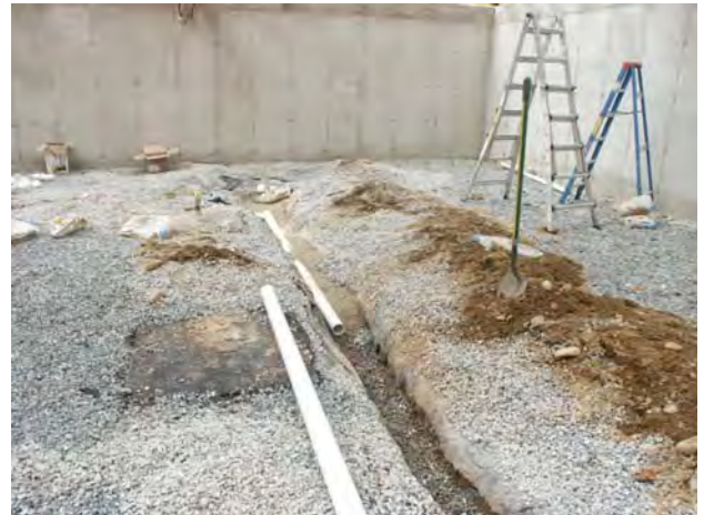
Figure 1.2 – Trench dug for basement plumbing
