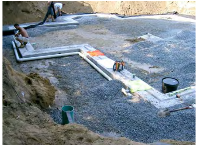
Figure 1.2 – Installing perimeter drain
