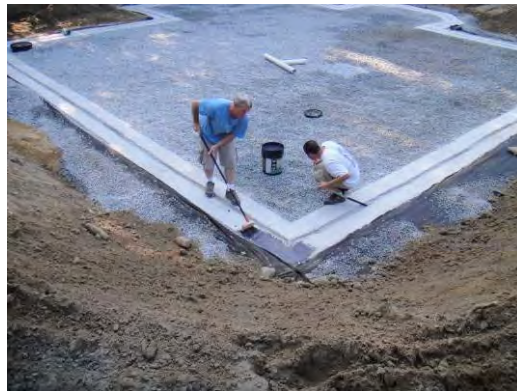
Figure 1.4.1: Applying capillary break on top of footings
