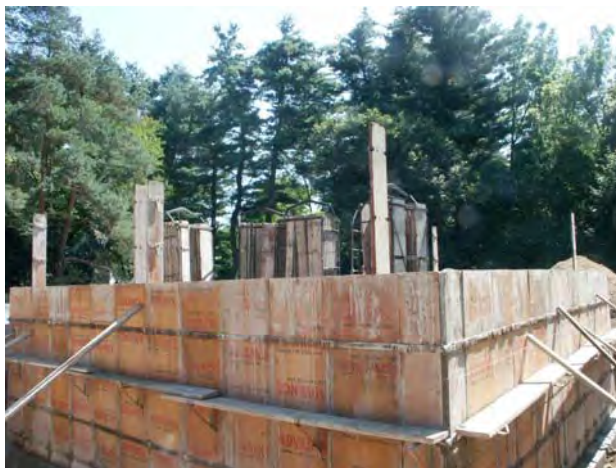
Figure 1.1 – Garage foundation wall formwork
