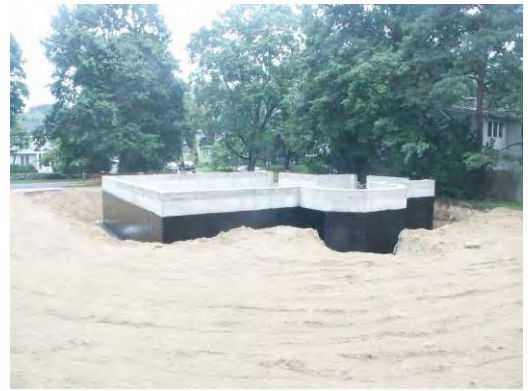
Figure 1.4.2: Foundation wall damproofing
