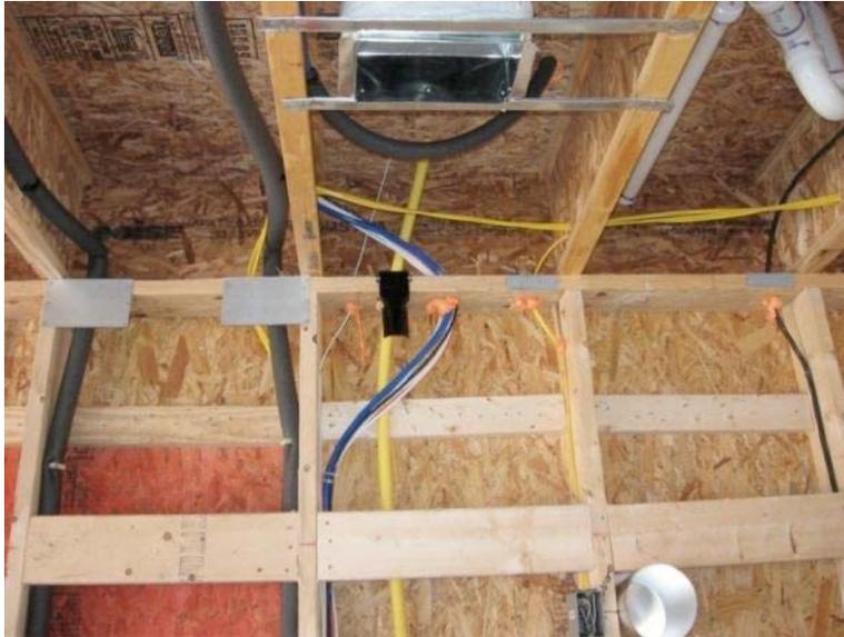
**Figure 4 - Exterior Walls Single Top Plate and Stacked Framing**
