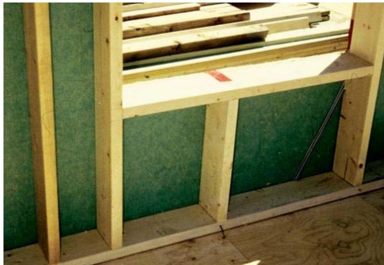
**Figure 5 - Exterior Walls Single King Studs without Jack Studs**
