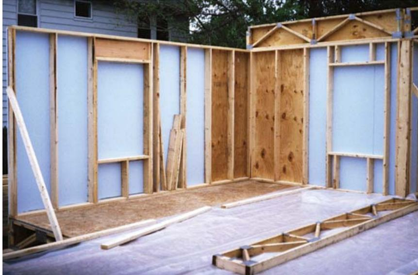
Figure 6 - Exterior Walls Non-Load Bearing Headers Removed
