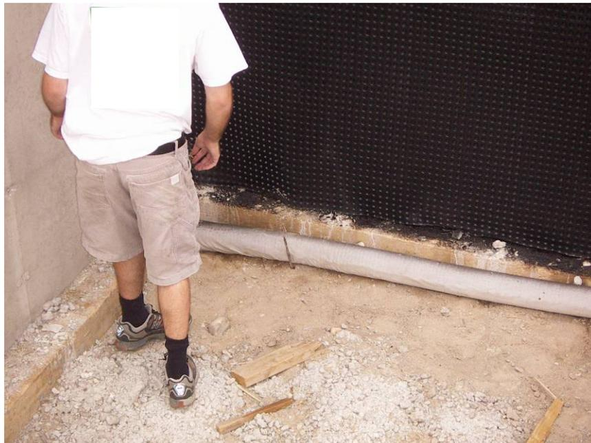
**Figure 16. Flexible footing drain installed, with pre-installed filter fabric mesh**
