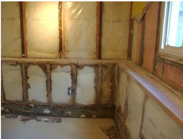
**Figure 4. Bulk water damage concealed behind interior finishes/insulation**
