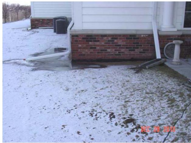
**Figure 5. Negative grade issues (accumulation refrozen roof runoff near foundation)**
