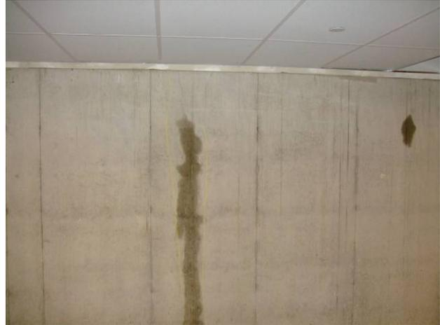
**Figure 3. Active seepage through cast concrete foundation wall (following rain event)**
