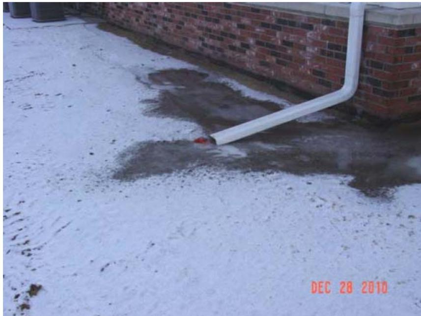
**Figure 10. Negative grade issues (accumulation refrozen roof runoff near foundation)**
