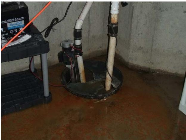
**Figure 19. Flooded basement due to saturated granular fill under slab**
