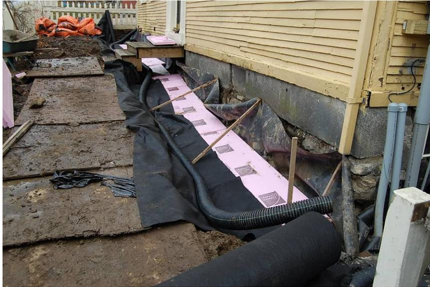
**Figure 30. Impermeable skirt with horizontal insulation and drainage (c/o Petersen Engineering)**
