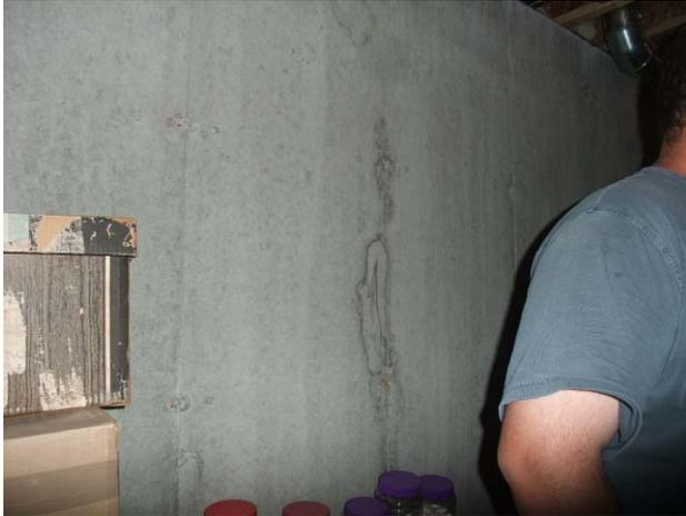
**Figure 2. Wall water seepage patterns (at form tie penetration in cast concrete wall)**
