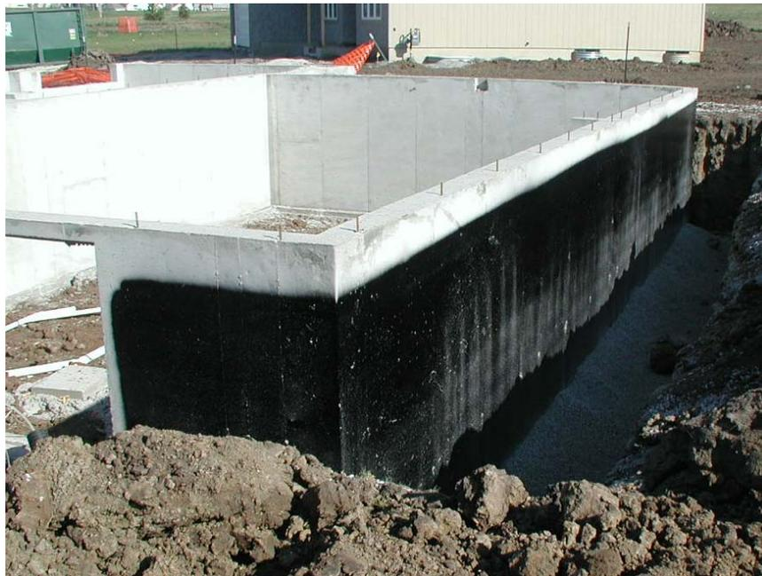
**Figure 11. Dampproofing applied to cast concrete foundation wall**
