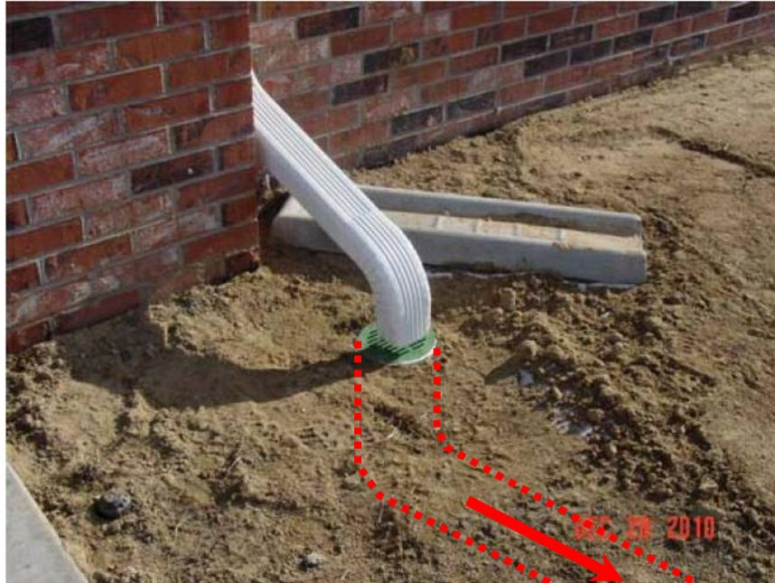
**Figure 7. Downspout directed to in-ground drain (not connected to footing drain system)**
