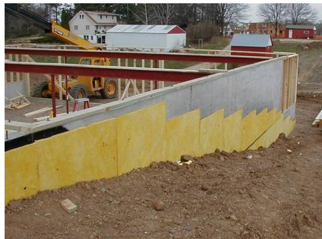
**Figure 13. Exterior foundation insulation using draining rigid fiberglass board**
