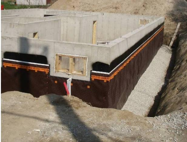
**Figure 14. Air gap membrane applied over damproofing on cast concrete wall**
