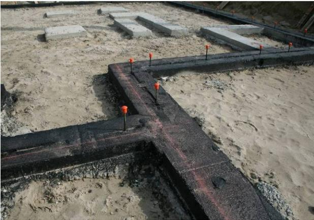
**Figure 22. Capillary break using liquid-applied dampproofing on top of footing**
