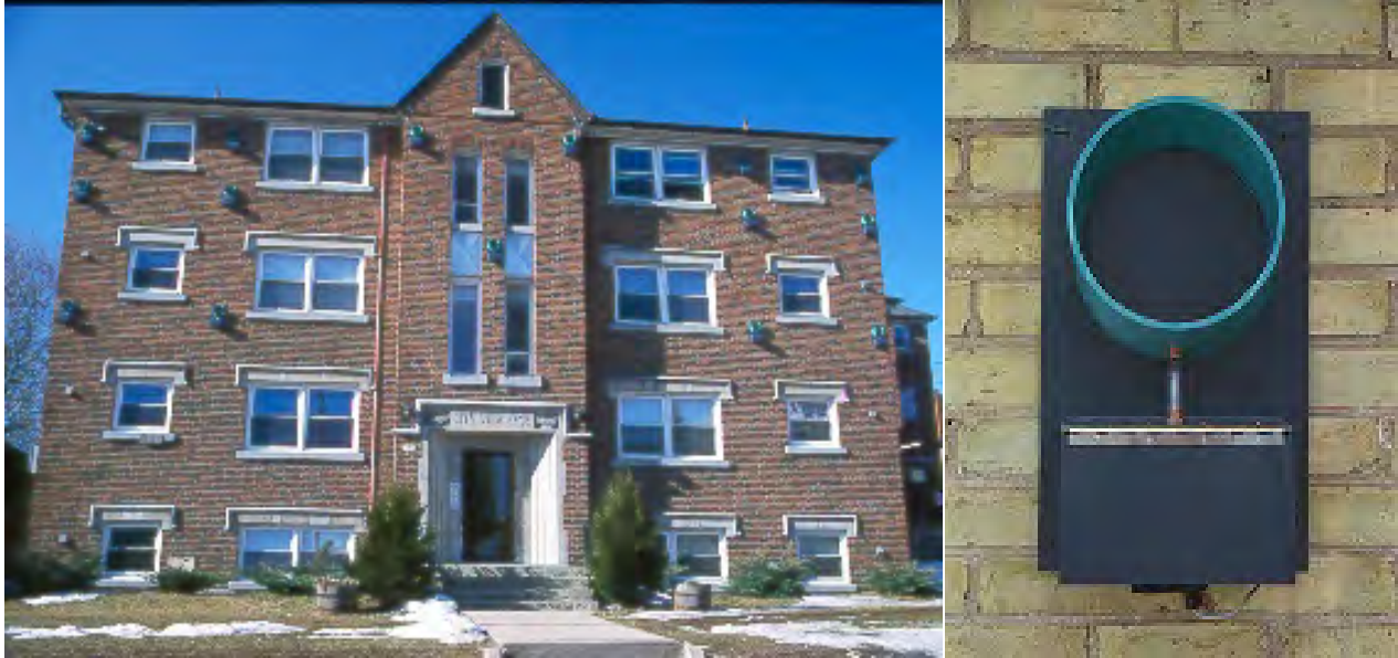
Figure 91: Instrumented occupied building (Waterloo, ON) with driving rain gauges
