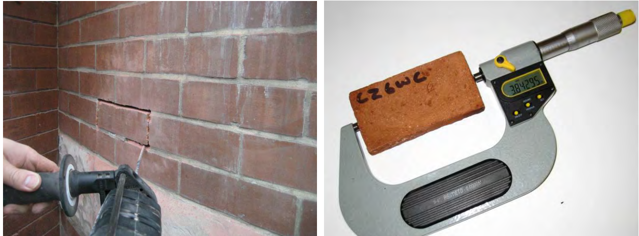
Figure 88: Removal of brick sample, and dilatometry (dimensional change) measurements
