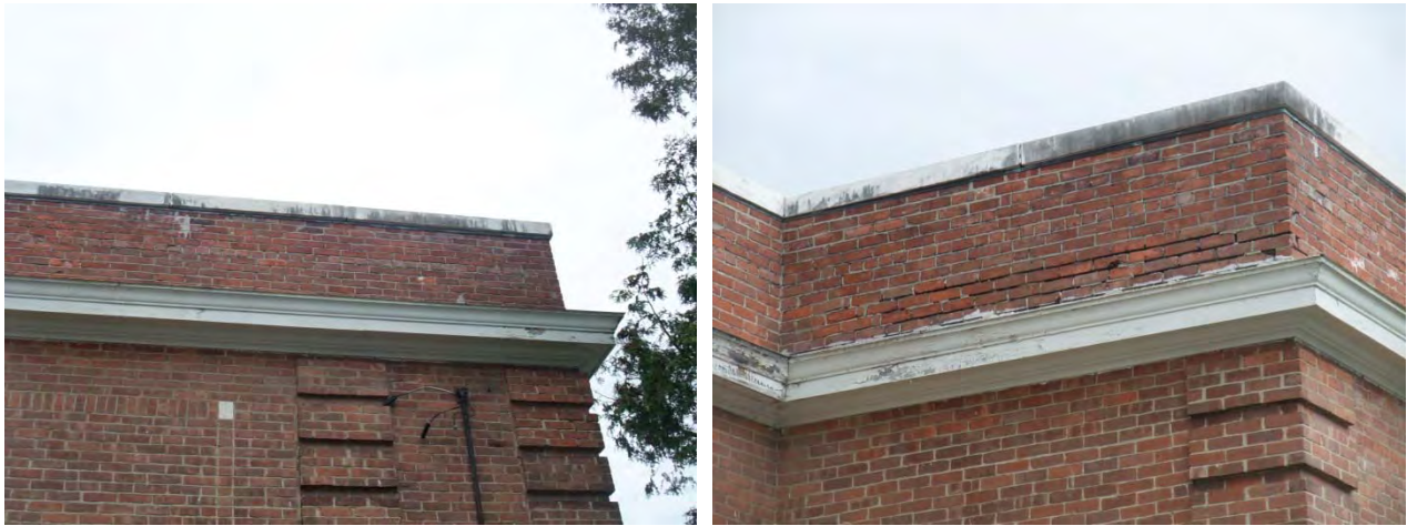
Figure 63: Stone parapet cap, with joints in stone coping
