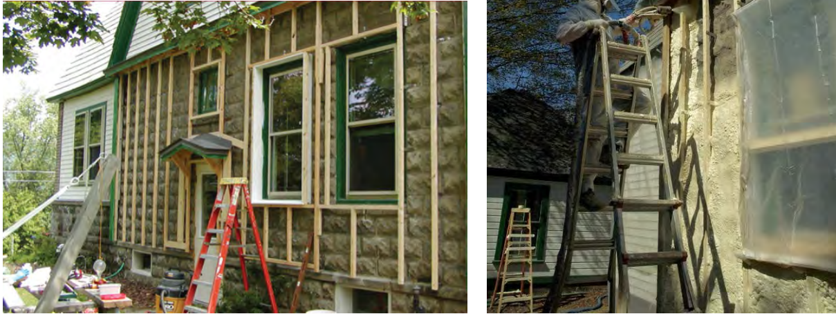
Figure 7: Exterior spray urethane foam retrofit on residential masonry
