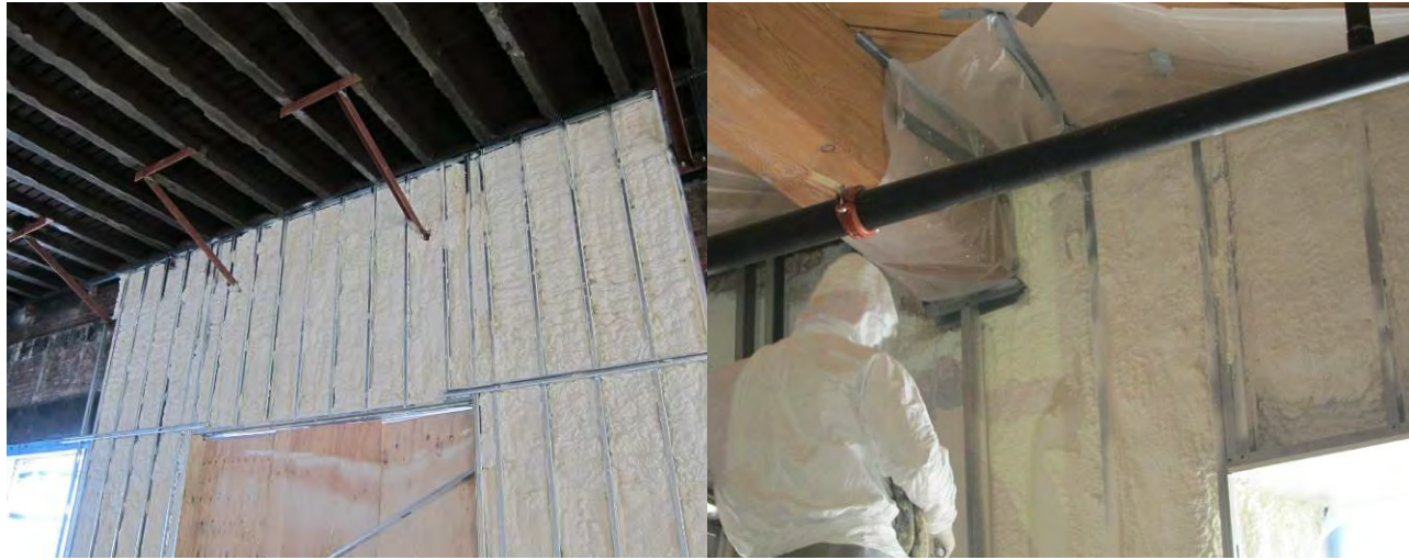
Figure 8: Various retrofit installations of interior spray foam insulation on mass masonry
